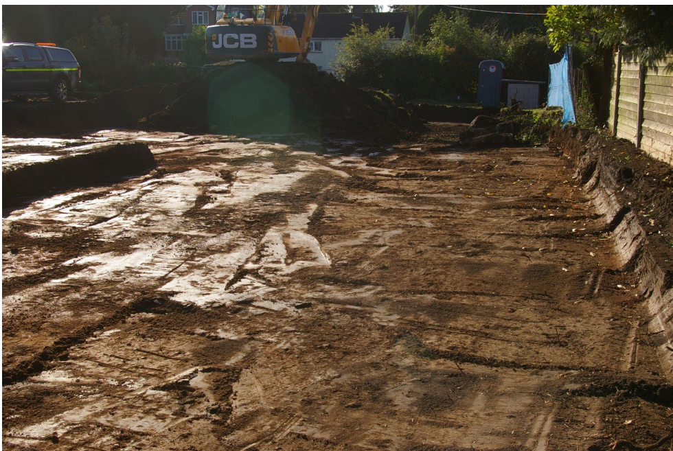
Figure 14: Western area, looking south
