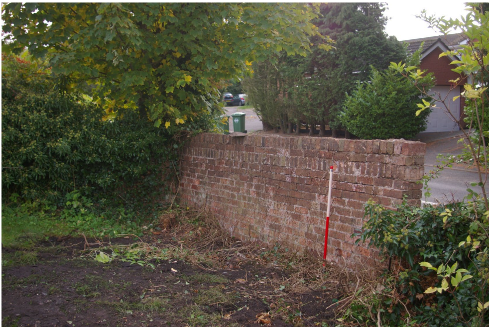
Figure 12: Boundary wall following clearance, looking south-east
