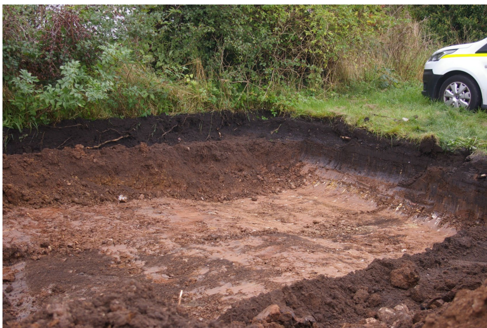
Figure 7: Reduction of ground level on eastern area of site, looking south-east
