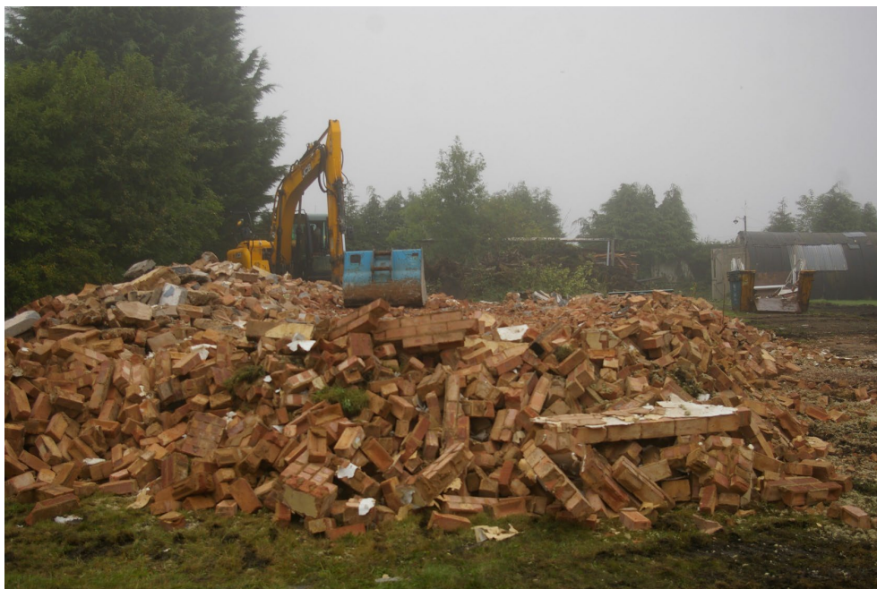
Figure 5: Rubble from demolition of bungalow, looking north
