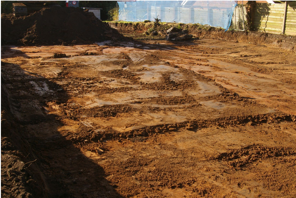
Figure 13: Western area once cleared of rubble and reduced, looking south-west
