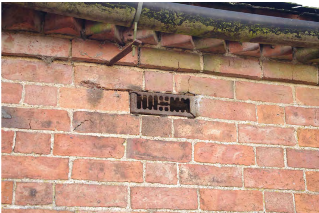
Figure 31 Building 1, south-east facing elevation vent and eaves detail Looking north-west
