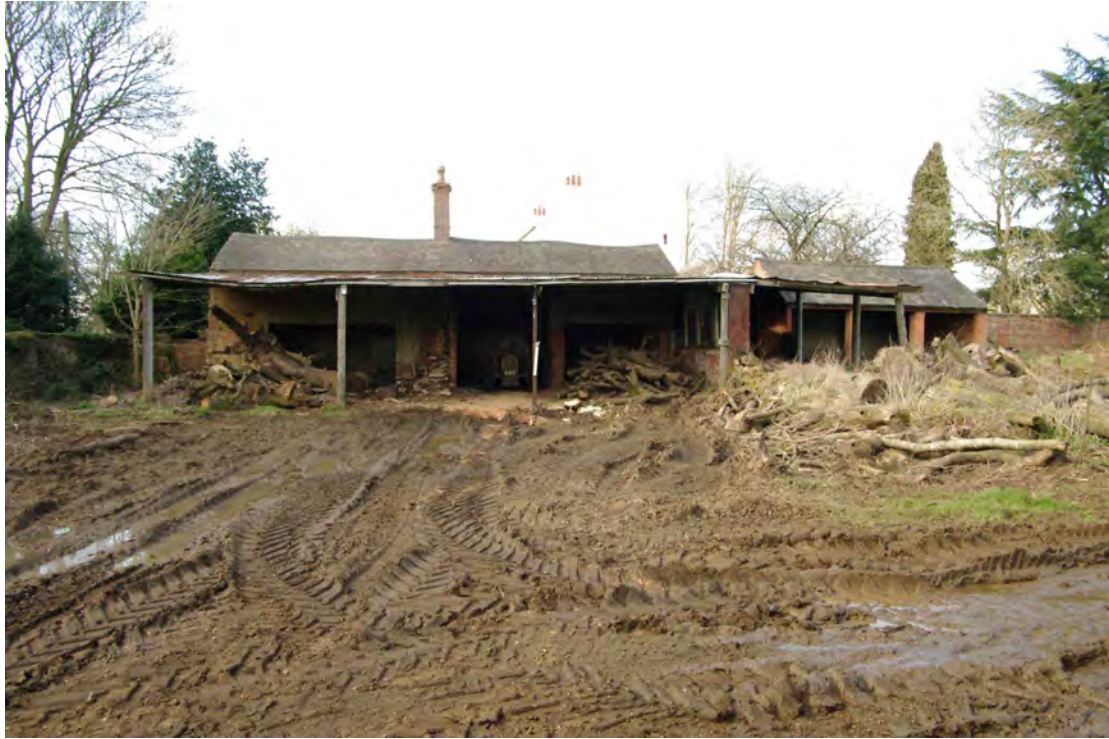
Figure 62 Building 4, east facing elevation Looking west. The former farmhouse element of Building 4 is everything to the left of the chimney stack
