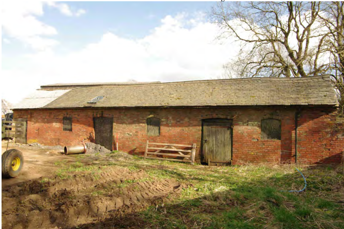
Figure 23 Building 1, north-west facing elevation Looking east
