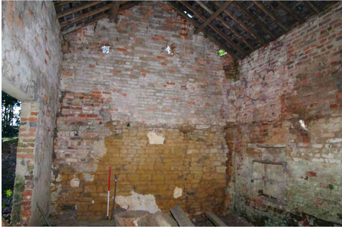
Figure 76 Building 4, southern gable end wall Looking south. 1m scale
