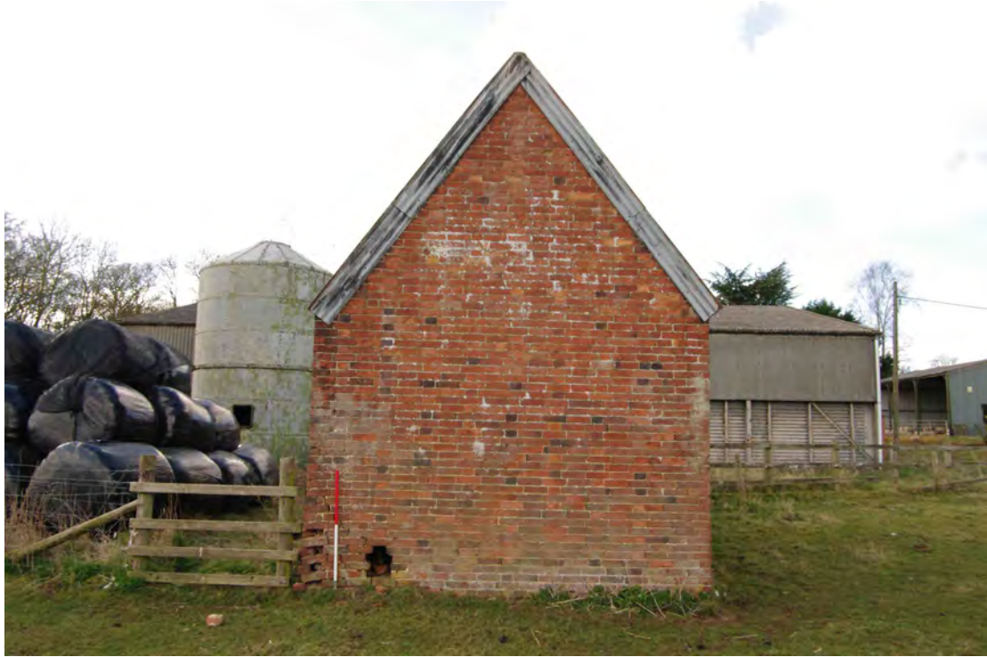
Figure 43 Building 2, east facing gable end Looking west. 1m scale
