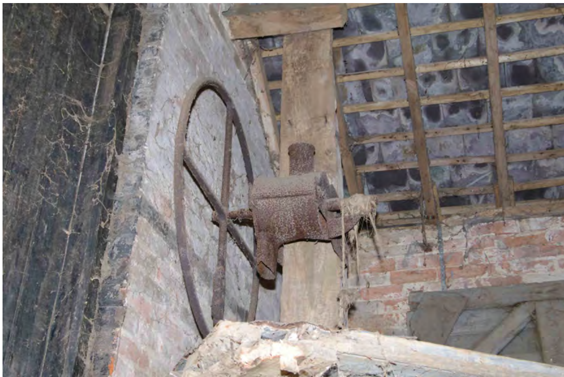
Figure 83 Building 4, northern room, milling equipment Looking west at equipment on 1st floor. The door on the left is the other side of the door shown in Figure 80
