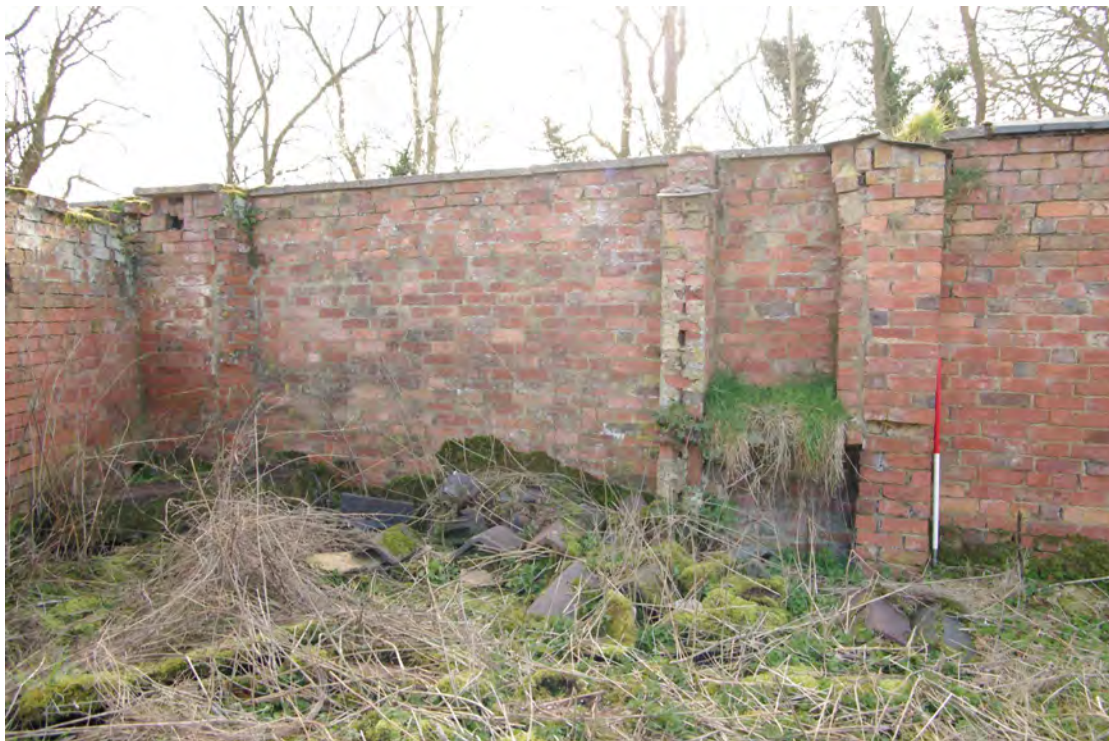
Figure 96 Eastern arm of boundary wall, former fireplace Looking south. 1m scale
