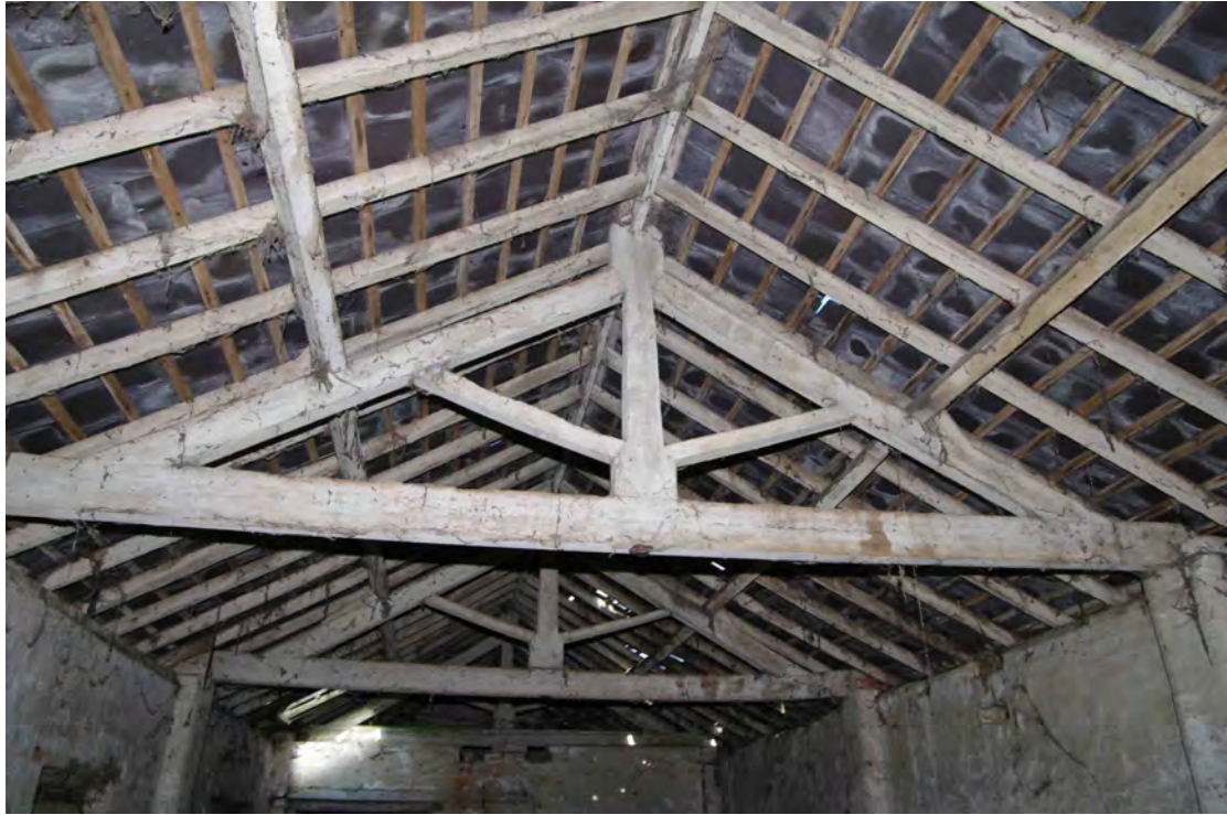
Figure 36 Building 1, roof detail Looking north-east
