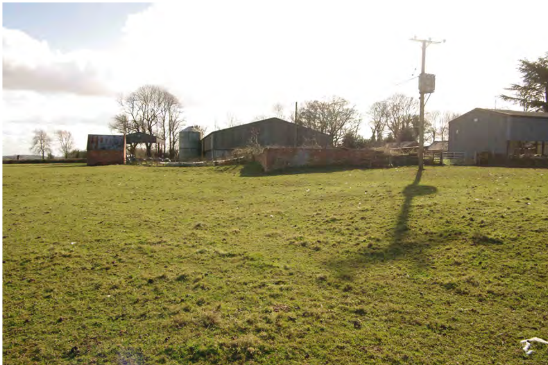
Figure 17 Cedars Farm viewed from the north Looking south. Building 2 on left, Buildings 3 and 4 can just be seen either side of the power line post. Note traces of earthworks in field
