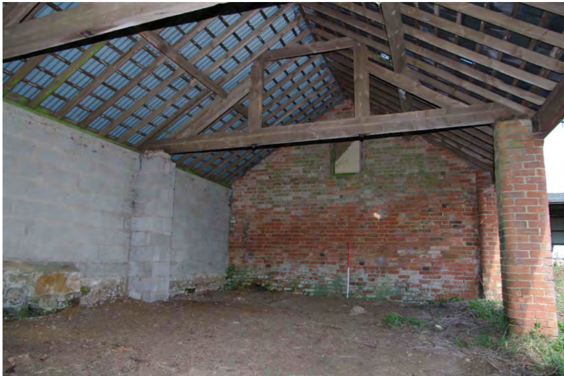
Figure 58 Building 3, internal view Looking north. 1m scale
