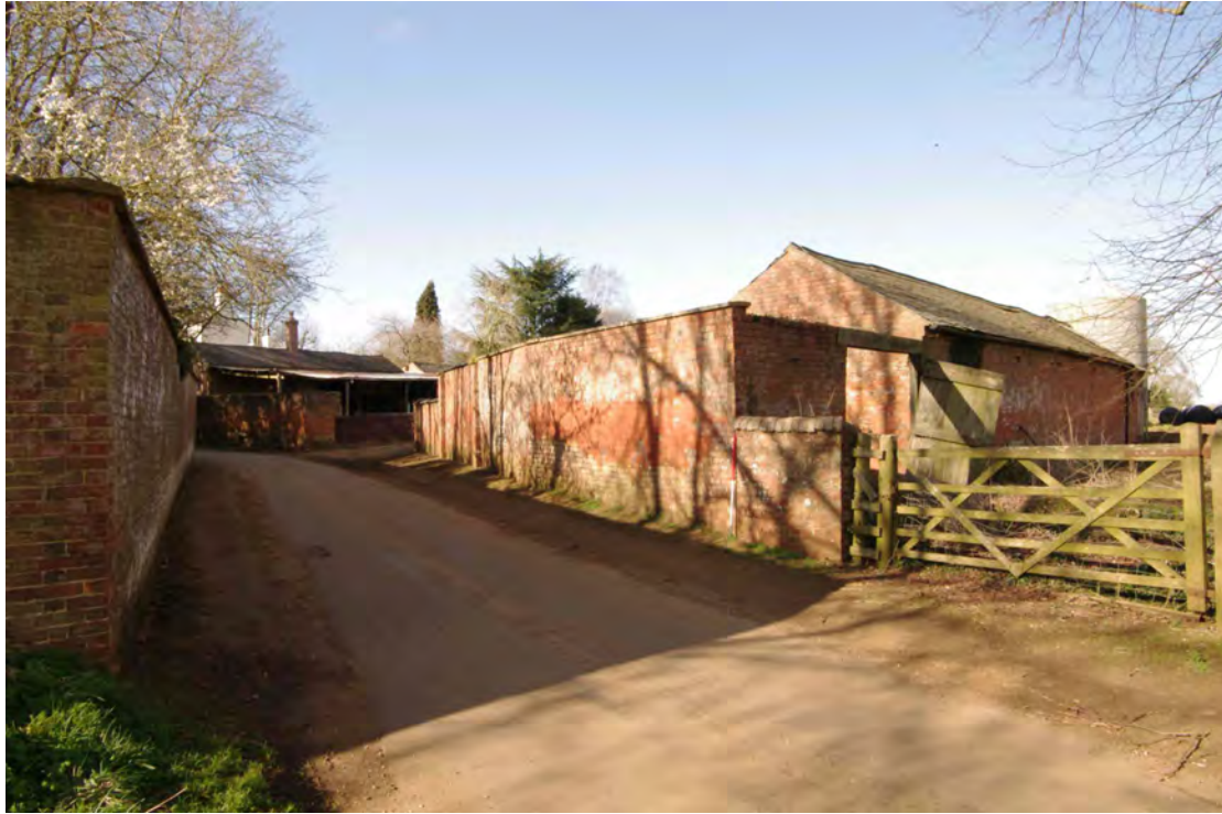
Figure 97 Eastern arm of boundary wall from Thornby Road Looking north-west. Initials picked out in blue bricks to left of 1m scale (see next figure). Building 1 is on the right
