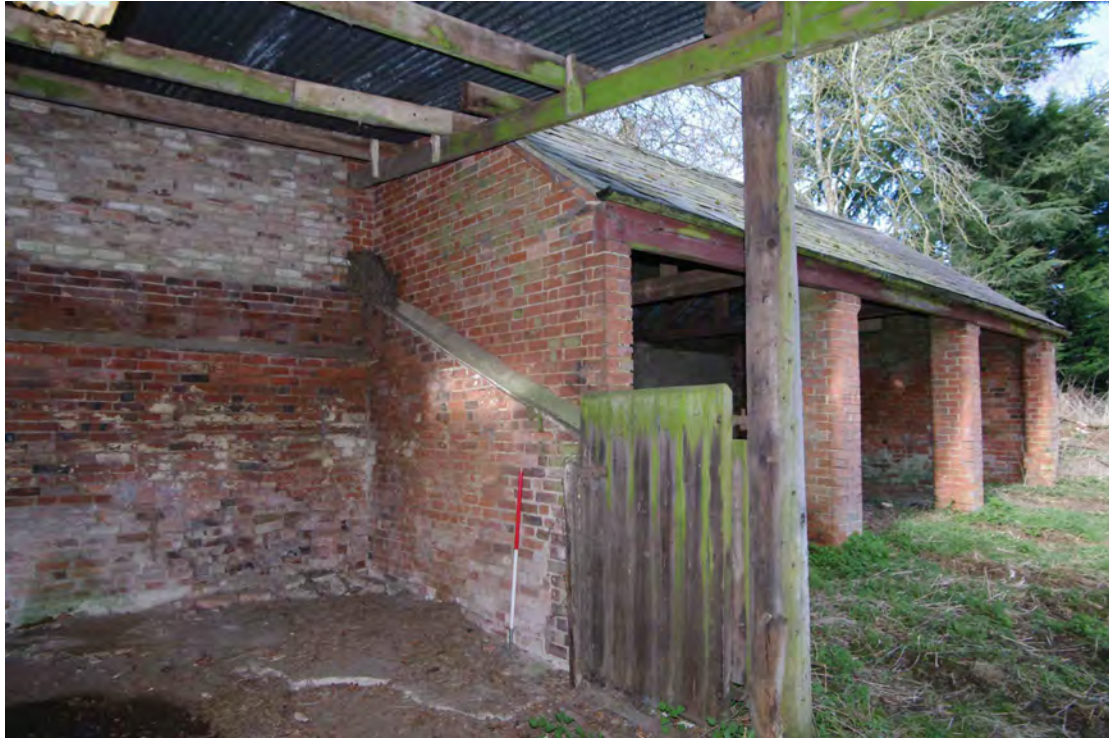
Figure 86 Building 4, north end bay Looking north-west. 1m scale. Building 3 to right
