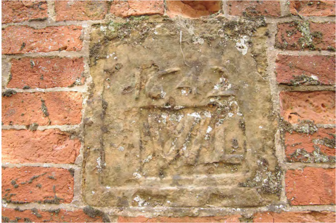
Figure 93 Boundary wall, datestone inserted into blocked doorway “1642 WL”
