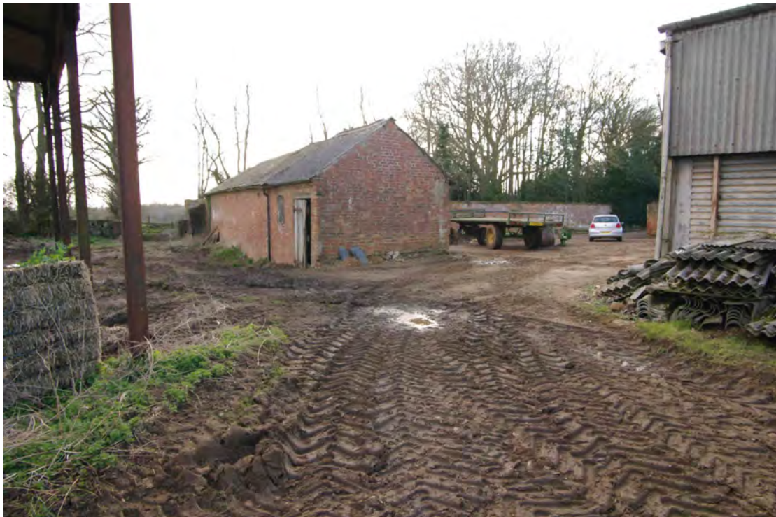
Figure 20 Building 1, northern gable end Looking south-west
