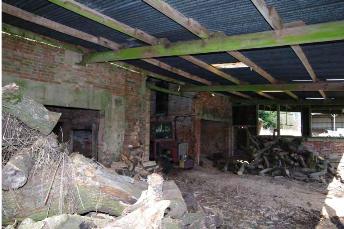
Figure 64 Building 4, east facing elevation Looking north-west
