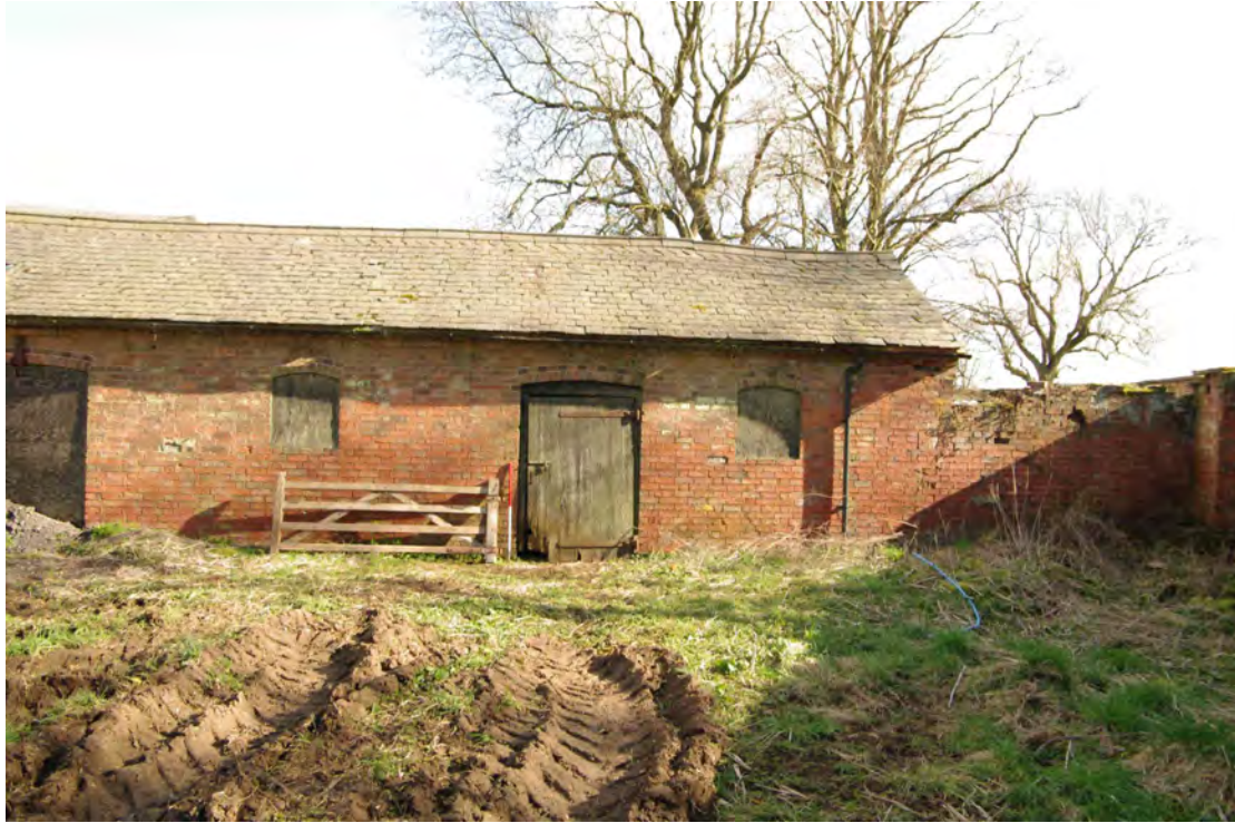
Figure 24 Barn 1, southern end of NW facing elevation Looking south-east. 1m scale. Note how the brickwork of the building is continuous with the open-roofed space at the right-hand end
