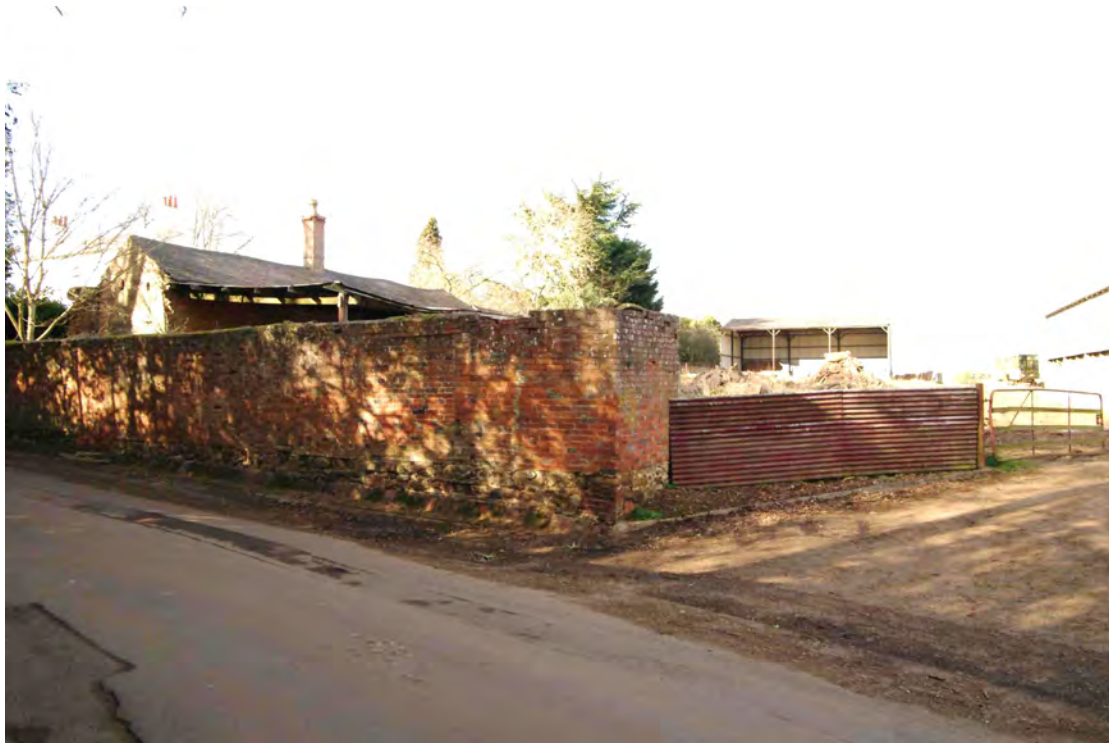
Figure 16 Site entrance and Building 4 from Thornby Road Looking north-west. Stone foundations to boundary wall (see later figures)
