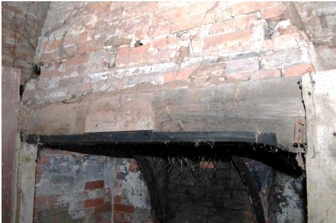
Figure 71 Building 4, bressumer beam across fireplace
