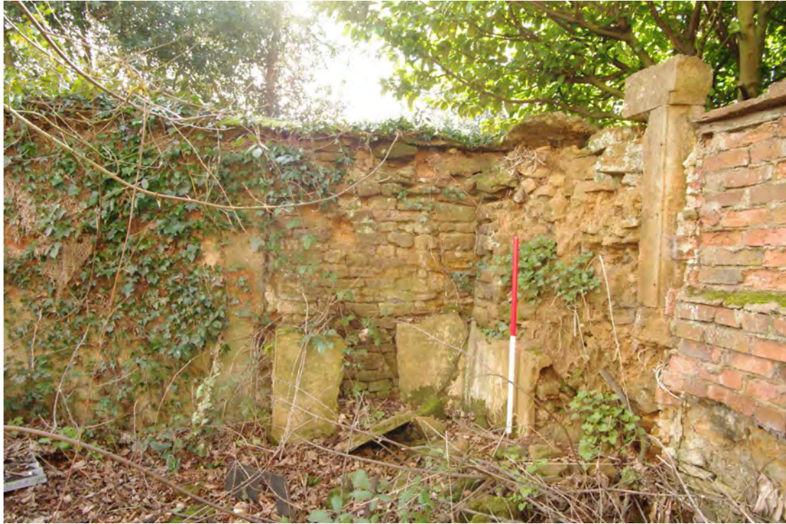
Figure 89 Blocked window on boundary wall alongside Thornby Road Looking south. 1m scale
