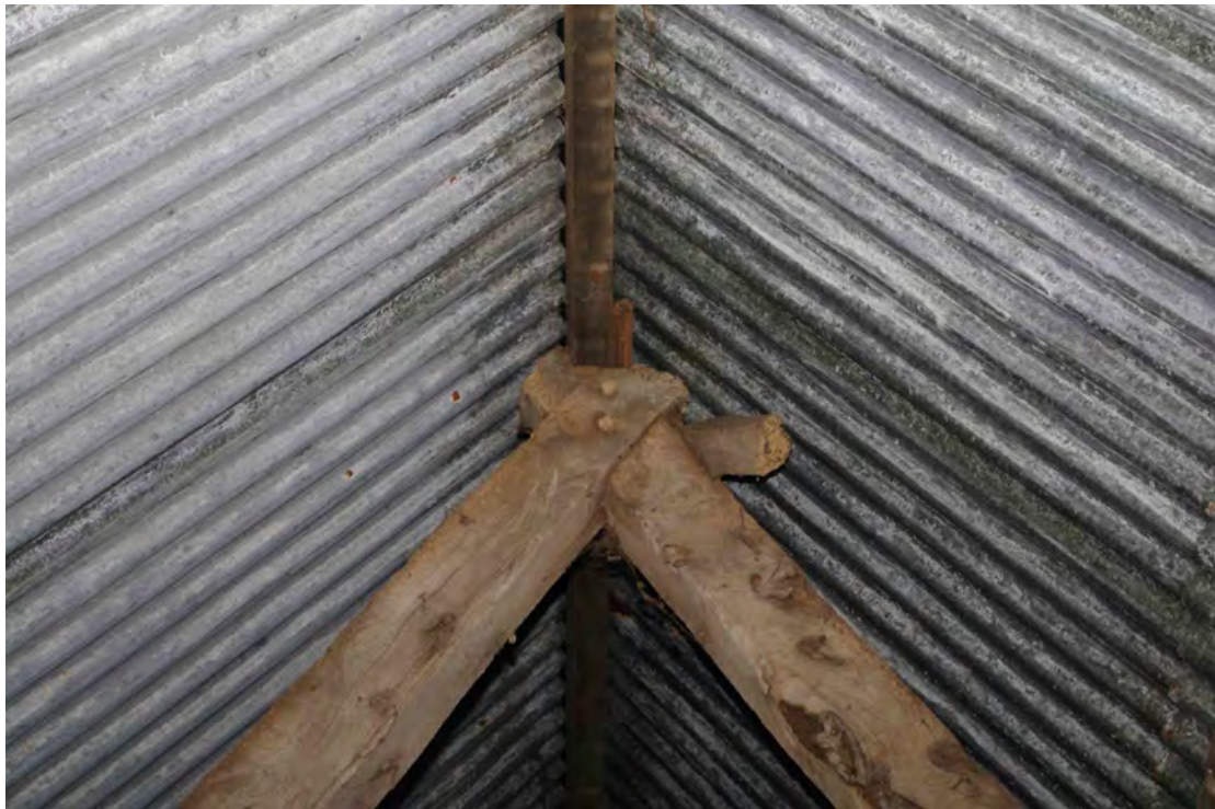
Figure 50 Building 2, pegged principal rafters at apex Looking east
