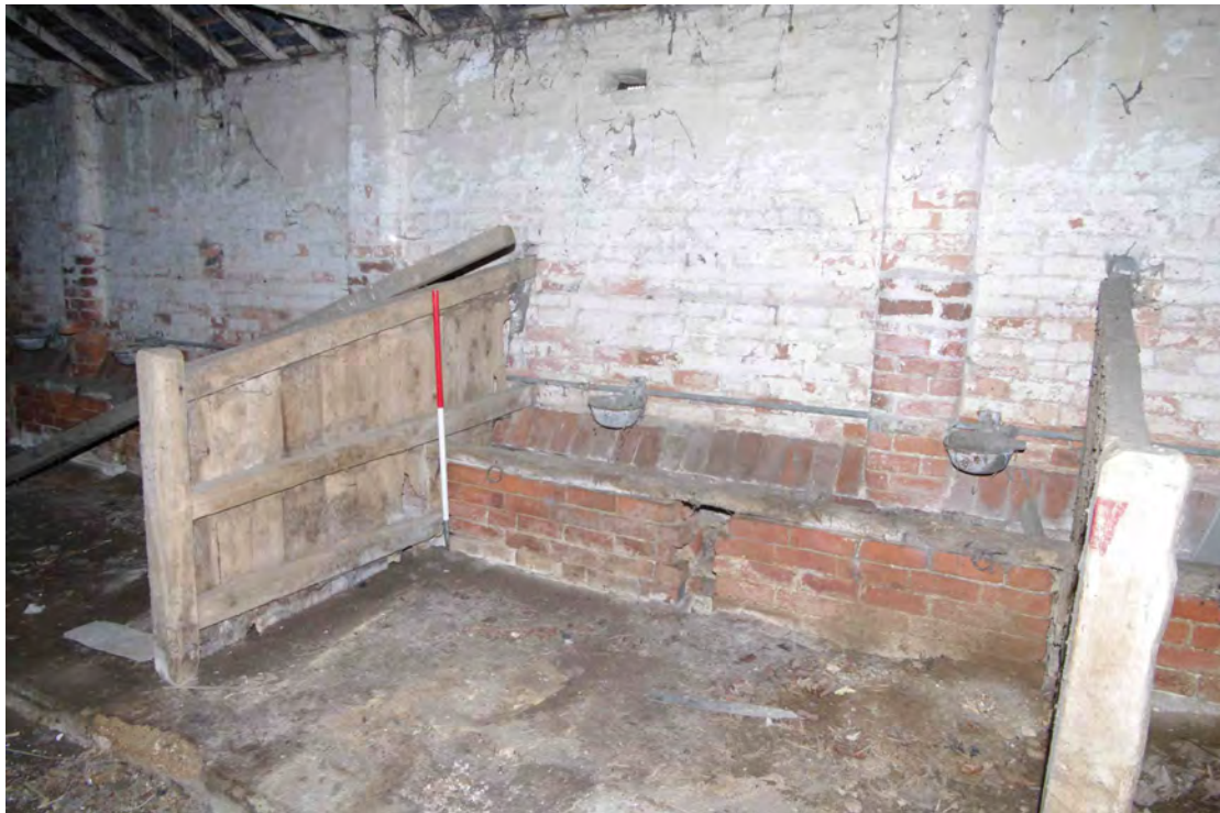
Figure 35 Building 1, stall detail Looking south-east. 1m scale
