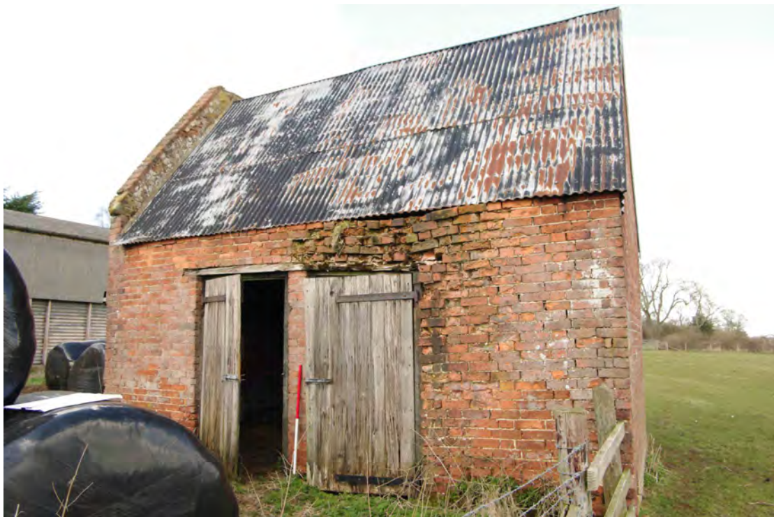
Figure 42 Building 2, south facing elevation Looking north-west. 1m scale
