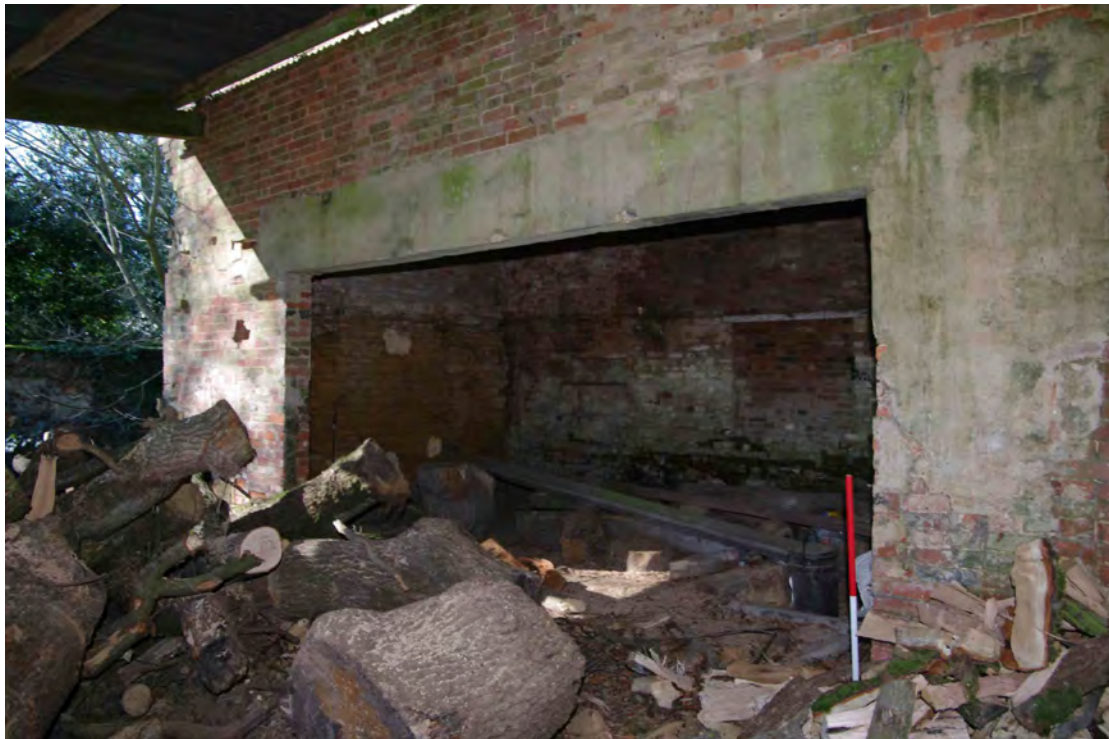
Figure 63 Building 4, southern end Looking south-west. 1m scale
