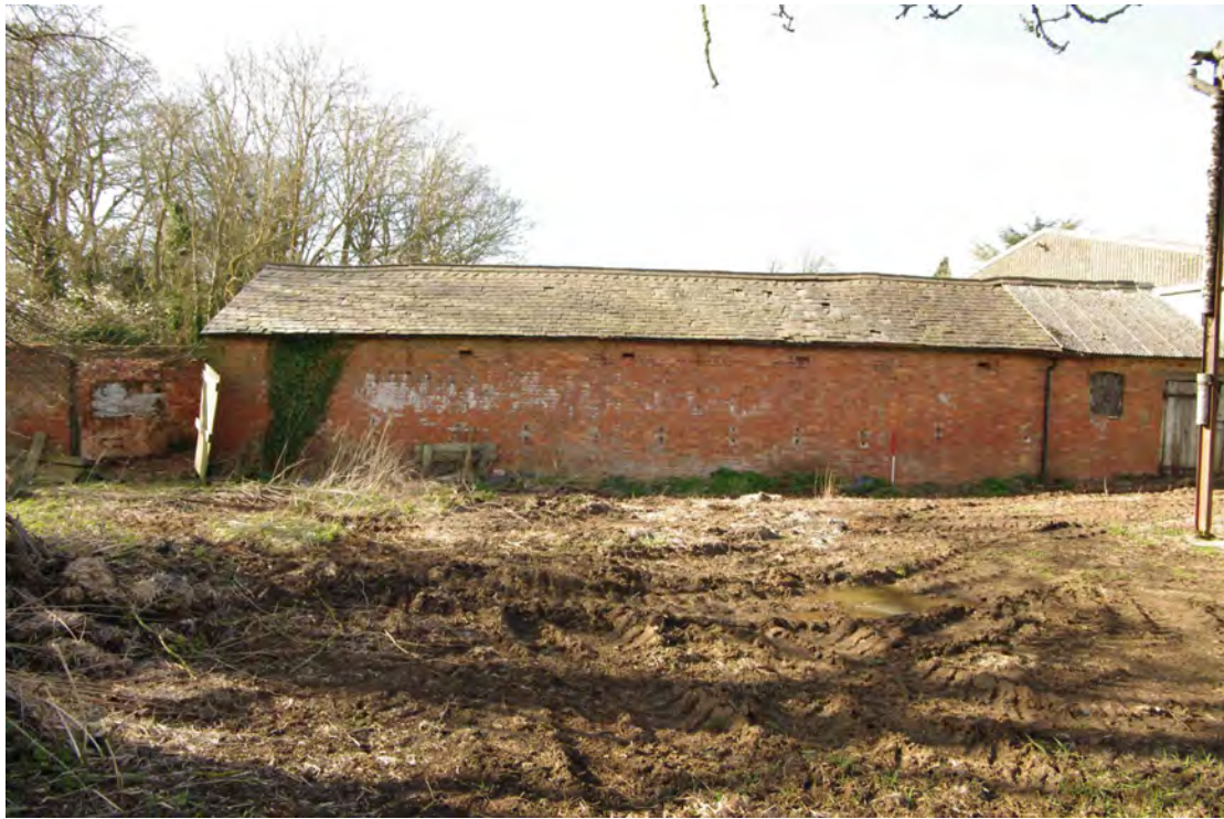
Figure 28 Building 1 south-east facing elevation Looking north-west. 1m scale
