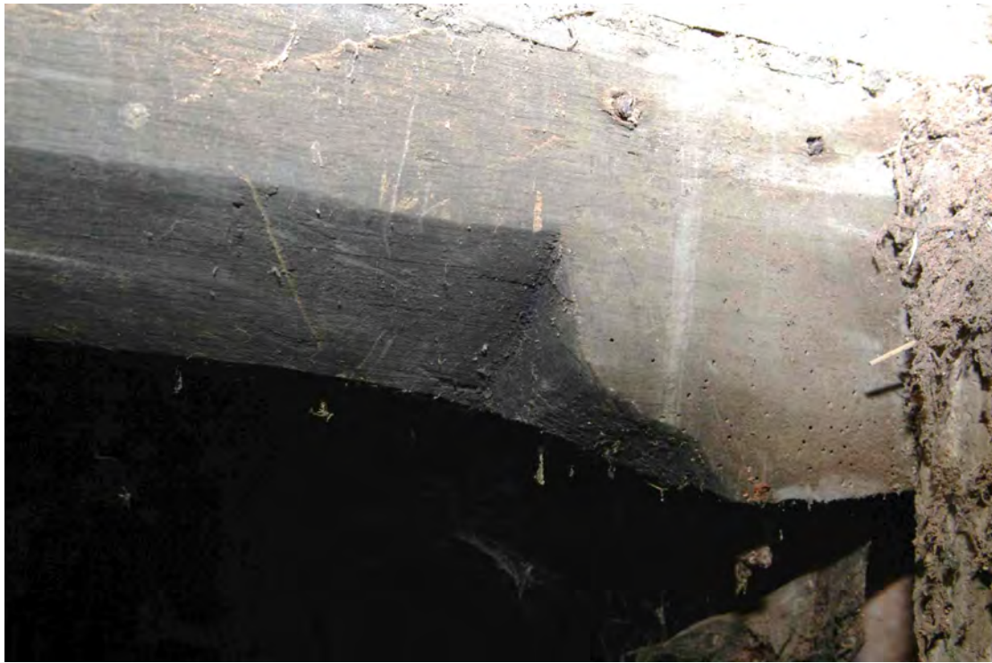
Figure 72 Building 4, chamfer detail on bressumer fireplace beam
