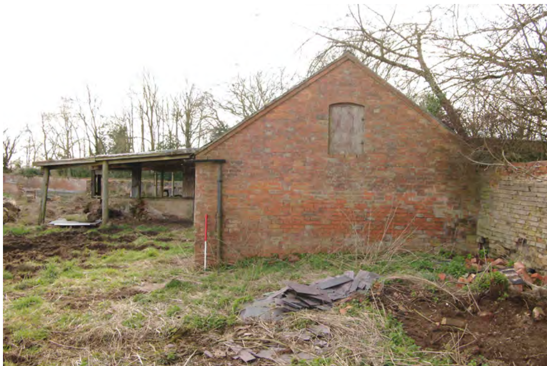
Figure 57 Building 3, north facing gable Looking south. 1m scale
