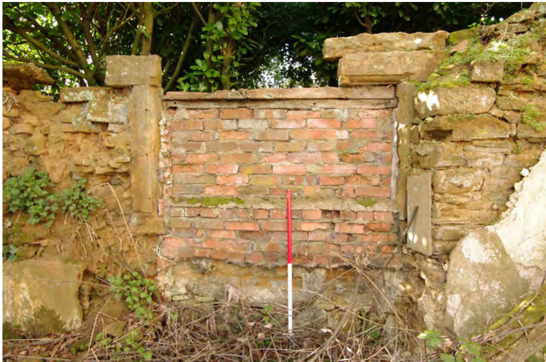
Figure 88 Blocked window on western part of boundary wall Looking west. 1m scale. Note the surviving wall plaster. Building 4 (out of shot) to right
