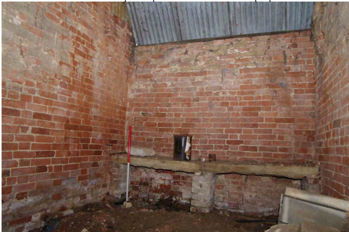
Figure 46 Building 2, western room
