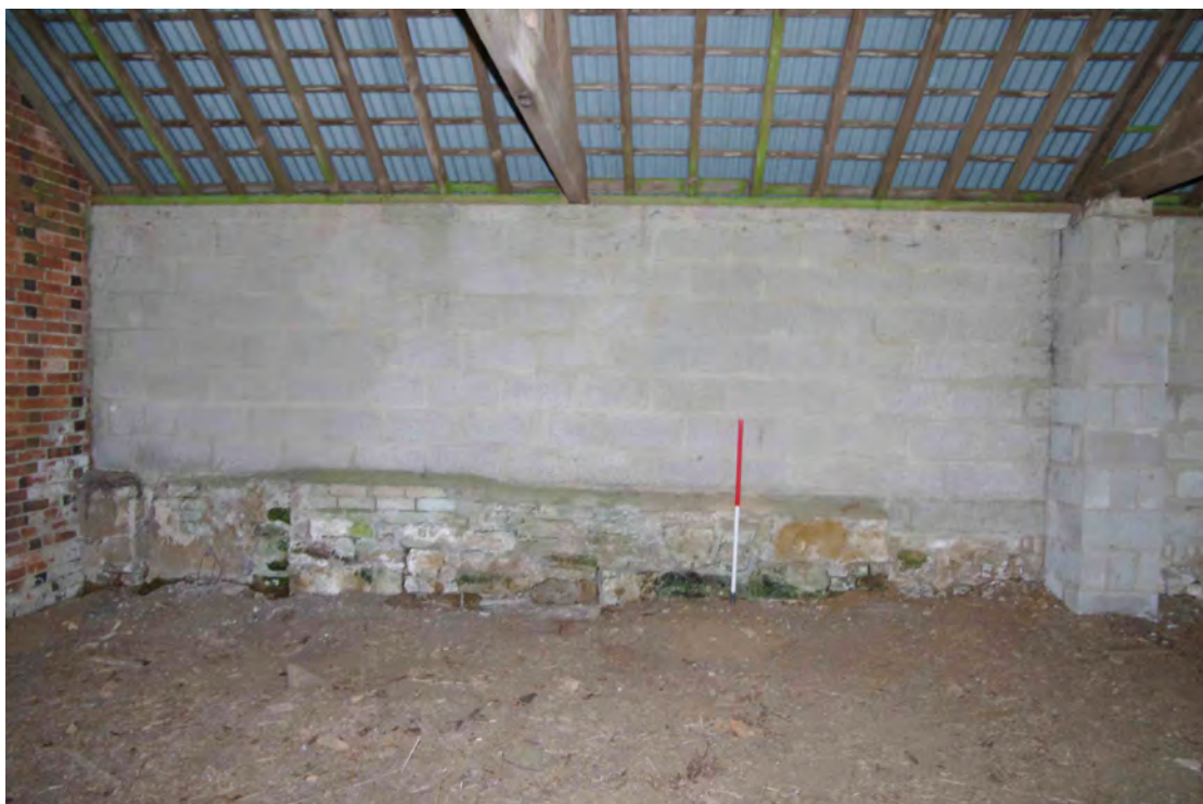
Figure 59 Building 3, stone wall base on west wall Looking west, 1m scale
