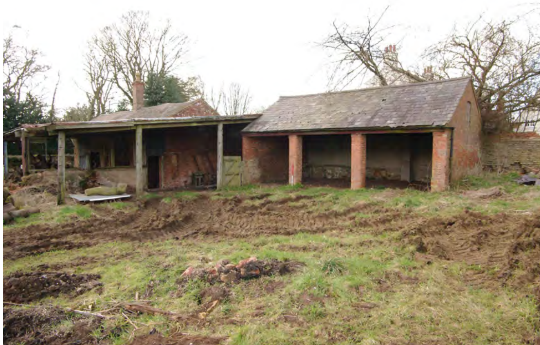
Figure 55 General view of Buildings 3 and 4 Looking south. Building 3 on the right
