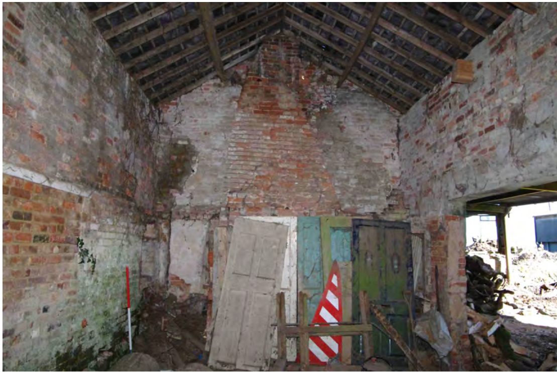
Figure 68 Building 4, general view of southern room Looking north. 1m scale
