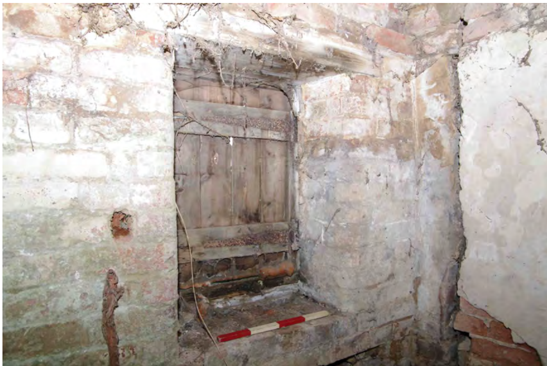
Figure 75 Building 4, shuttered window to side of fireplace Looking north-west. 0.4m scale
