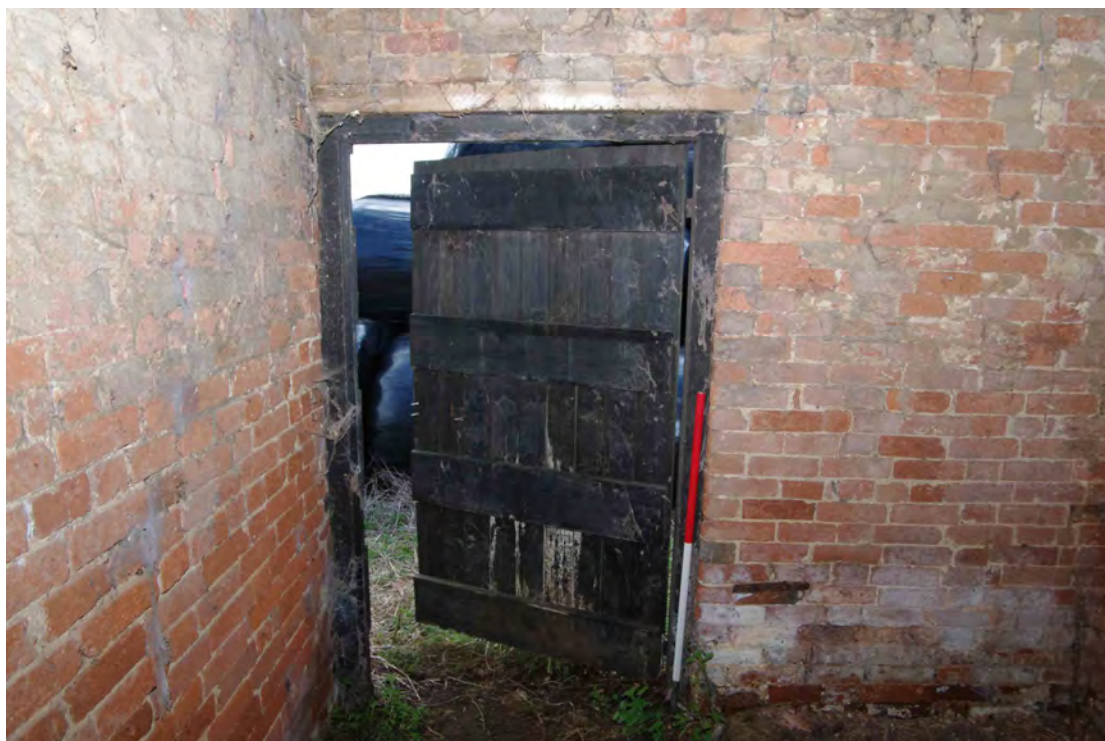
Figure 47 Building 2, western room Looking south. 1m scale
