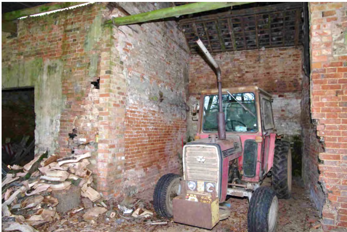
Figure 79 Building 4, centre room Looking south-west. Farmhouse room on left
