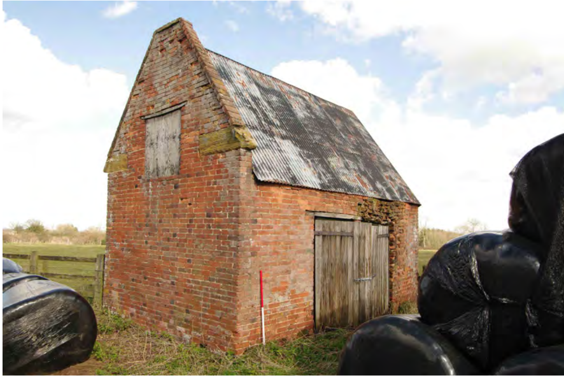
Figure 41 Building 2, west and south facing elevations Looking north-east. 1m scale
