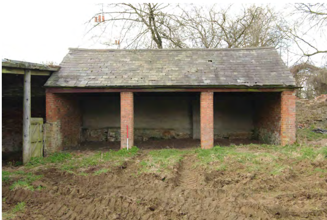
Figure 56 Building 3, east facing elevation Looking west. 1m scale
