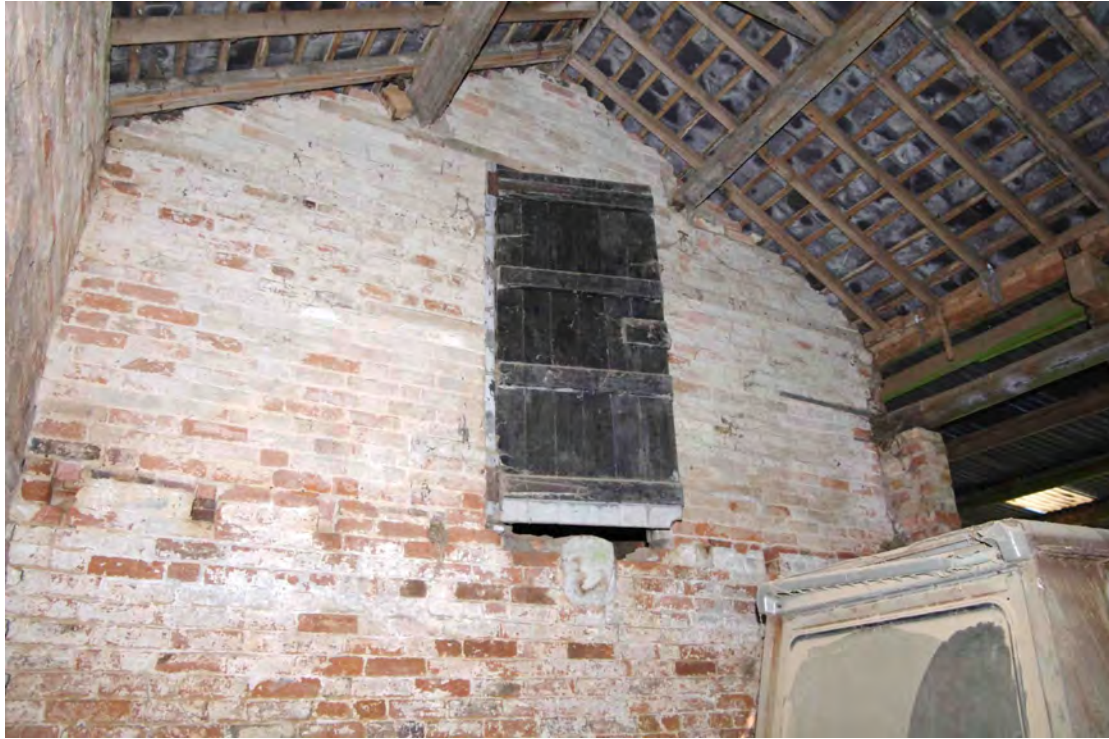
Figure 80 Building 4, centre room north wall Looking north. Note empty joist sockets
