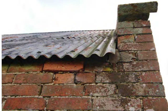
Figure 45 Building 2, close up of parapet
