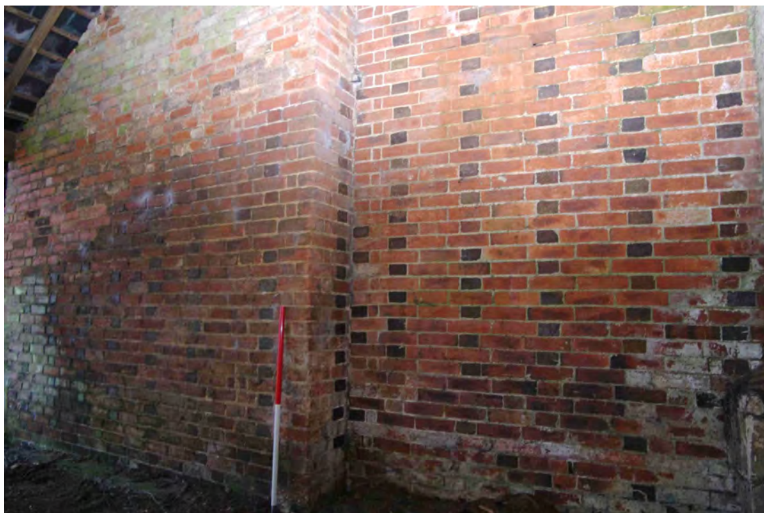
Figure 60 Building 3, internal view of south gable wall
