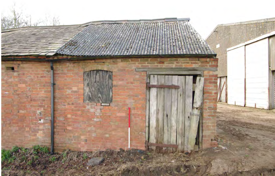
Figure 30 Building 1, south-east facing elevation, northern end Looking north-west. 1m scale
