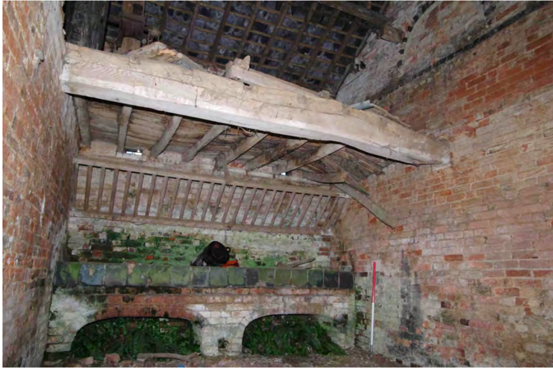
Figure 82 Building 4, northern room Looking north-west. 1m scale
