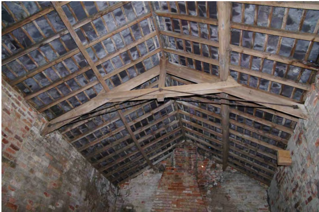
Figure 77 building 4, southern room roof structure Looking north
