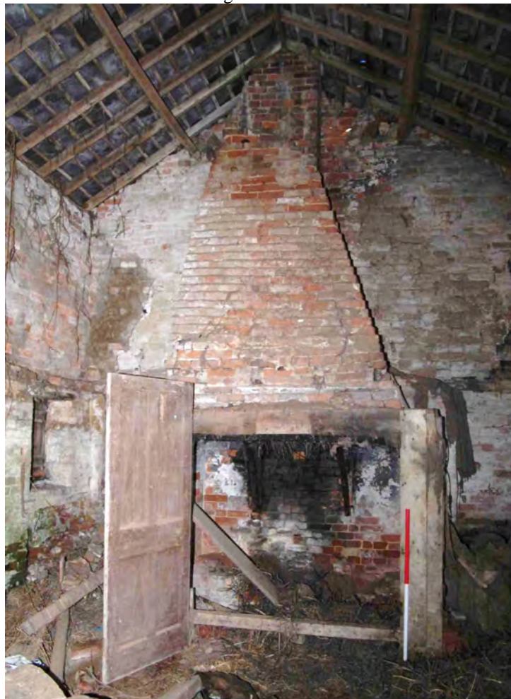
Figure 69 Building 4, fireplace Looking north. 1m scale
