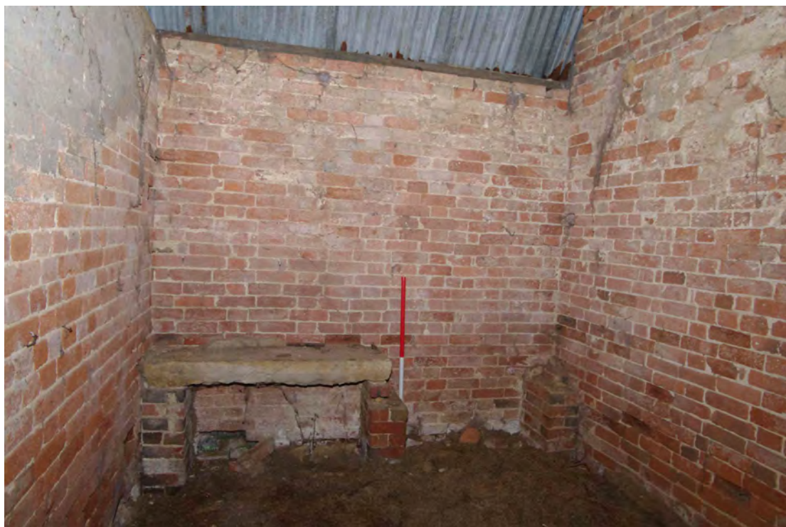
Figure 52 Building 2, eastern room Looking north. 1m scale
