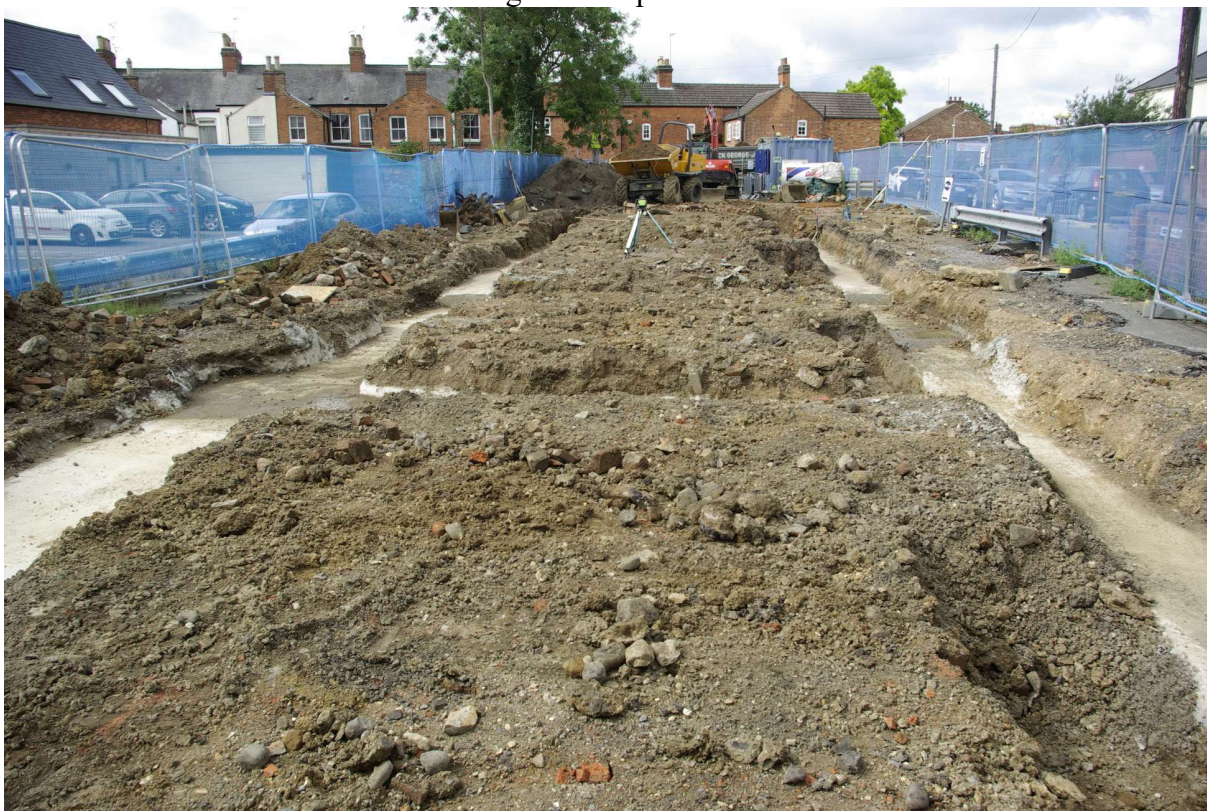
Figure 23 Concreted foundation trenches Looking south-west
