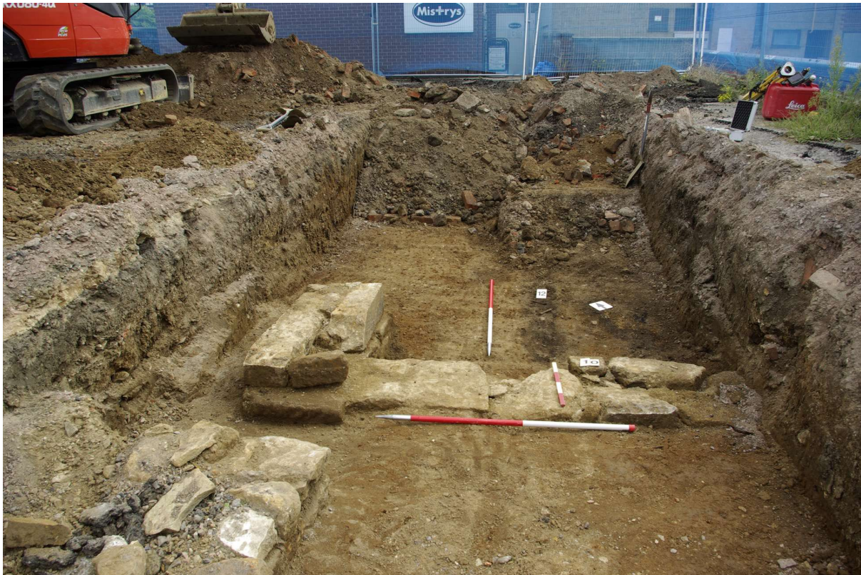
Figure 17 Wall (10) Looking north-east. Wall (5) lower left of picture. The gully [12] was modern
