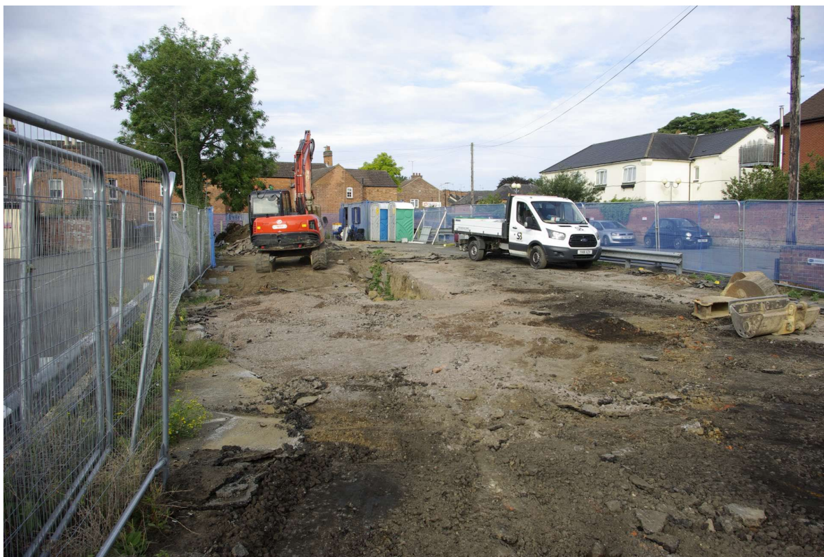
Figure 9 Site prior to excavation
