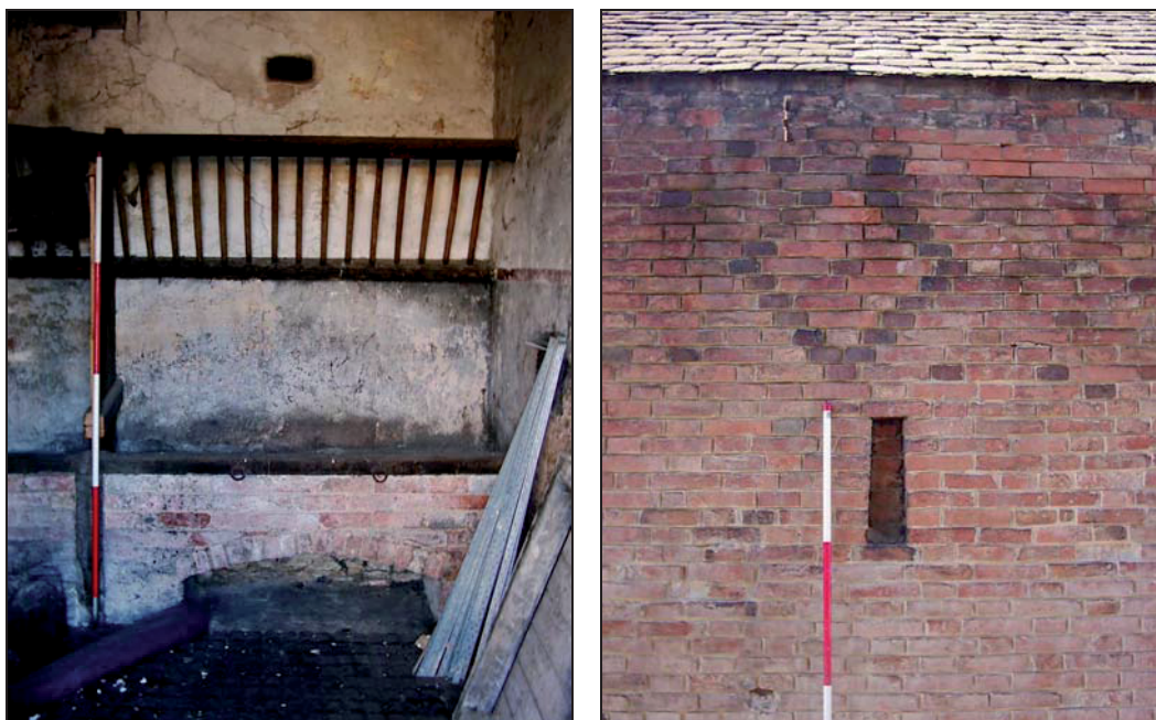
Figures 16 and 17: Bay 3, stable block and Diaper patterning on outhouse.
