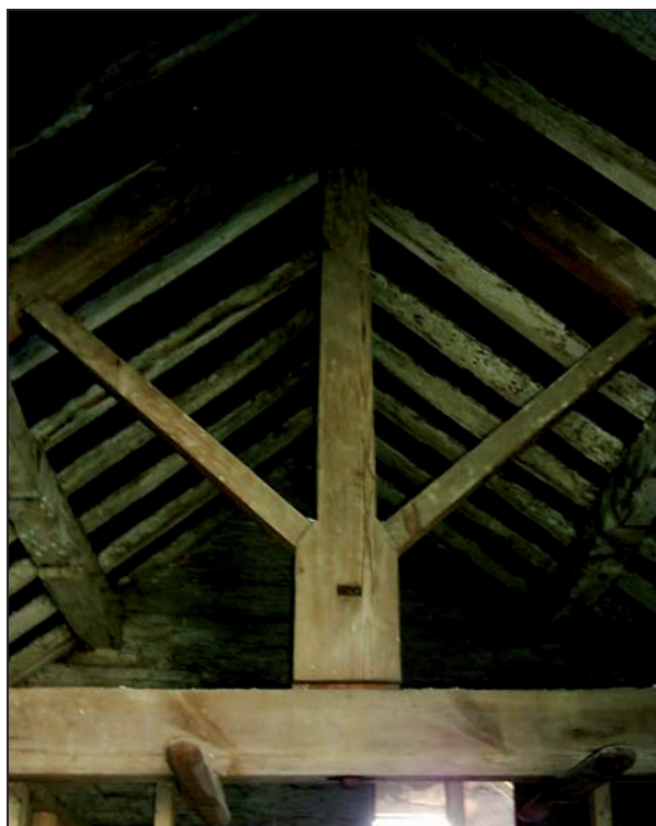
Figure 10: King-post roof truss.
