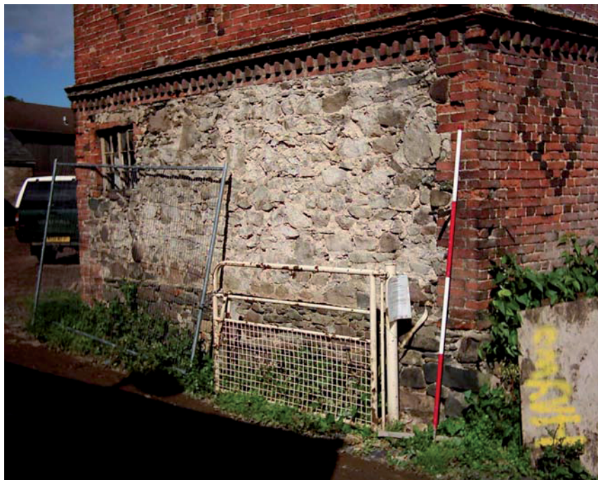
Figure 9: West gabled elevation showing stone built lower section of wall.
