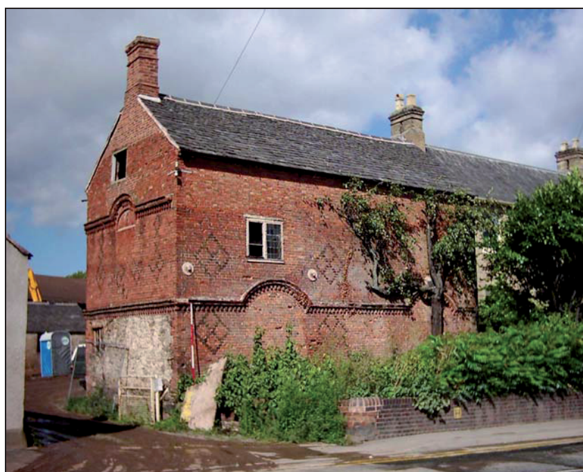
Figure 1: Front (south-east) elevation.
