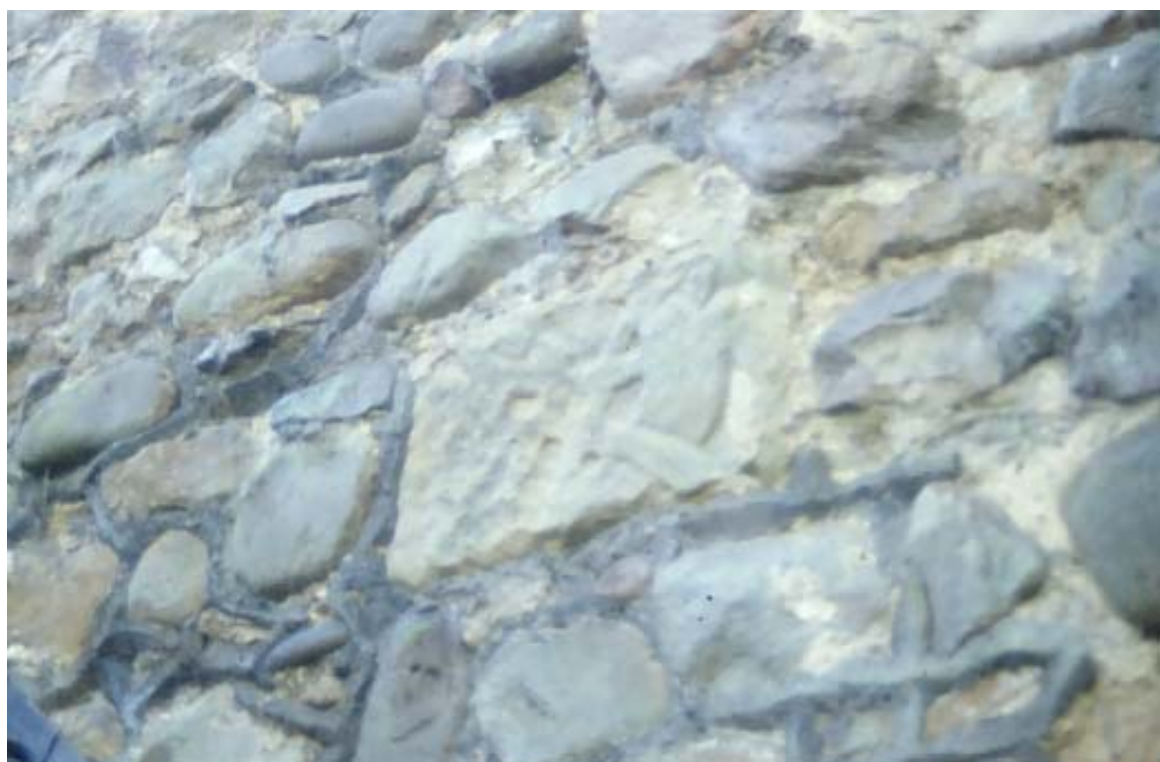
Figure 4 Detail of Re-used Saxon Stone in North wall.
