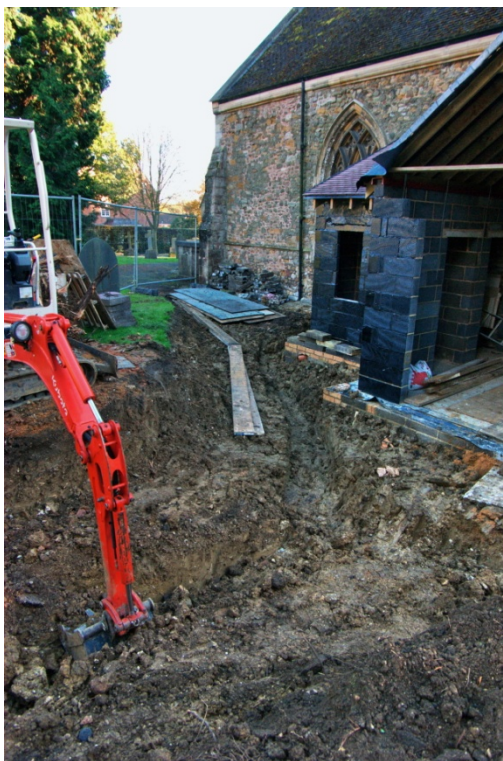
Figure 7 External Groundworks (looking east-south east).
