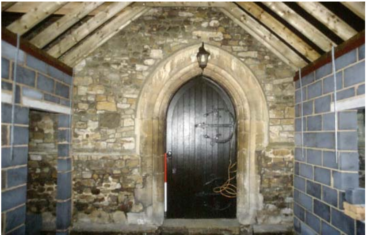
Figure 2 Northern wall and door.
