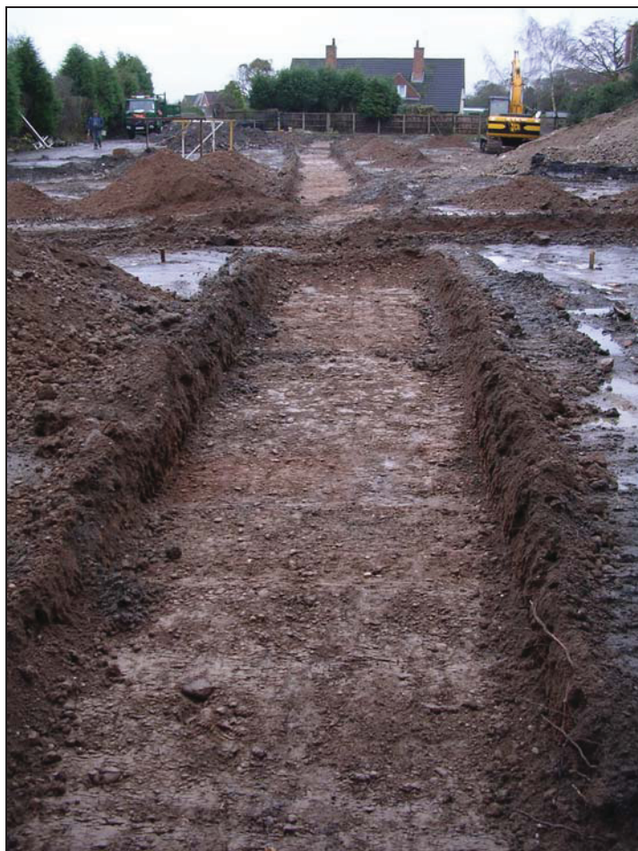
Figure 3: Trench 1 looking south
