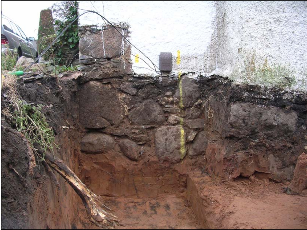
Figure 5: The exposed footings of The Gate House's north-west corner. Road level is represented by the top of the section on the left of the image, the footings for the extruding chimney stack can be observed on the right.
