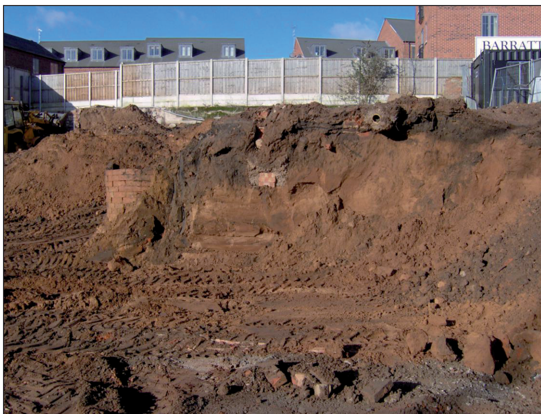
Figure 5. Section of area being stripped.
