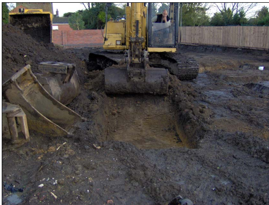
Figure 5 Plot 2 trial trench
