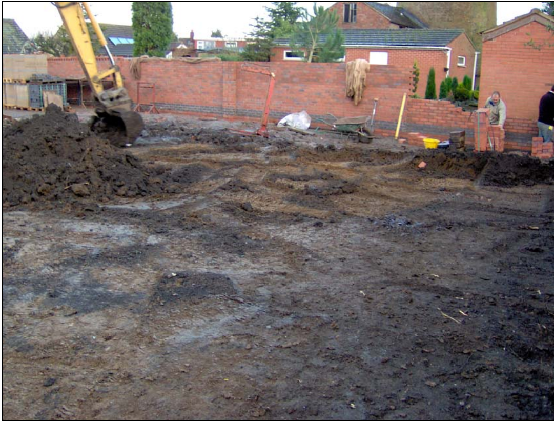
Figure 7 Plot 4 being stripped
