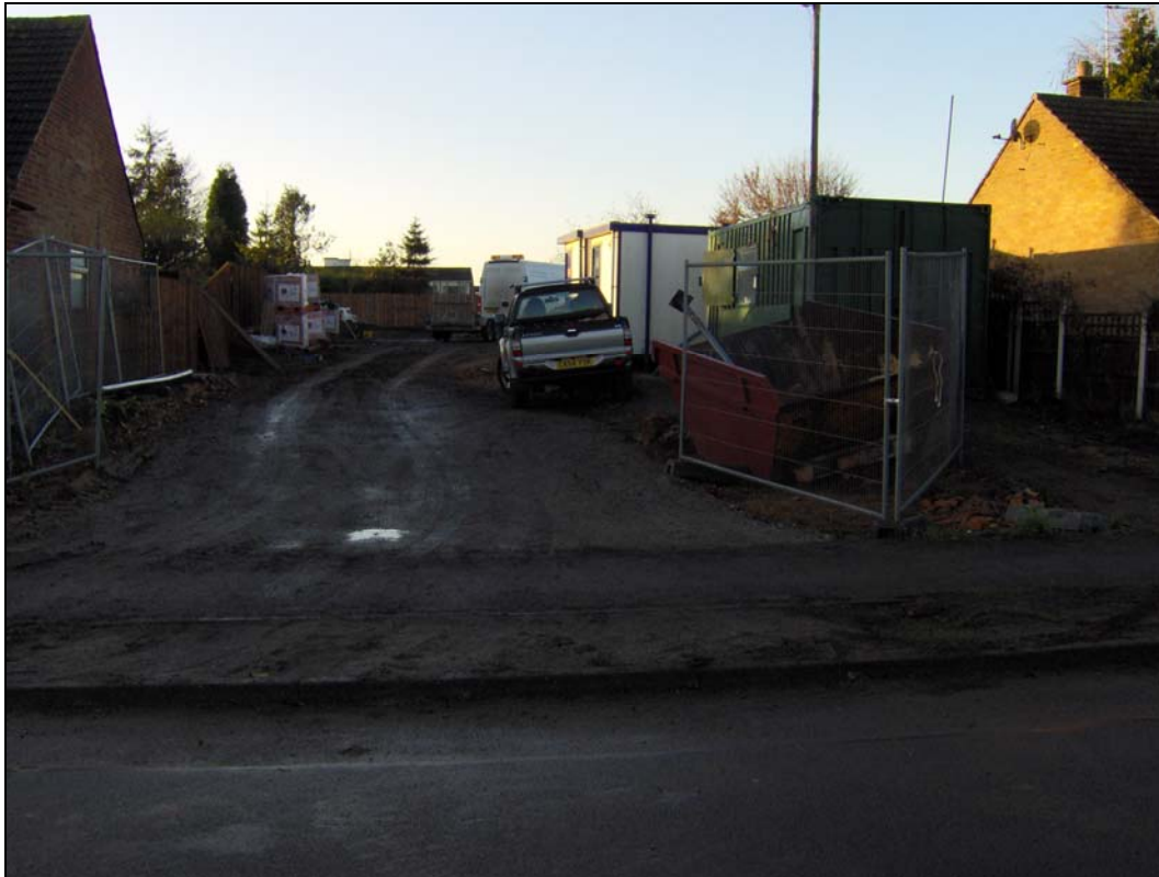
Figure 3 Site entrance Former bungalow beneath cabins.
