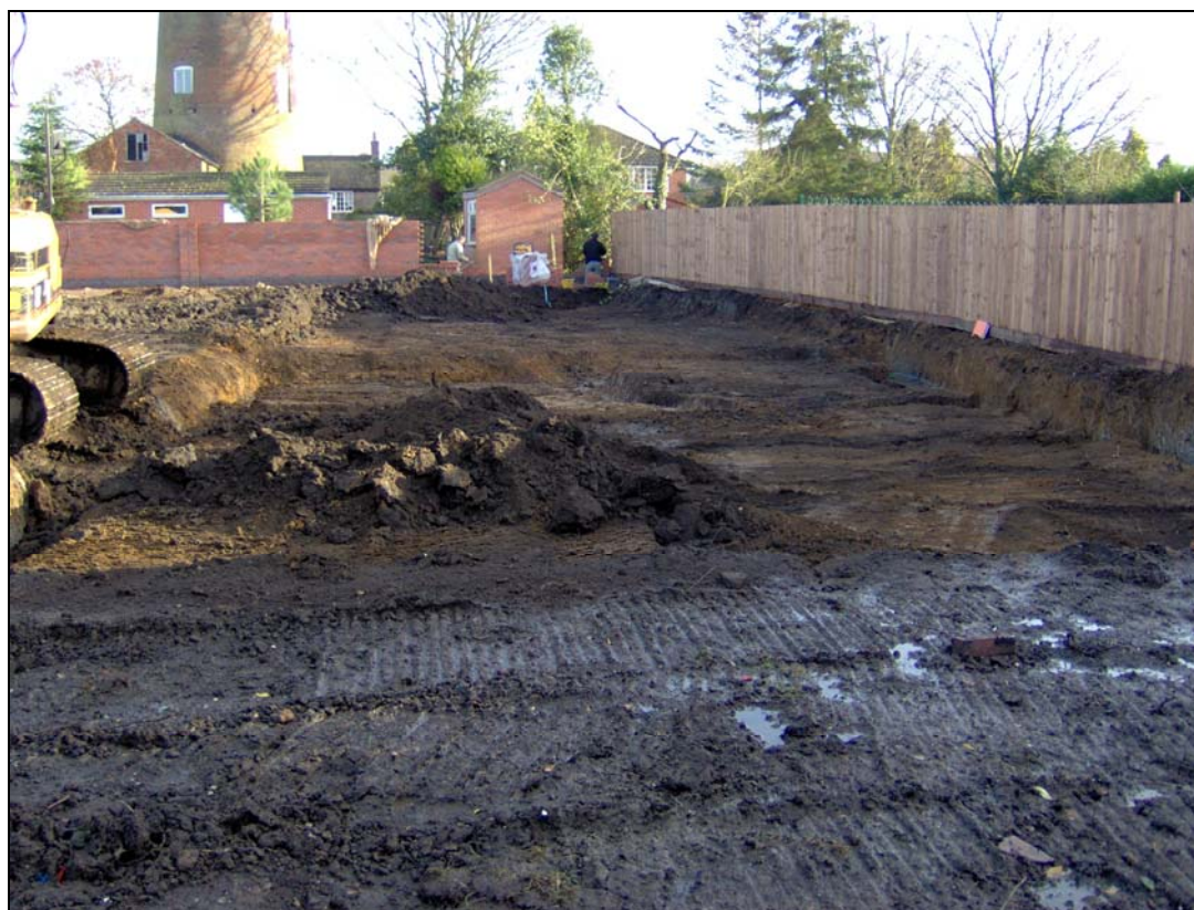
Figure 6 Stripped footprint of Plot 3 Note root disturbance along fenceline
