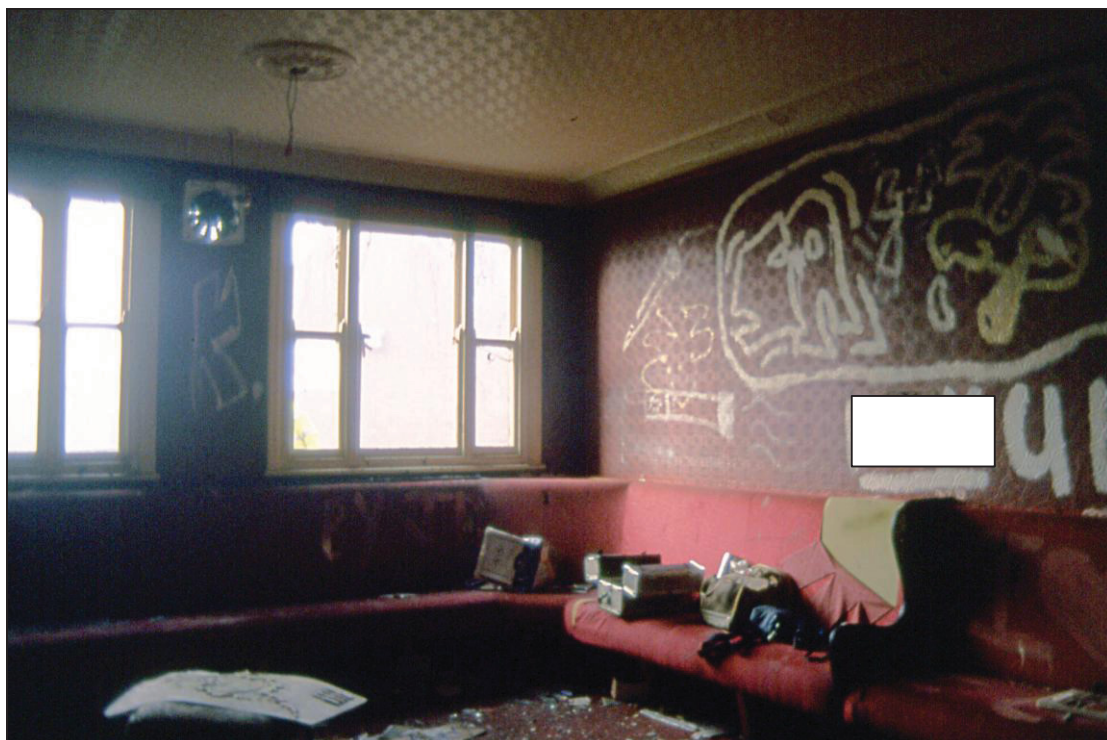
Plate 9 South end, back bar facing west
