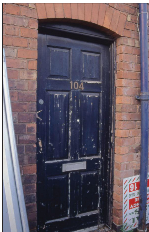
Plate 5 North end, street frontage
