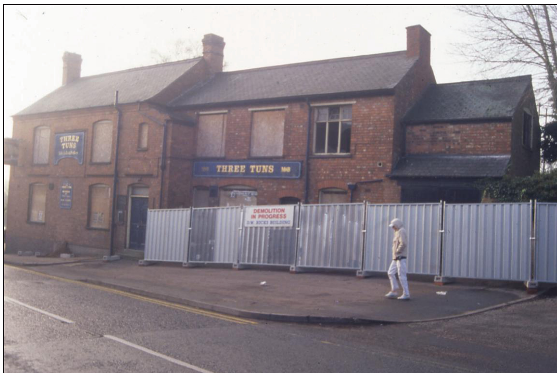
Plate 7 Street frontage, looking west
