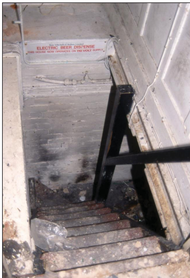
Plate 13 Stairs down to cellar
