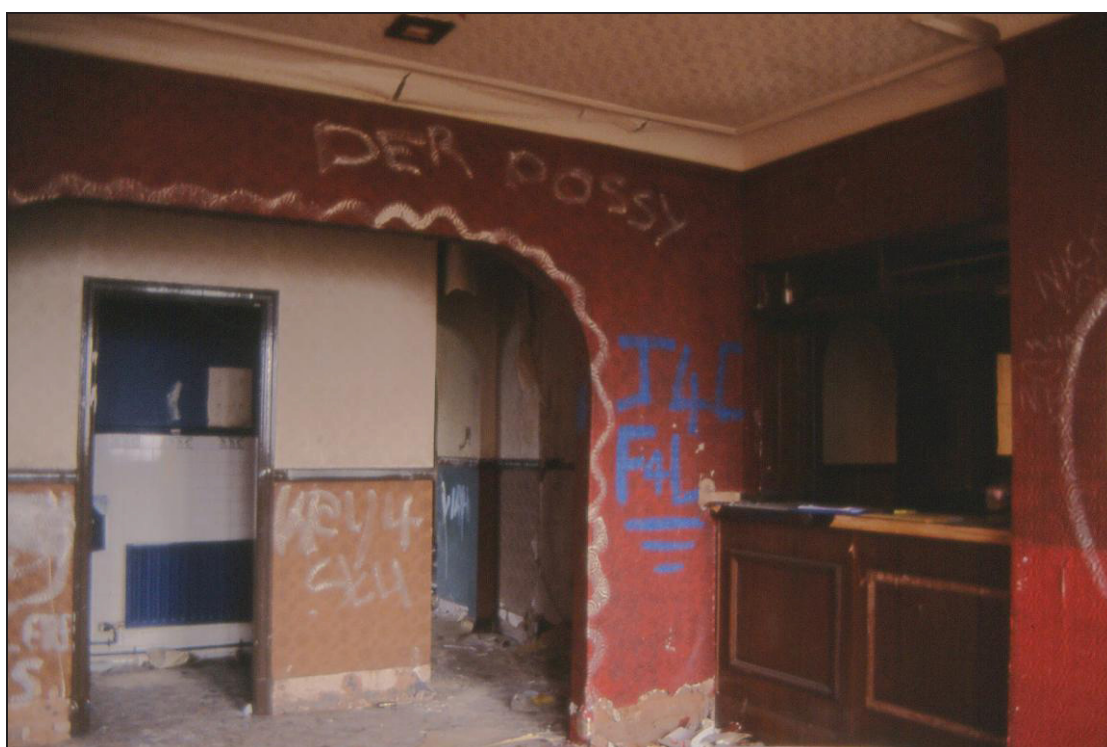
Plate 10 South end, back bar looking north-east
