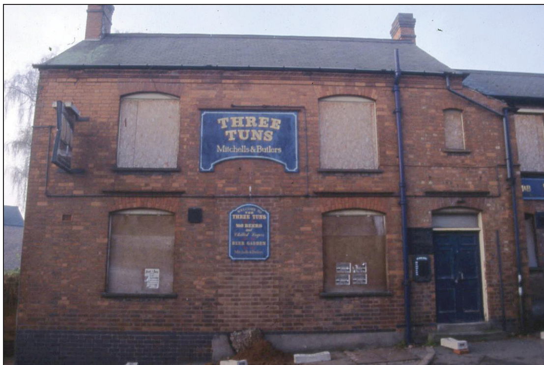
Plate 1 Facade, south end looking west
