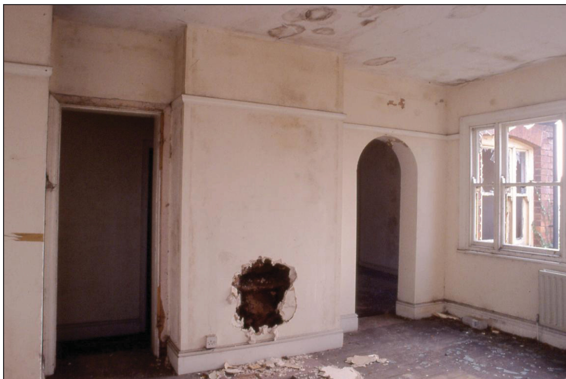
Plate 17 South cross wing, first floor bedroom, looking south east
