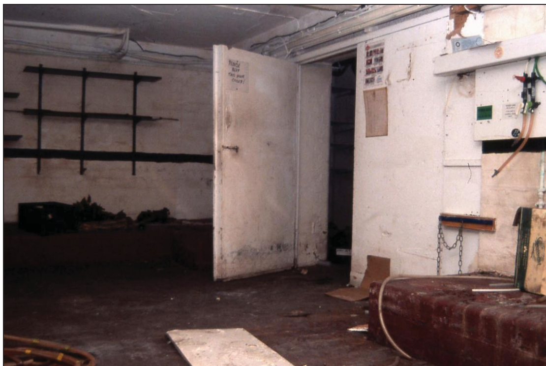
Plate 15 Rear cellar, looking north-east
