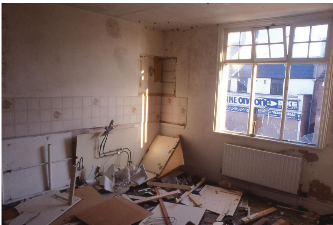
Plate 20 North end, first floor kitchen, looking towards the street
