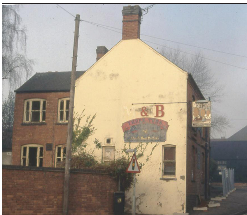
Plate 2 South end, looking north
