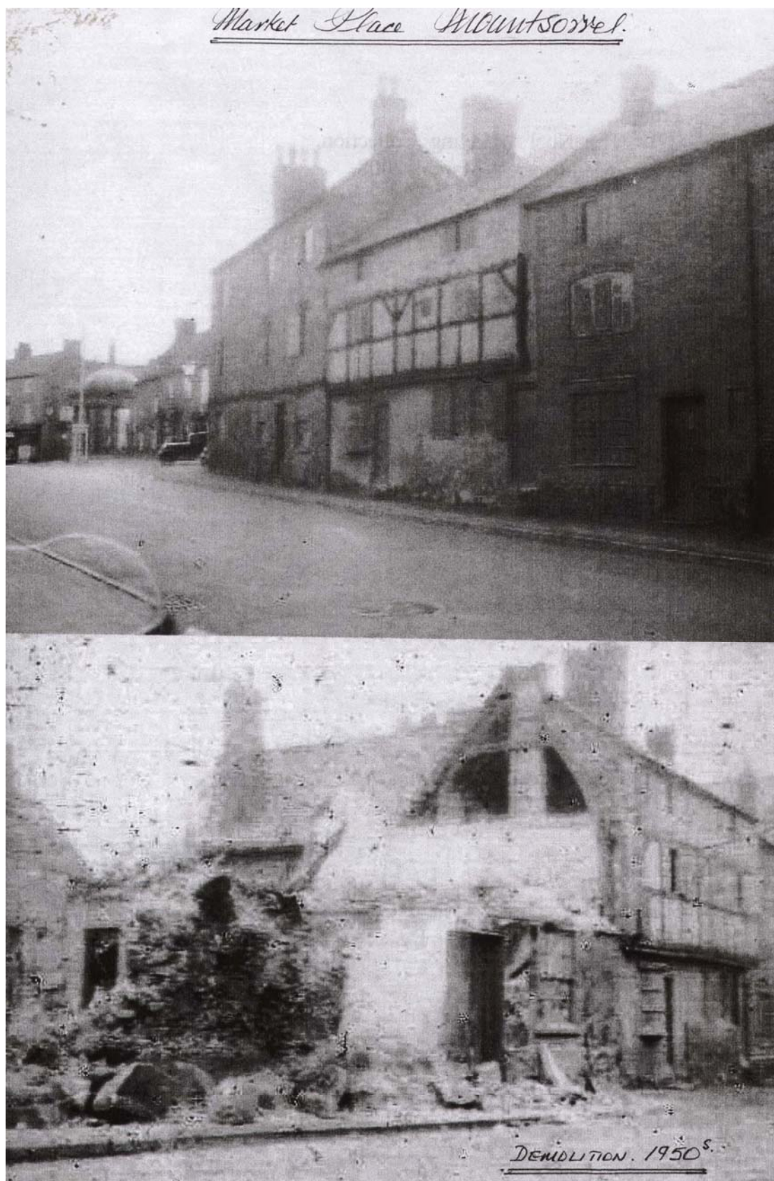
Fig. 17 + 18 The old post office before and after being demolished in the 1950's (Noel Wakeling's private collection)
