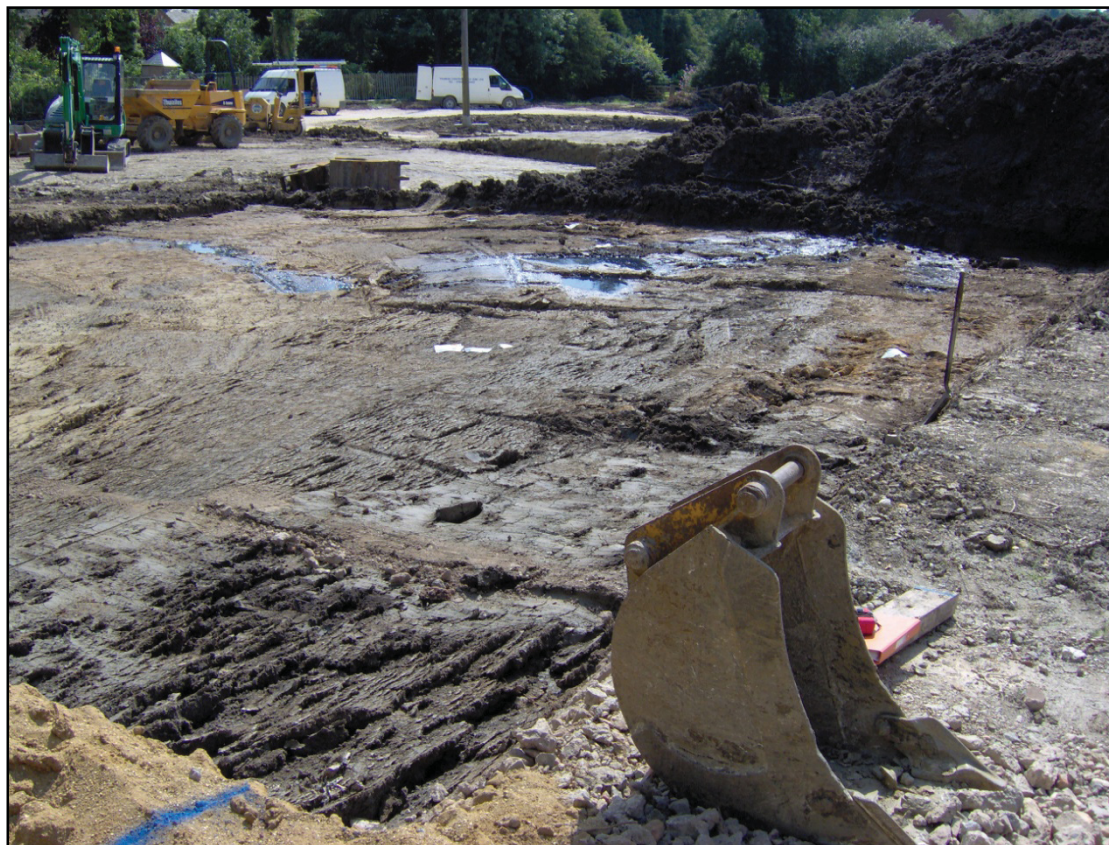
Figure 11. Plot 4 pre-excavation picture.
