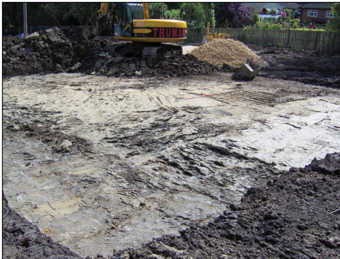
Figure 3. Plot 1 watching brief area. Looking south.
