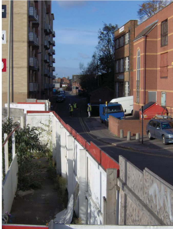
Figure 3: view north along Bath Lane prior to groundwork.
