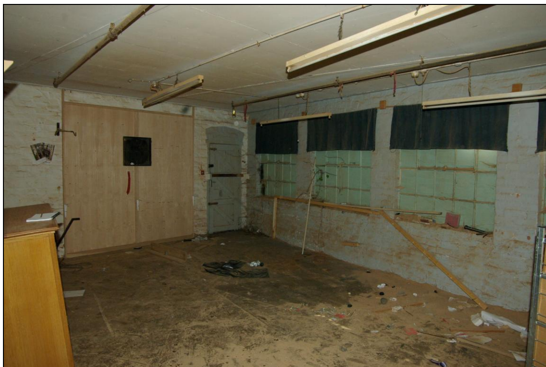
Figure 14. Main building, ground floor. Front windows and north wall. Looking north-east.
