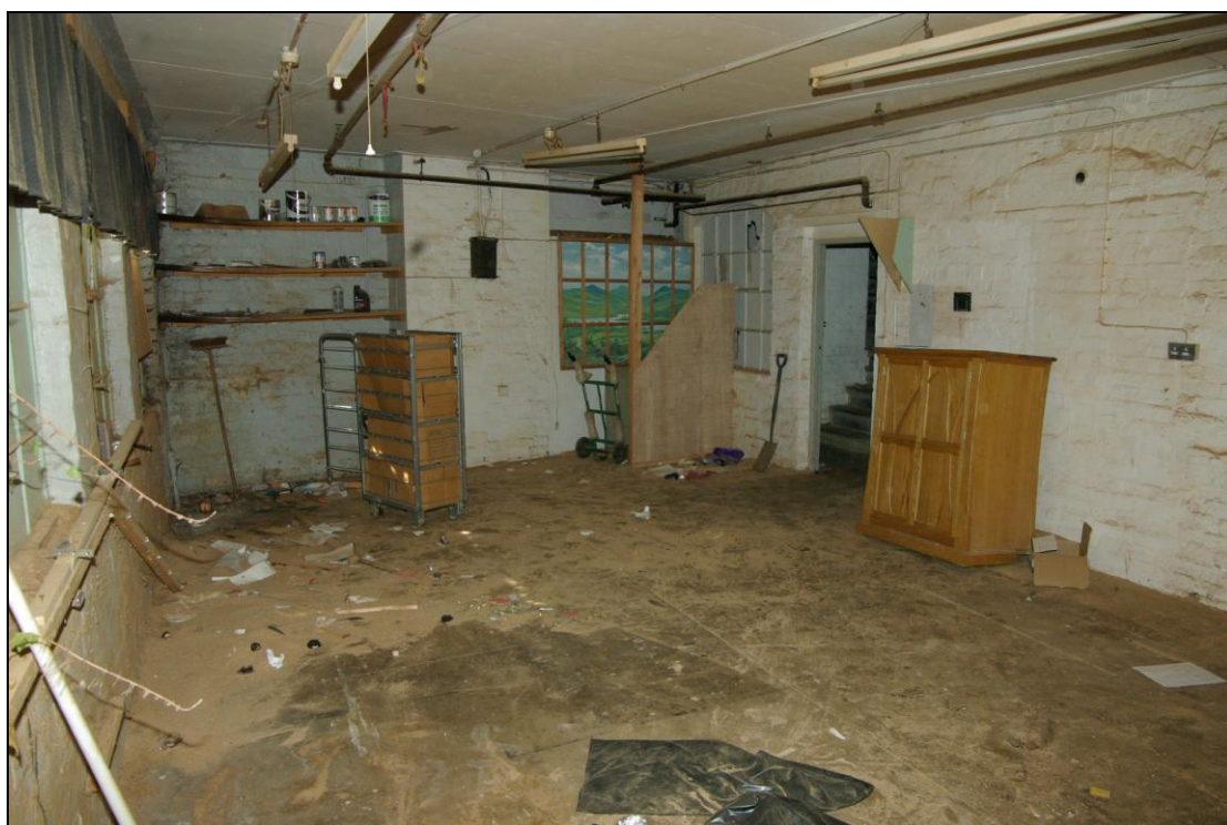
Figure 13. Main building, ground floor. Blocked windows on rear wall and inserted doorway. Looking south-west.
