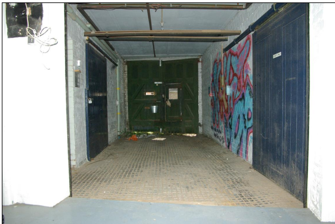
Figure 12. Inside of goods entrance. Looking east.
