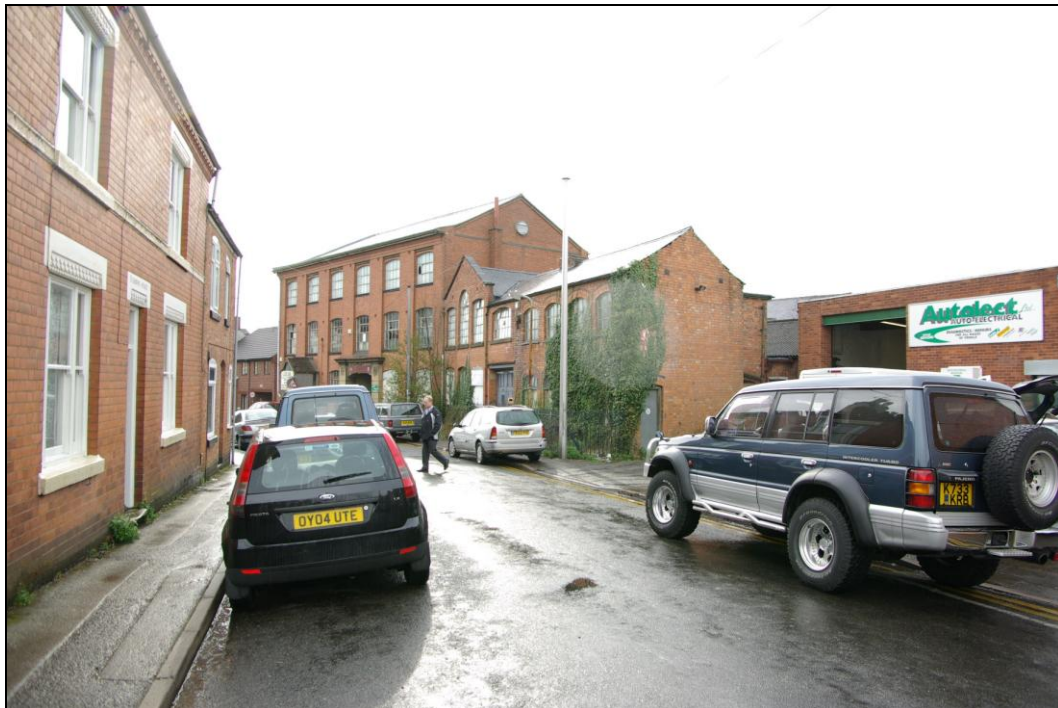
Figure 6. Laban Tansey building and adjacent buildings. Looking south-west down Druid Street.
