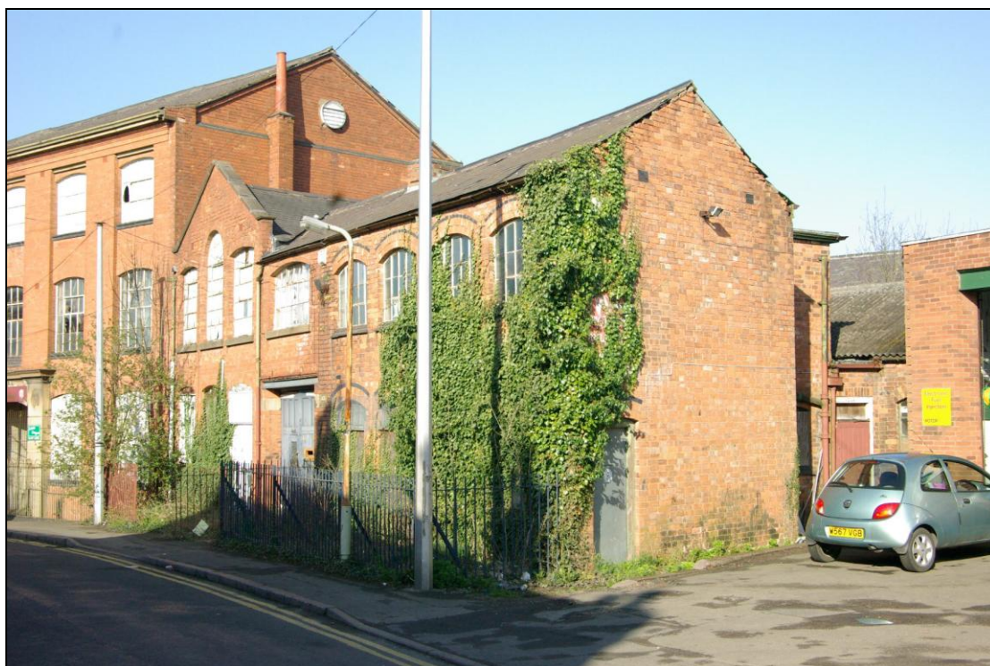
Figure 10. North wall of main building. Looking south-west.
