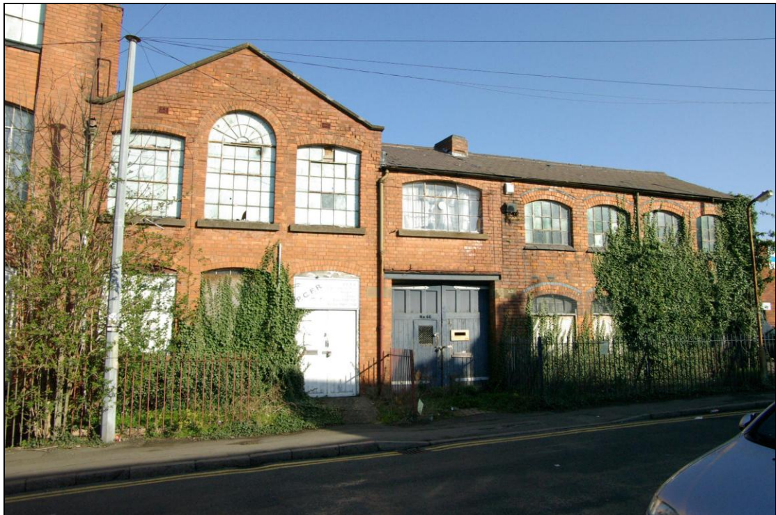
Figure 8. Laban Tansey building. Frontage. Looking west.
