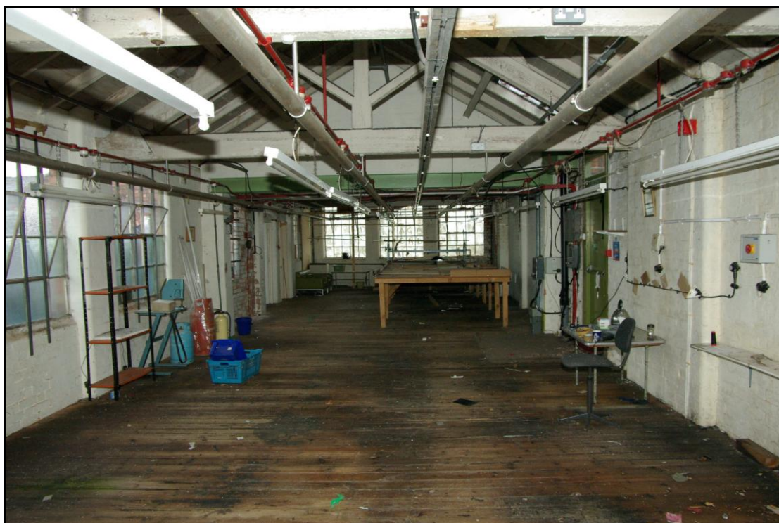
Figure 21. Gable-ended building, first floor. Front windows. Looking east.
