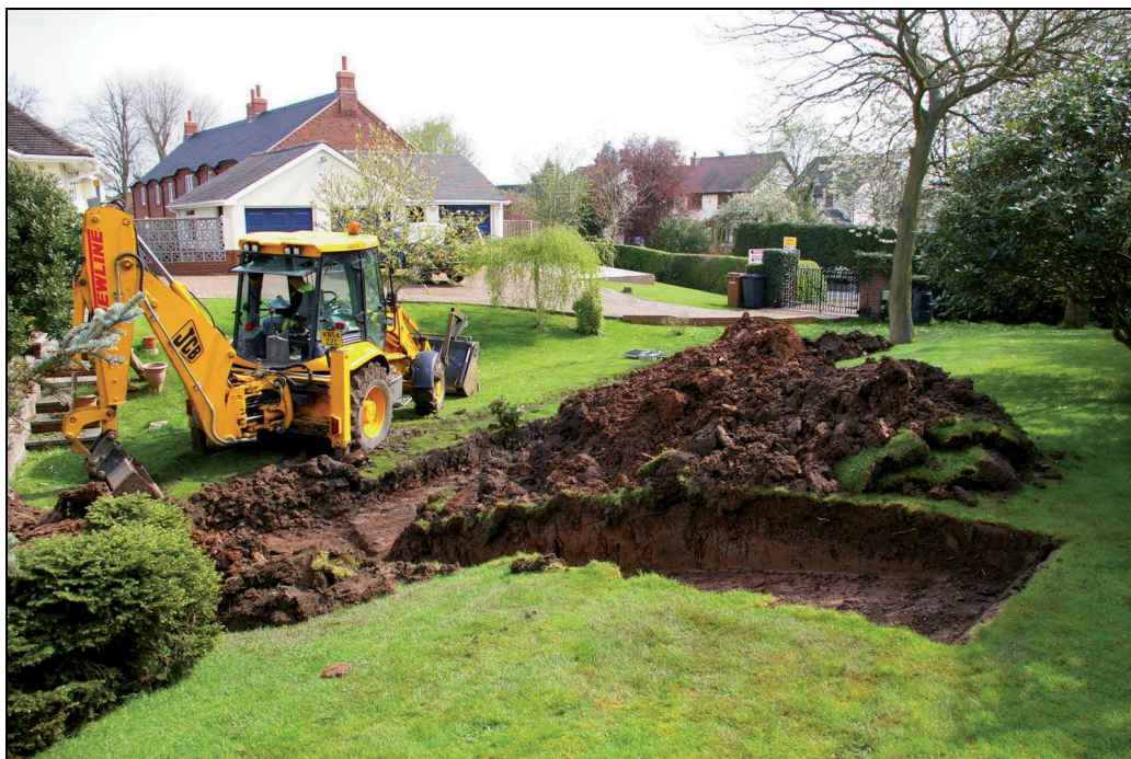
Figure 4: Trench looking north-east, scale 2m.
