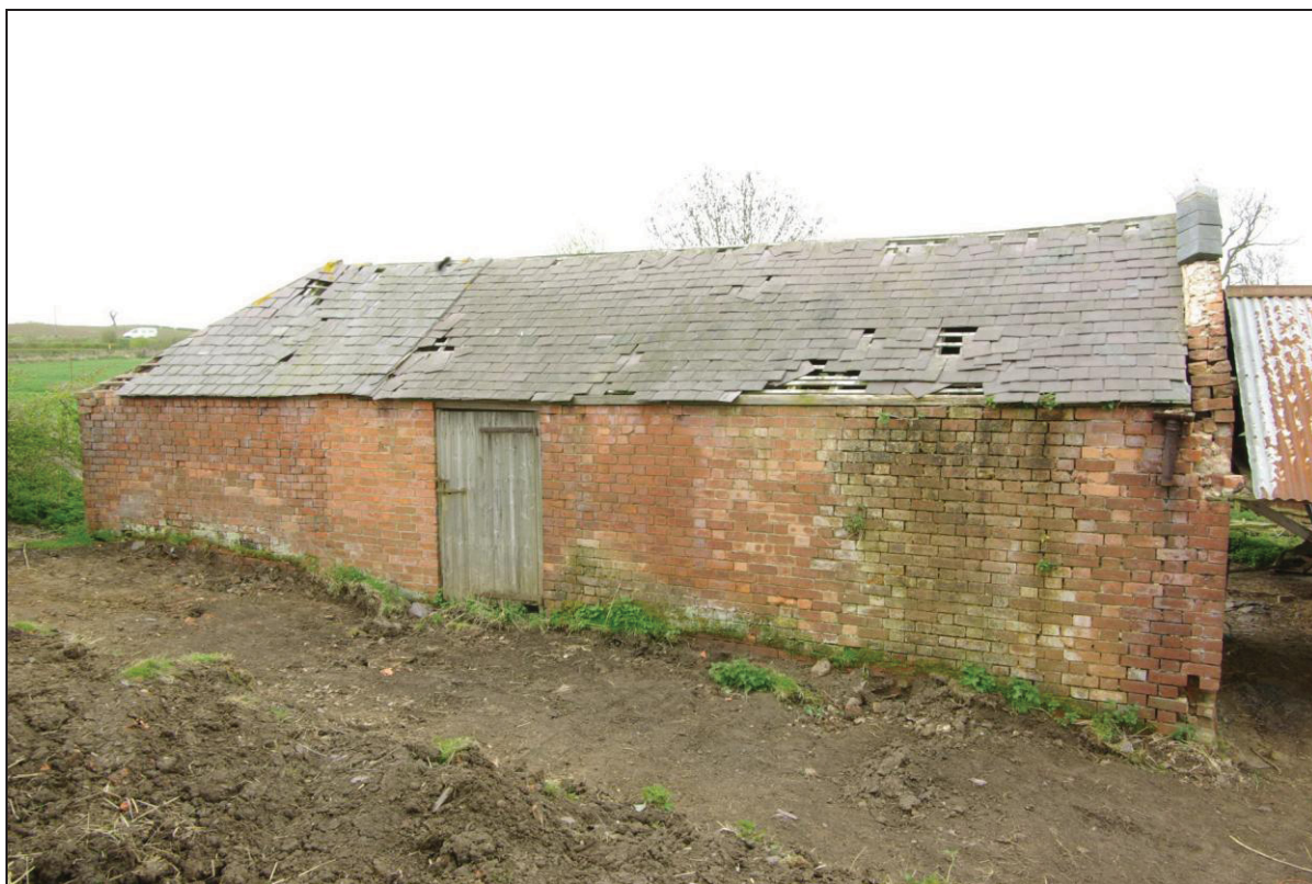
Fig. 7. North elevation of barn.
