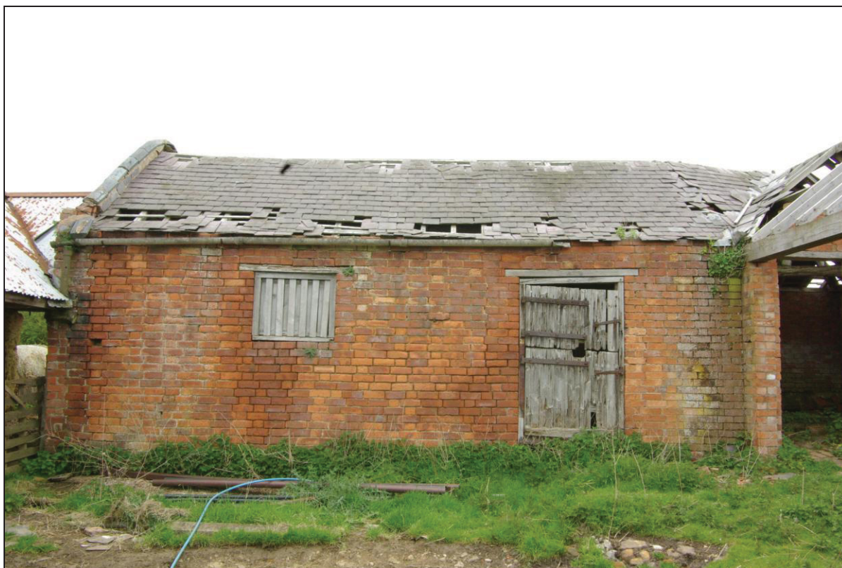
Fig. 13. Barn, south elevation.
