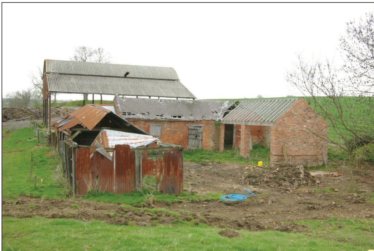
Fig. 6. Barns, looking north-east.
