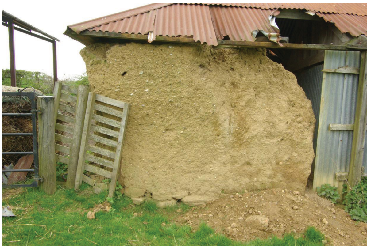
Fig. 10. Cob wall, looking east
