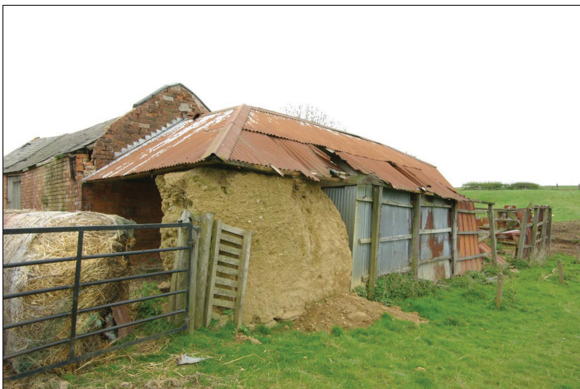
Fig. 11. Cob wall, looking south-east.
