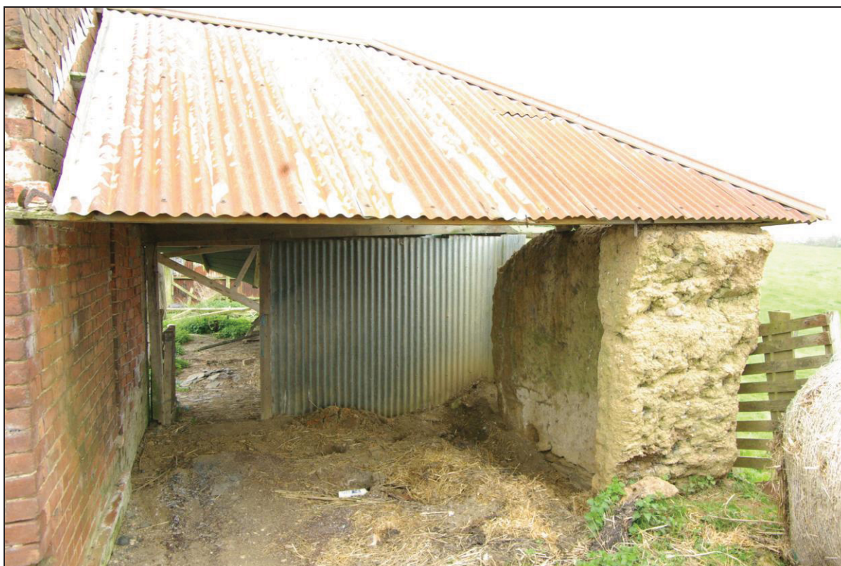
Fig. 8. Cob wall, looking south.
