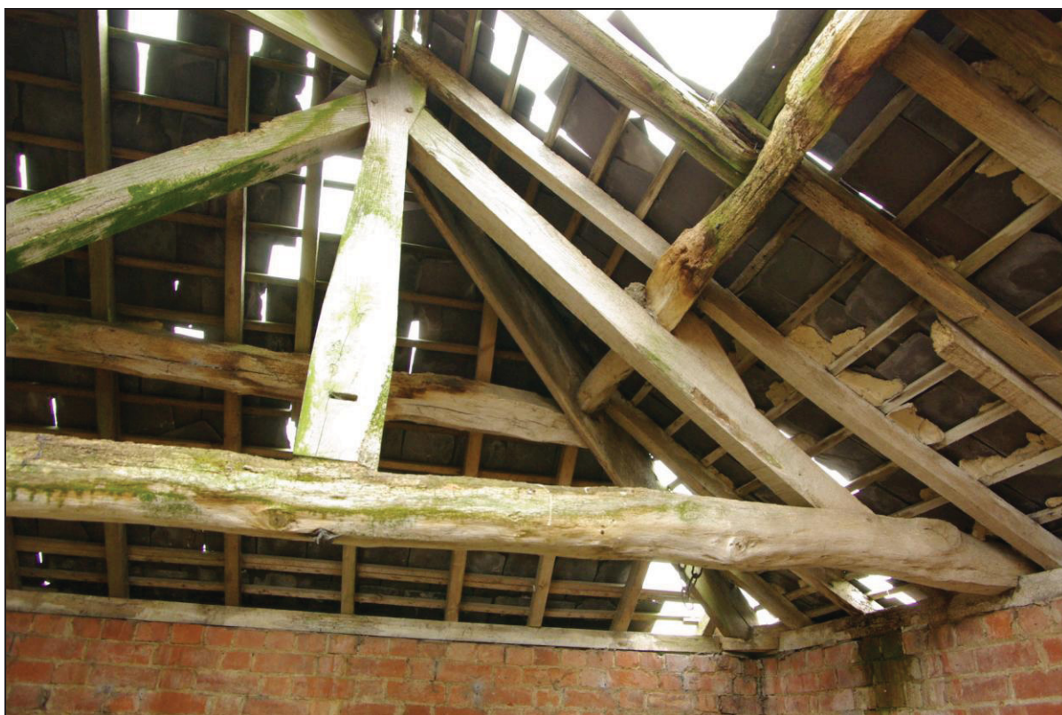
Fig. 14. Roof timbers of barn.
