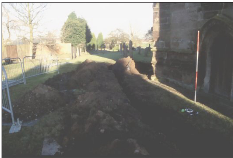
Figure 4: Excavated service trench. Looking north.
