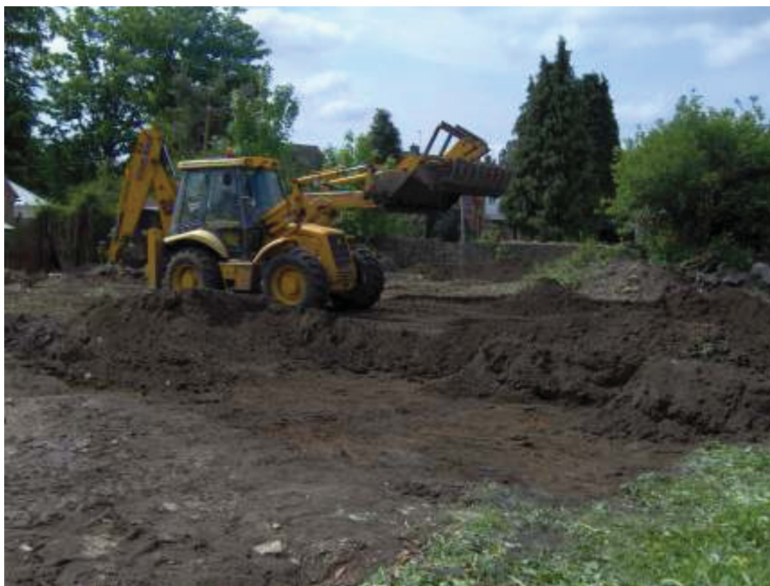
Plate 1: Work in progress, stripping area. Looking south-west.
