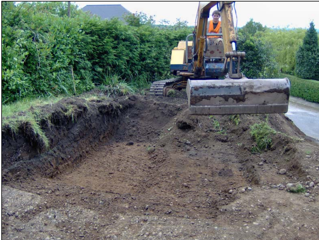
Figure 6: Machining away the overburden on the site.
