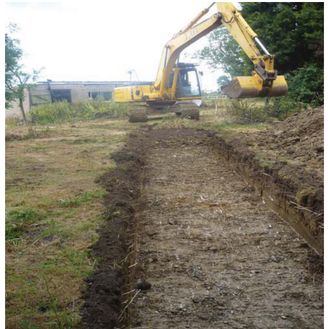
Figure 7: Trench 1 looking south-west
