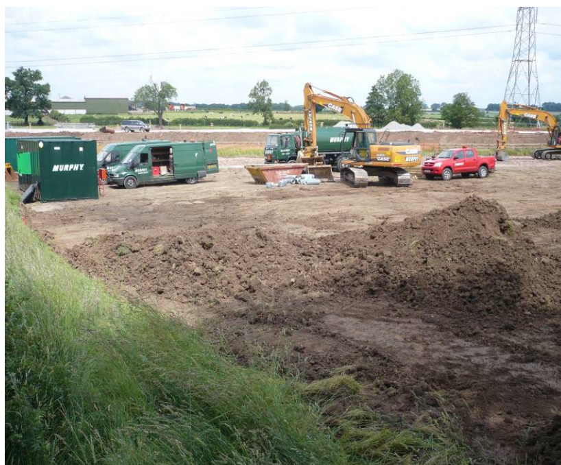
Figure 5: View of area 6/7 from the north-west (see figure 2).
