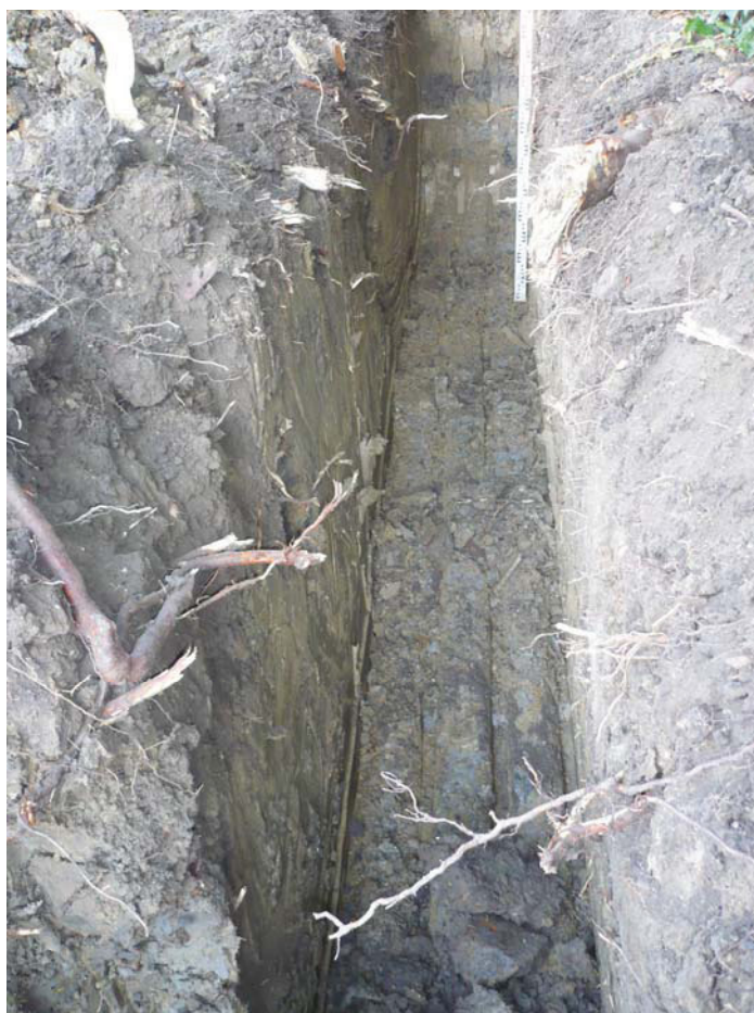
Figure 5: View looking south-west showing westernmost foundation trench
