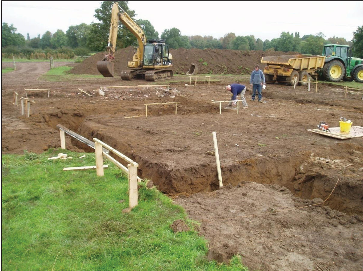
Fig.4 General view of the site facing south
