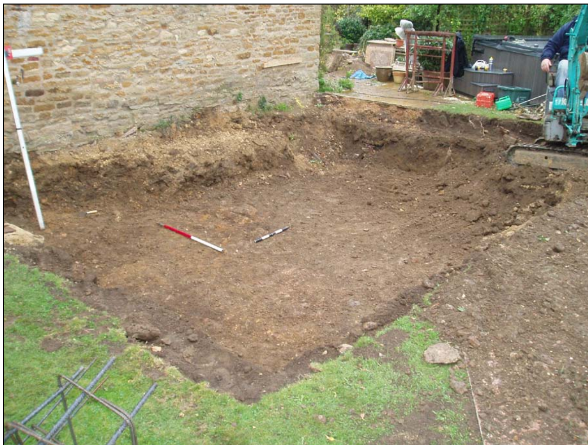
Figure 8 General view south-east facing
