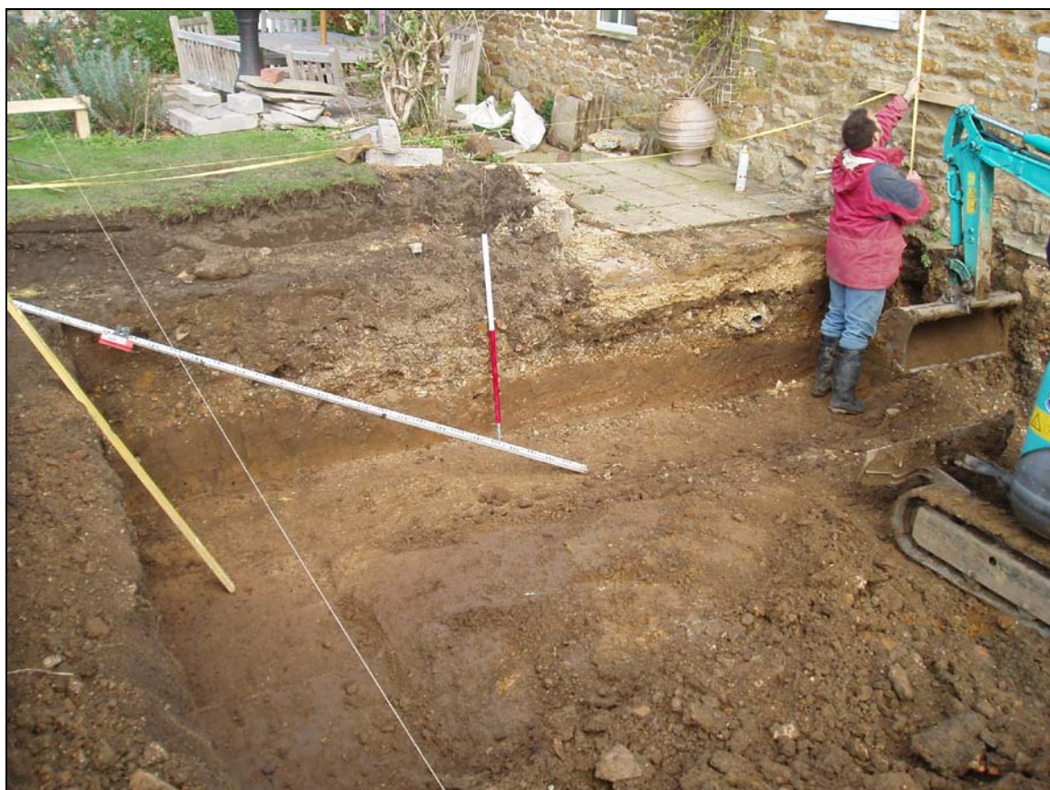
Figure 6 section of trench north facing
