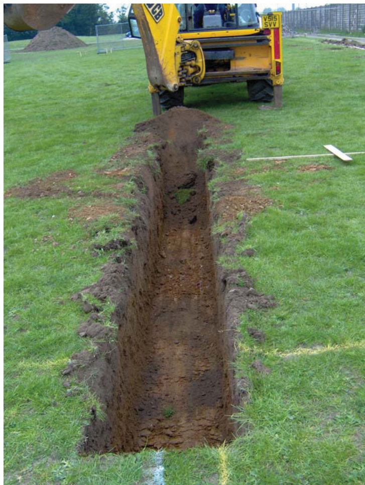
Figure 4: View looking north of foundation trench for internal wall.
