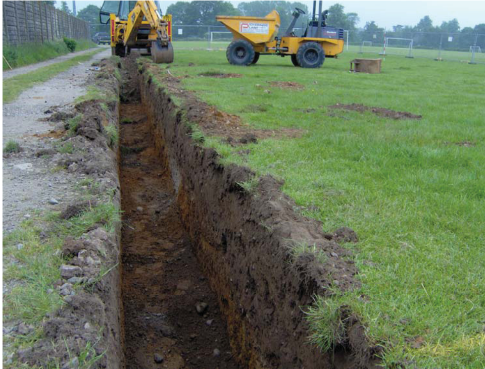
Figure 3: view south of groundwork for foundation trench rear wall
