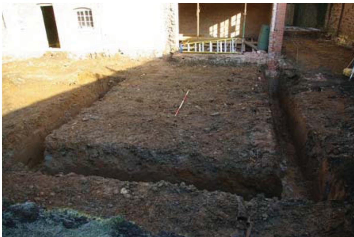
Figure 6 Looking North West after Excavation
