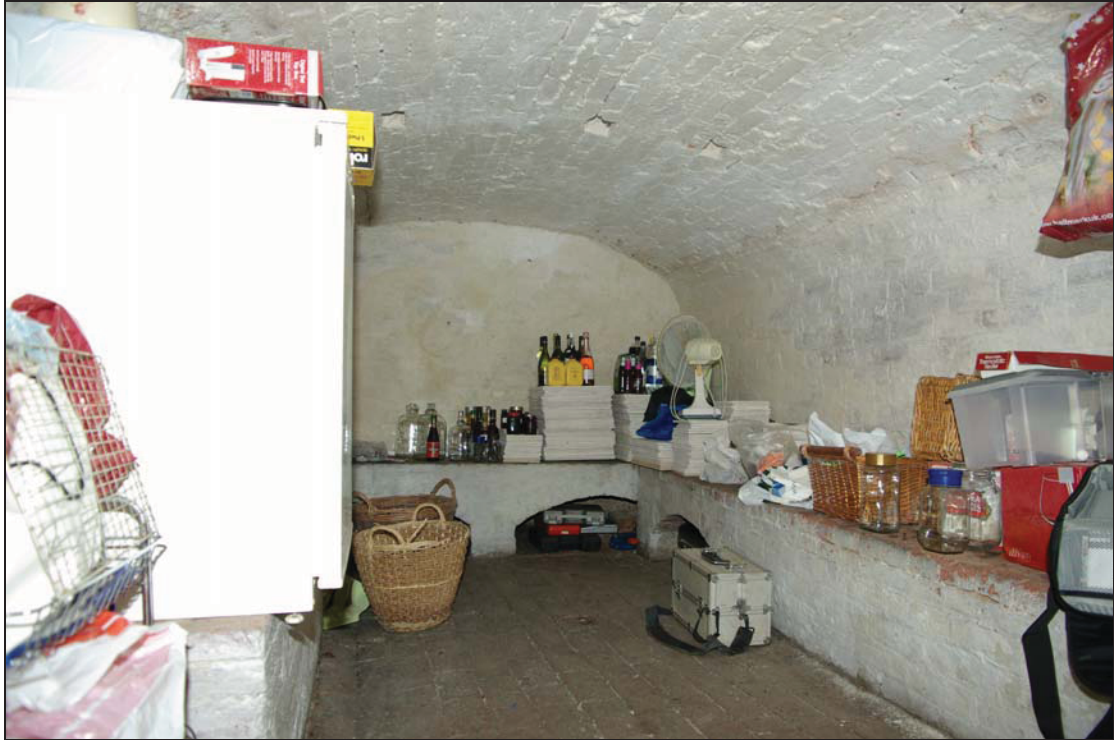
Plate 15. 18 th century cellar, with brick thrall and storage below. Looking east.
