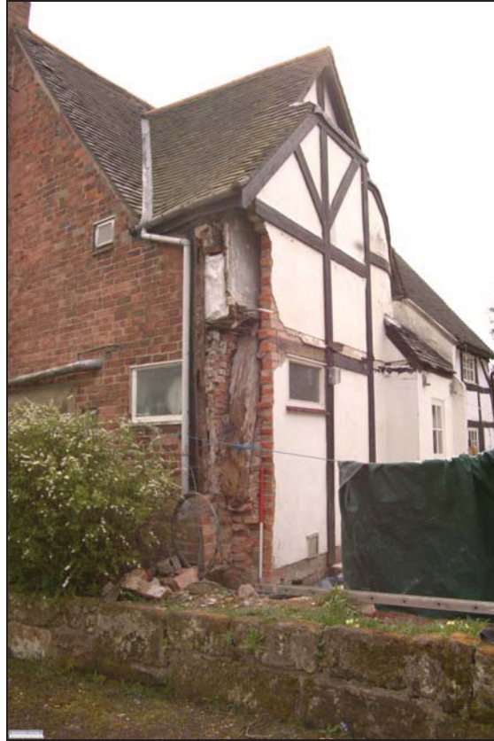
Plate 27. As above, prior to demolition of modern brick façade. Looking southeast.
