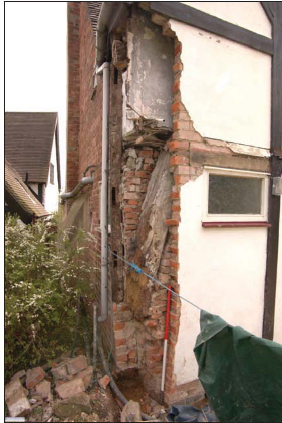
Plate 26. Lower portion of cruck blade revealed behind modern brick façade. Looking east.
