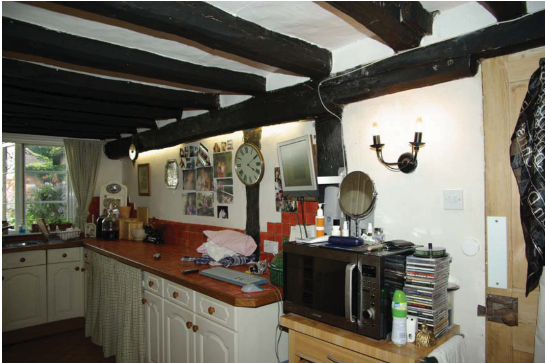
Plate 13. Blocked former doorway leading from service end bay to living kitchen. Looking southeast.
