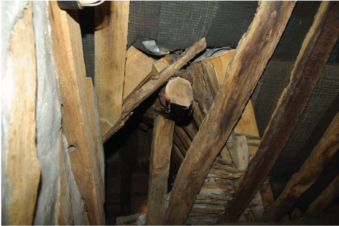
Plate 7. Truncated ridge piece from cruck roof structure. Looking west
