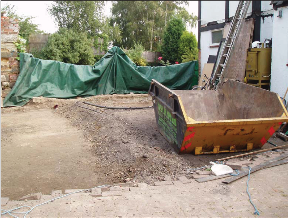
Plate 22. The excavation area, with 24 High Street visible to east. Looking north
