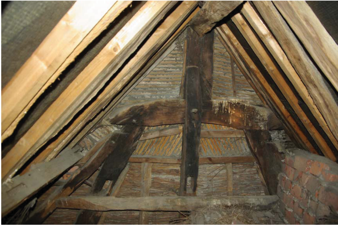
Plate 5. Upper portion of cruck frame, seen within roof space. Looking west.
