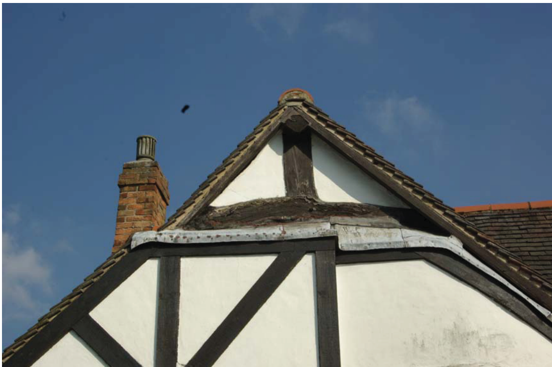
Plate 4. Detail of Cruck apex. Looking east.
