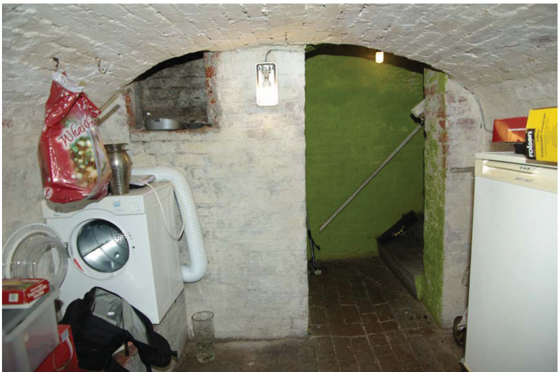
Plate 16. Cellar, with ventilated alcove and stairs up to kitchen. Looking west.
