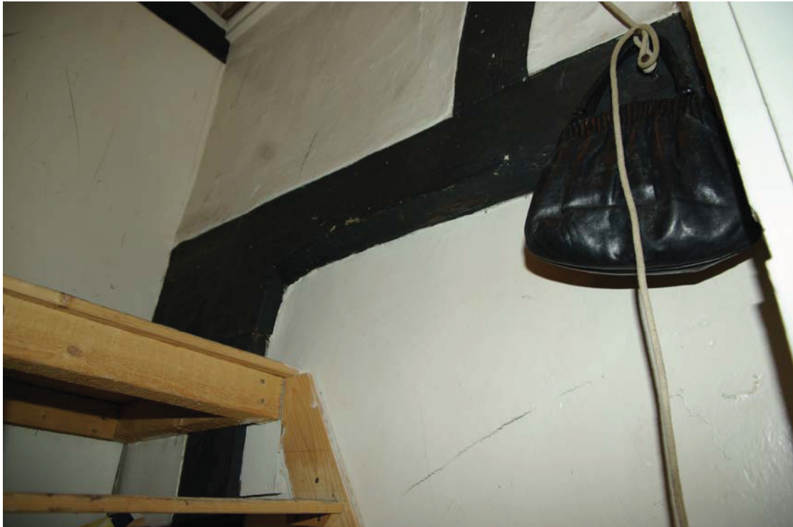
Plate 11. Early doorway through truss of box-framed structure.
