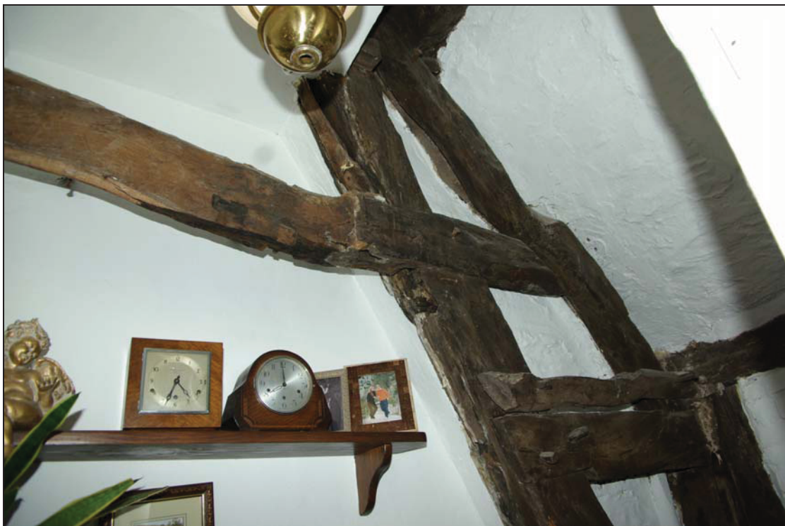
Plate 6. Lower portion of cruck, seen above stairwell. Looking northwest
