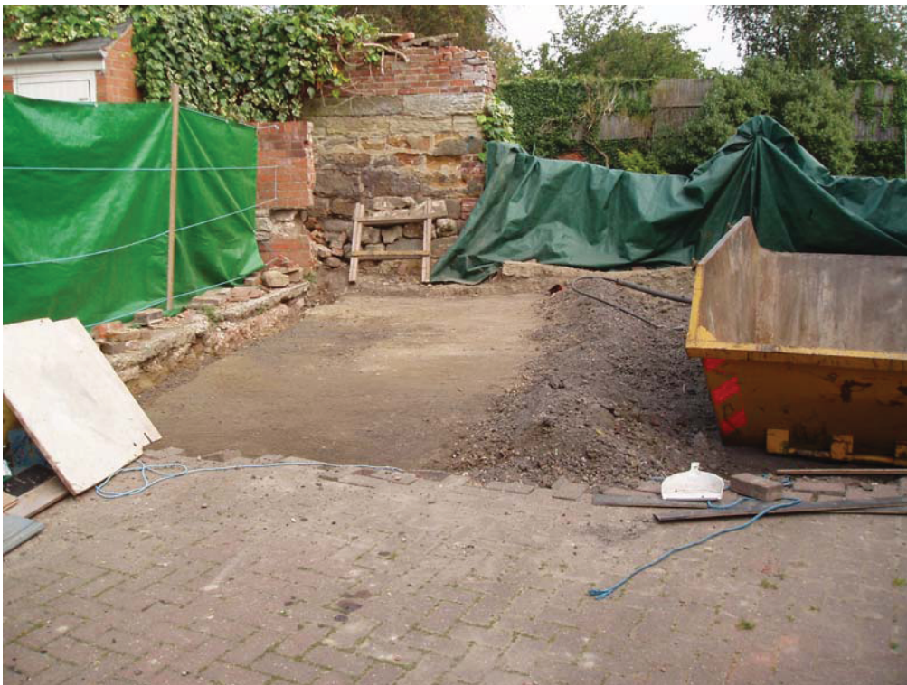
Plate 23. Excavation area following clean-up. Looking north.
