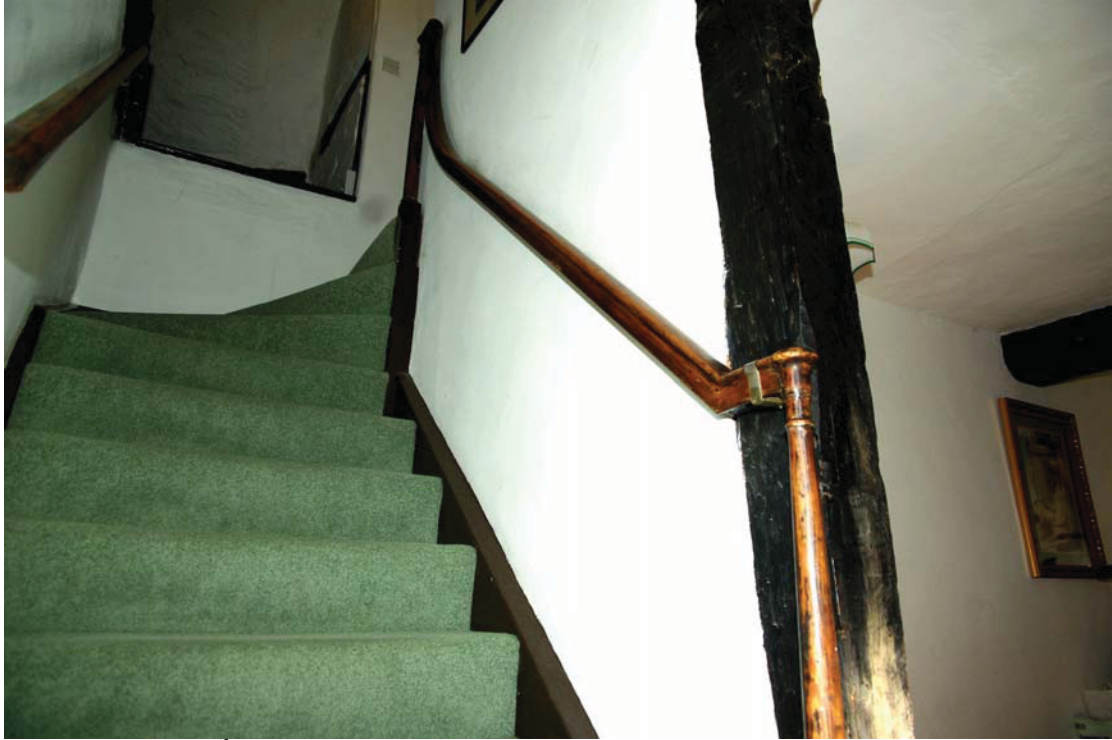
Plate 19. 18 th century staircase, with ramped handrail and turned newels. Looking northeast.
