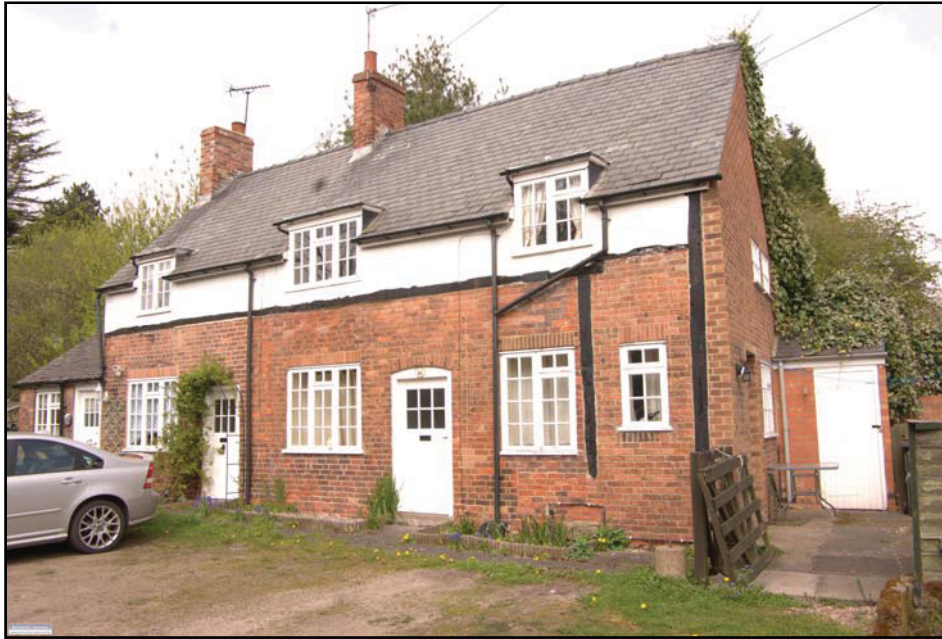
Plate 21. 26 and 28 High Street, with evidence of early timber frame. Looking north.
