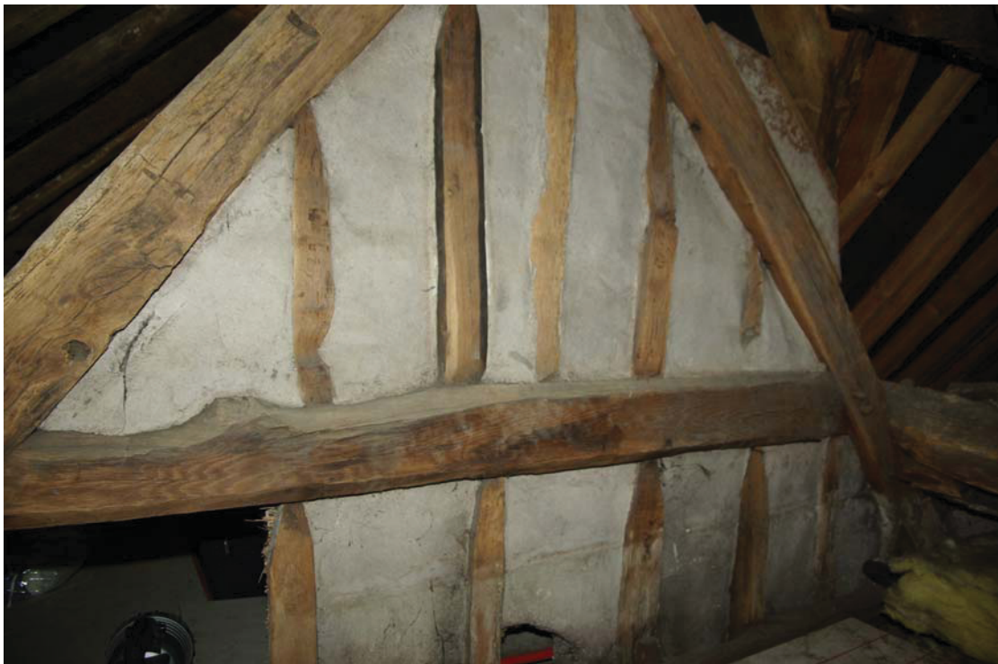
Plate 10. Closed roof truss, within box-framed structure. Looking south.
