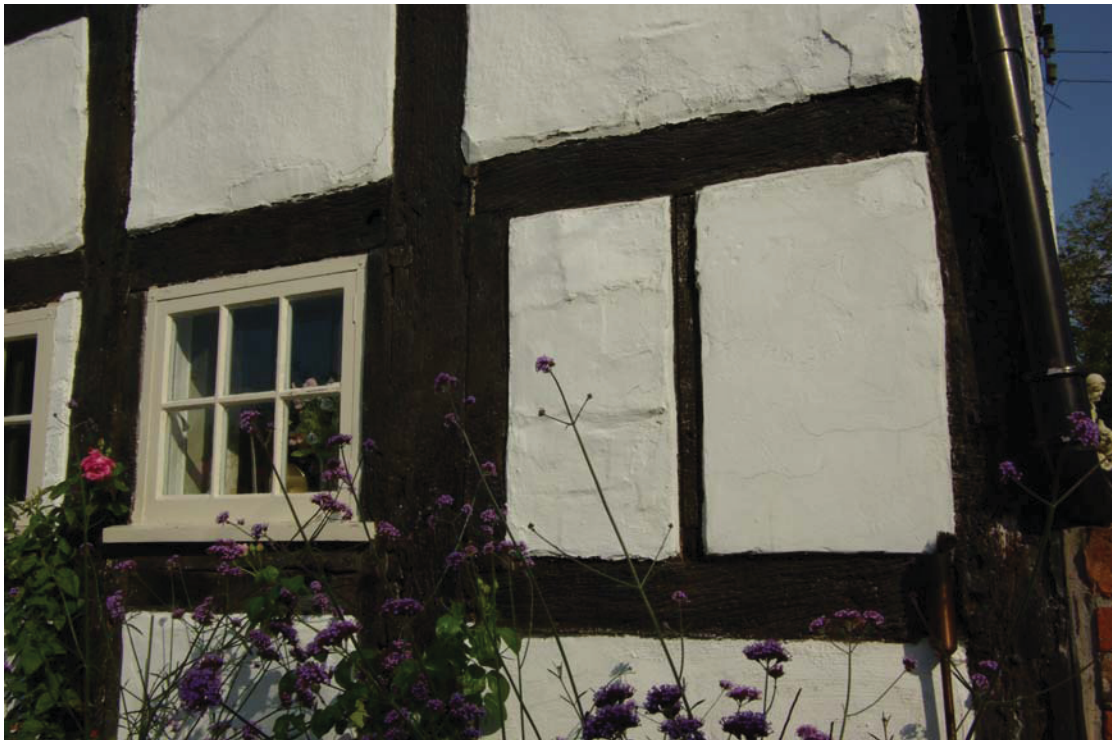
Plate 2. Early blocked window within timber frame. Looking east.
