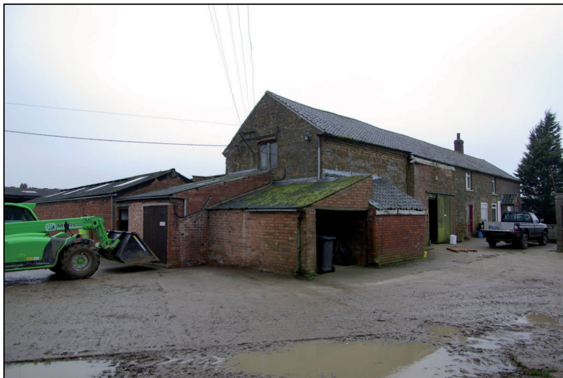
Figure 7 North and east faces of barn, farmhouse and outbuildings. Facing south west.
