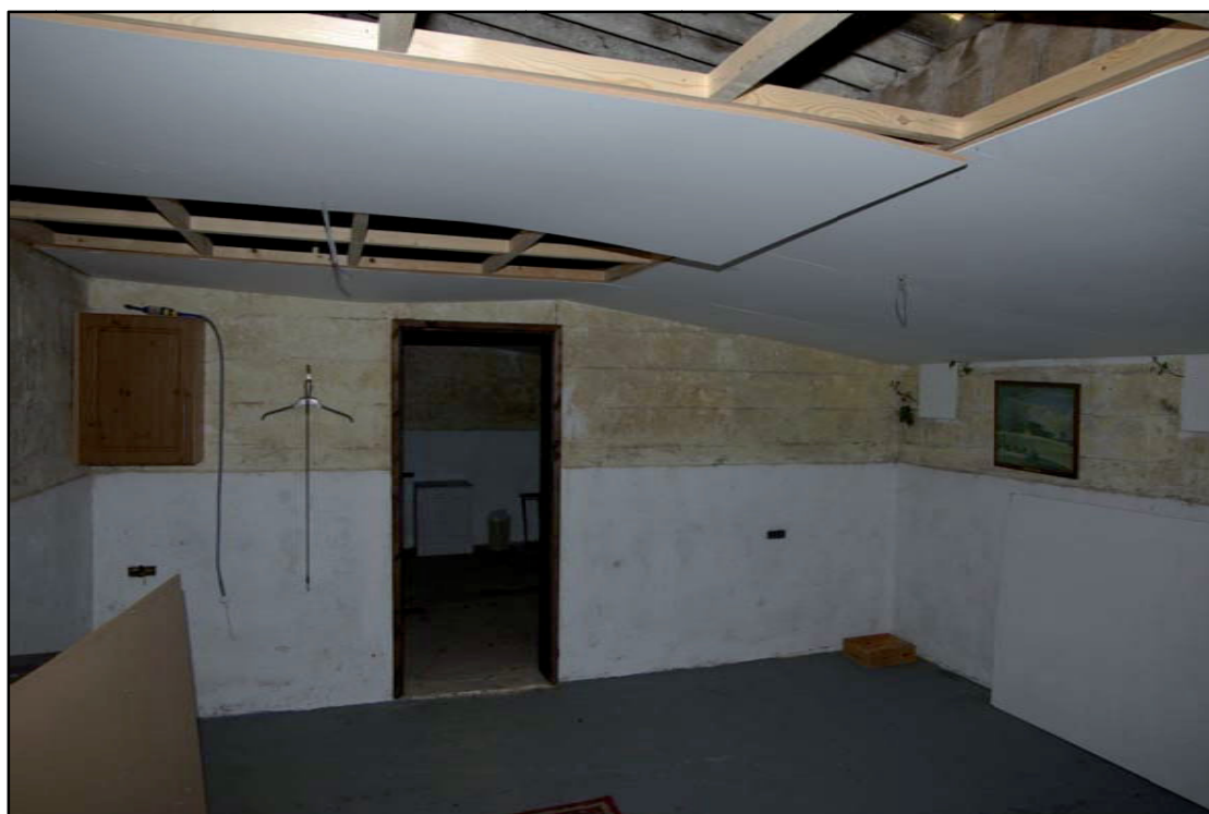
Figure 19 Stable converted to utility room. Facing south.
