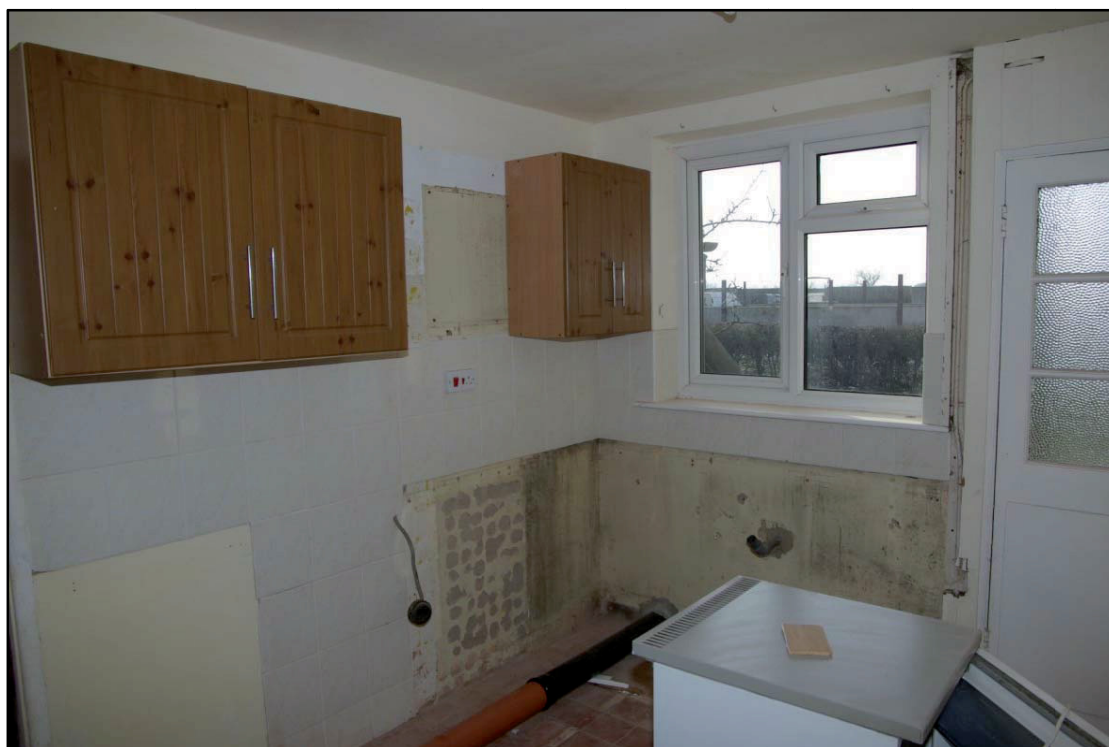
Figure 18 Ground floor of gable extension. Facing south west
