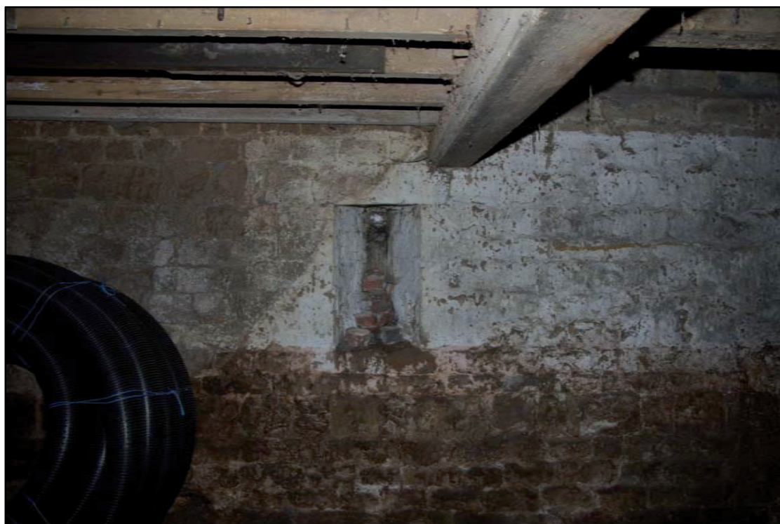
Figure 9 Blocked splayed window. South side of barn.
