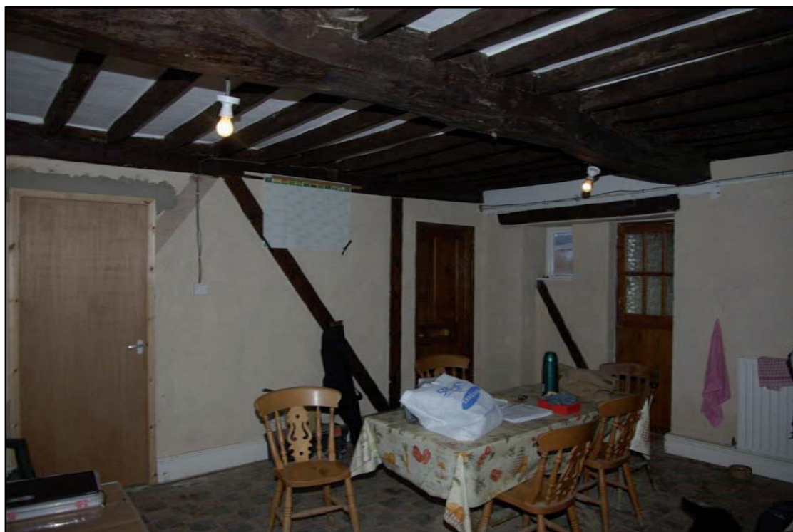
Figure 16 Main ground floor room. Facing south east.
