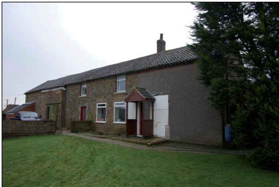
Figure 14 North face of farmhouse.
