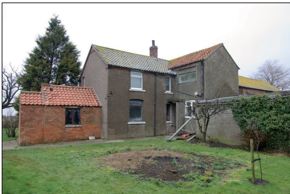
Figure 35 Rear of stable, outhouse and farmhouse extension. Facing north east.
