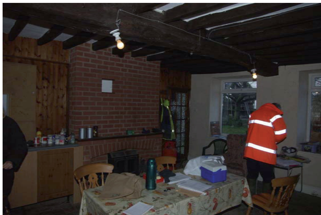
Figure 17 Main ground floor room. Facing north west.
