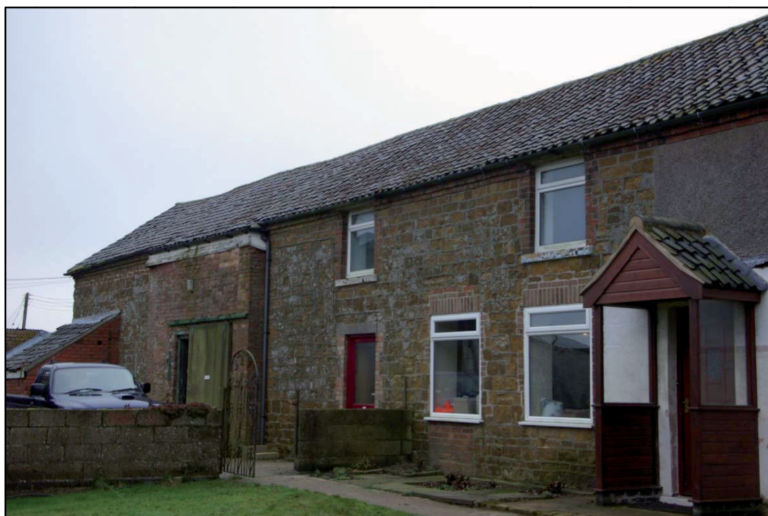
Figure 15 Original portion of farmhouse. Blocked doorway in centre.
