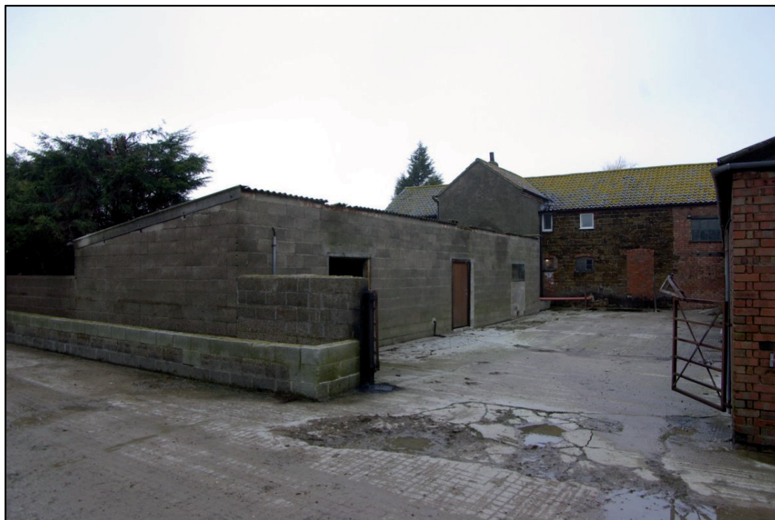
Figure 34 Stable block. Facing north west.
