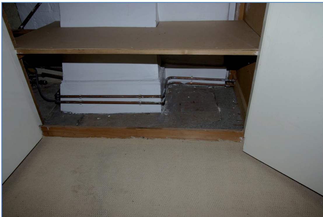
Figure 26 First floor centre room. Bricks around chimney breast.
