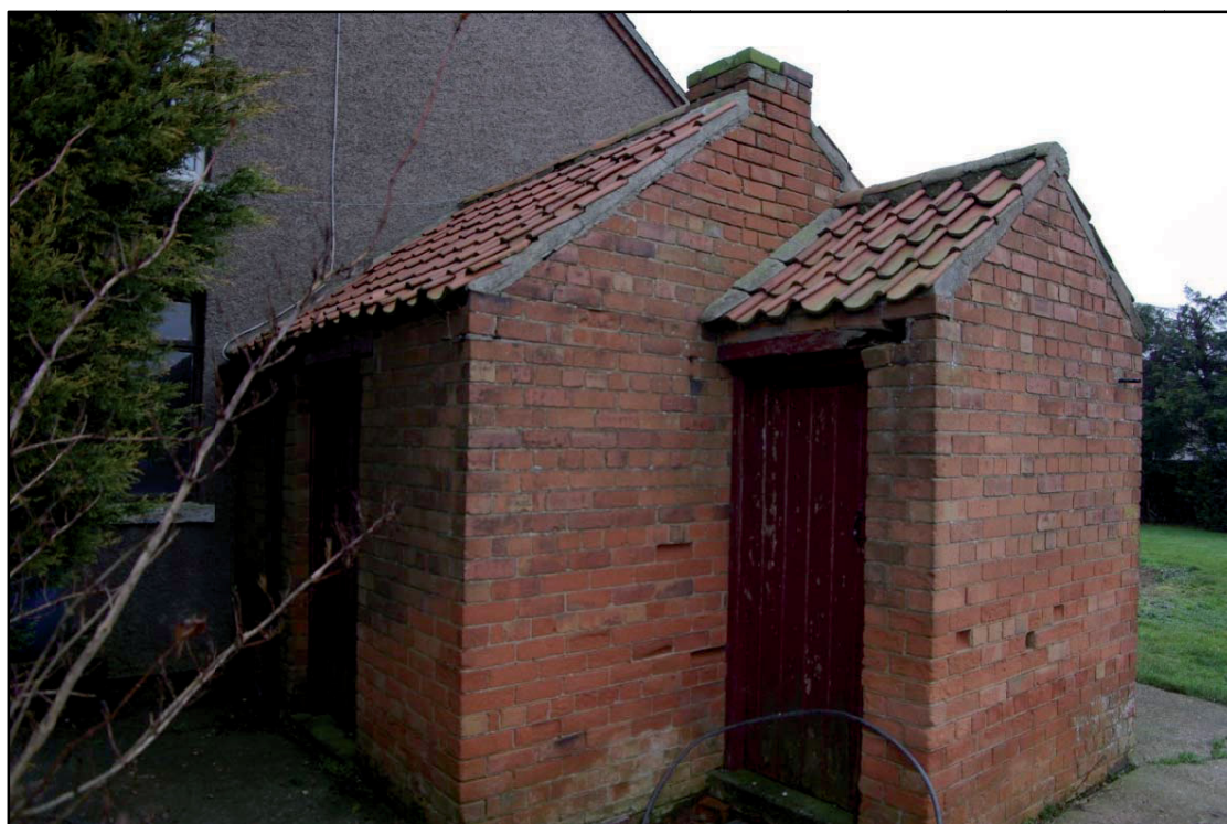
Figure 29 Outhouses at western end of farmhouse. Facing south east.
