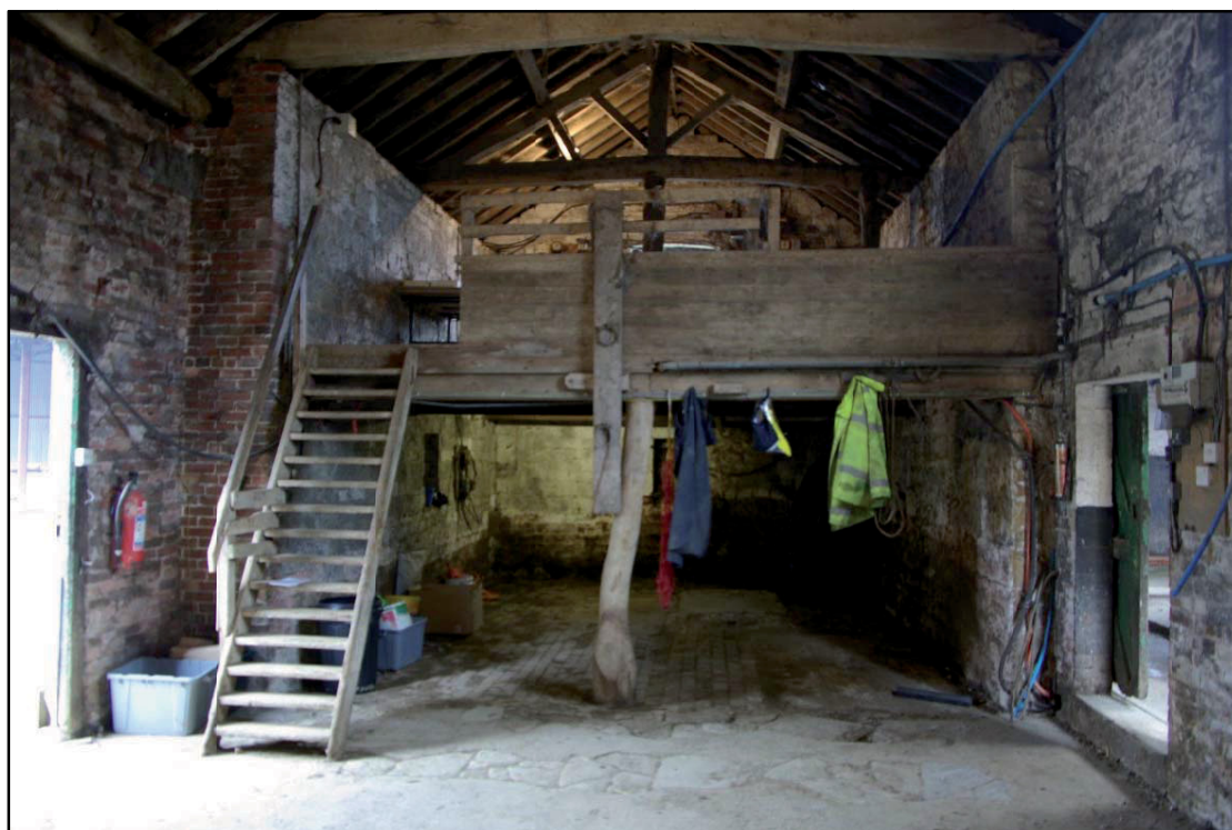
Figure 12 East end of threshing barn and mezzanine.
