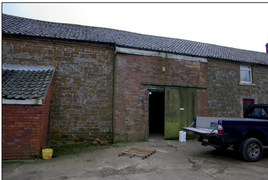
Figure 8 Blocked door of threshing barn. Facing south.
