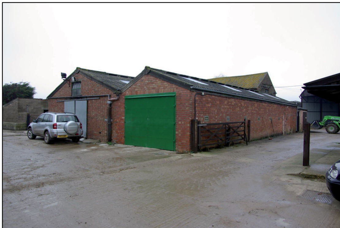
Figure 32 Shed attached to milking parlour. Facing north west.
