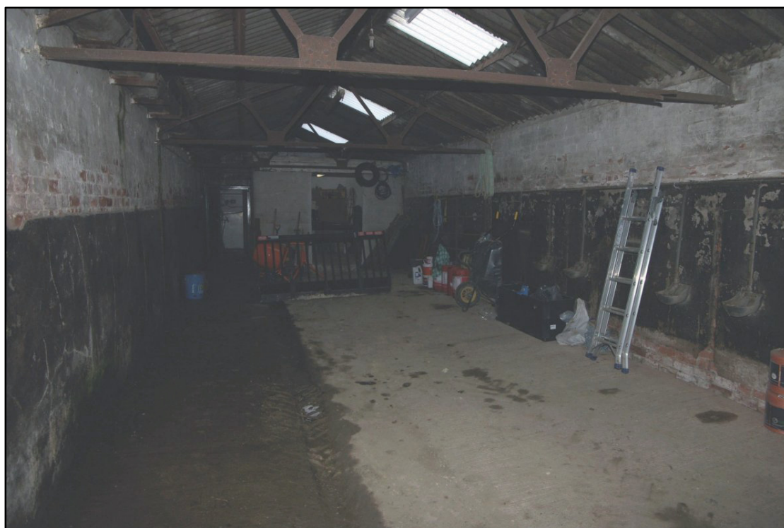
Figure 33 Inside shed. Facing north.
