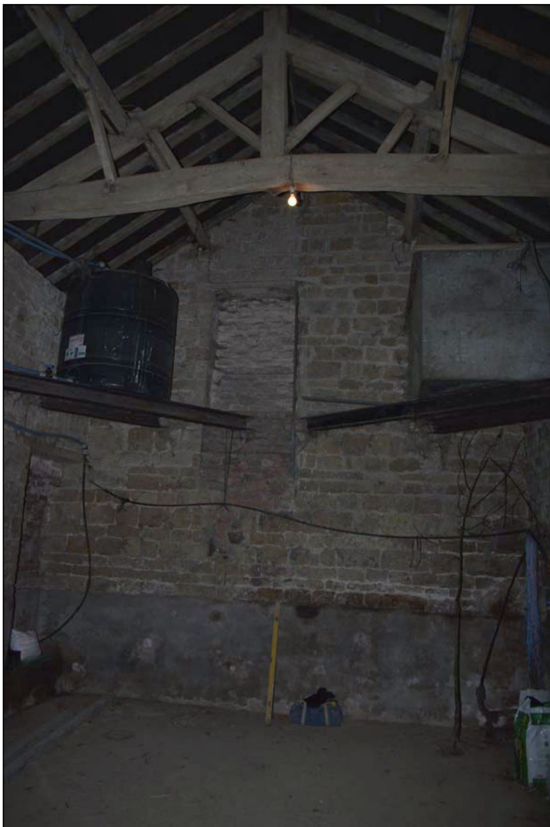
Figure 11 West end of threshing barn.
