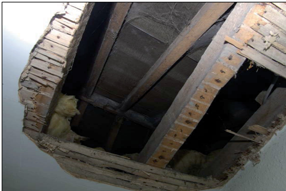
Figure 28 First floor, eastern room. Roof detail.
