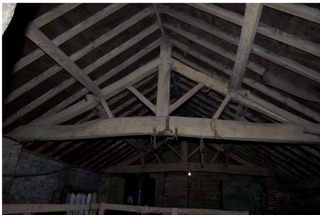
Figure 13 Roof structure of threshing barn. Facing west.
