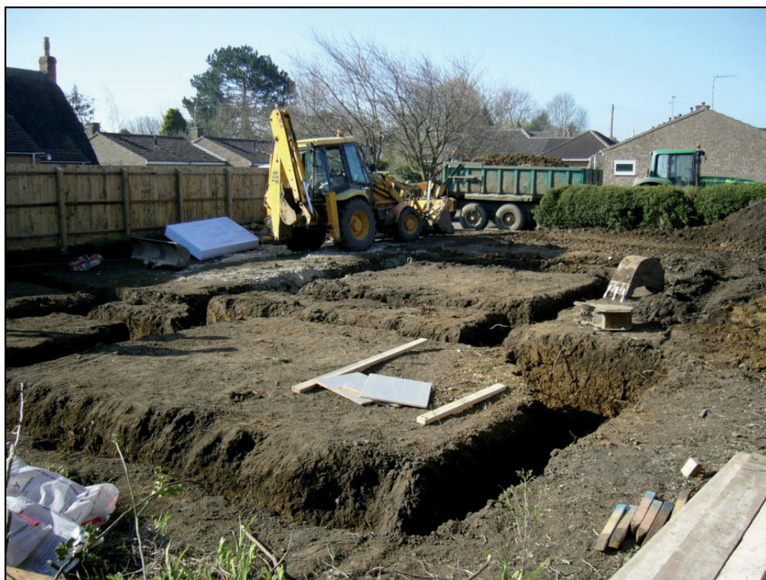
Figure 5. Site after excavation of foundations. Facing South east.
