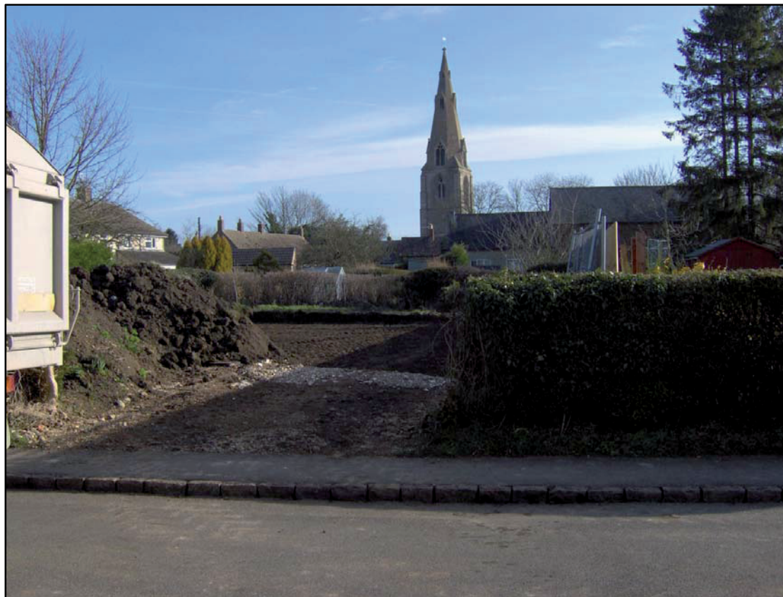
Figure 4. Site from Bridge Street after topsoil strip. Facing north west.
