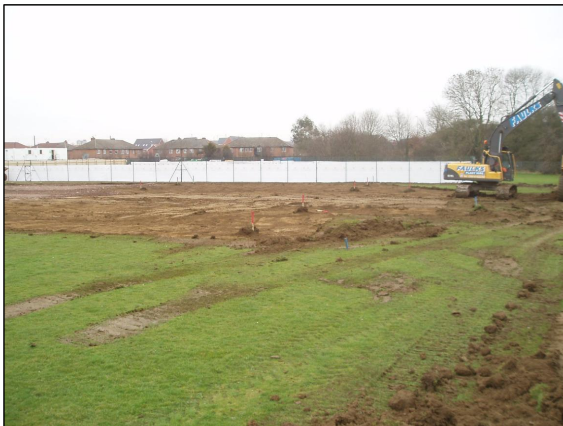
Figure 5. Southern area of site. Facing north east.
