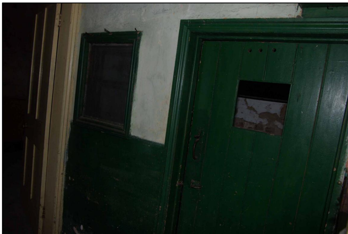
Figure 11. Pantry door and window. Looking south-east.
