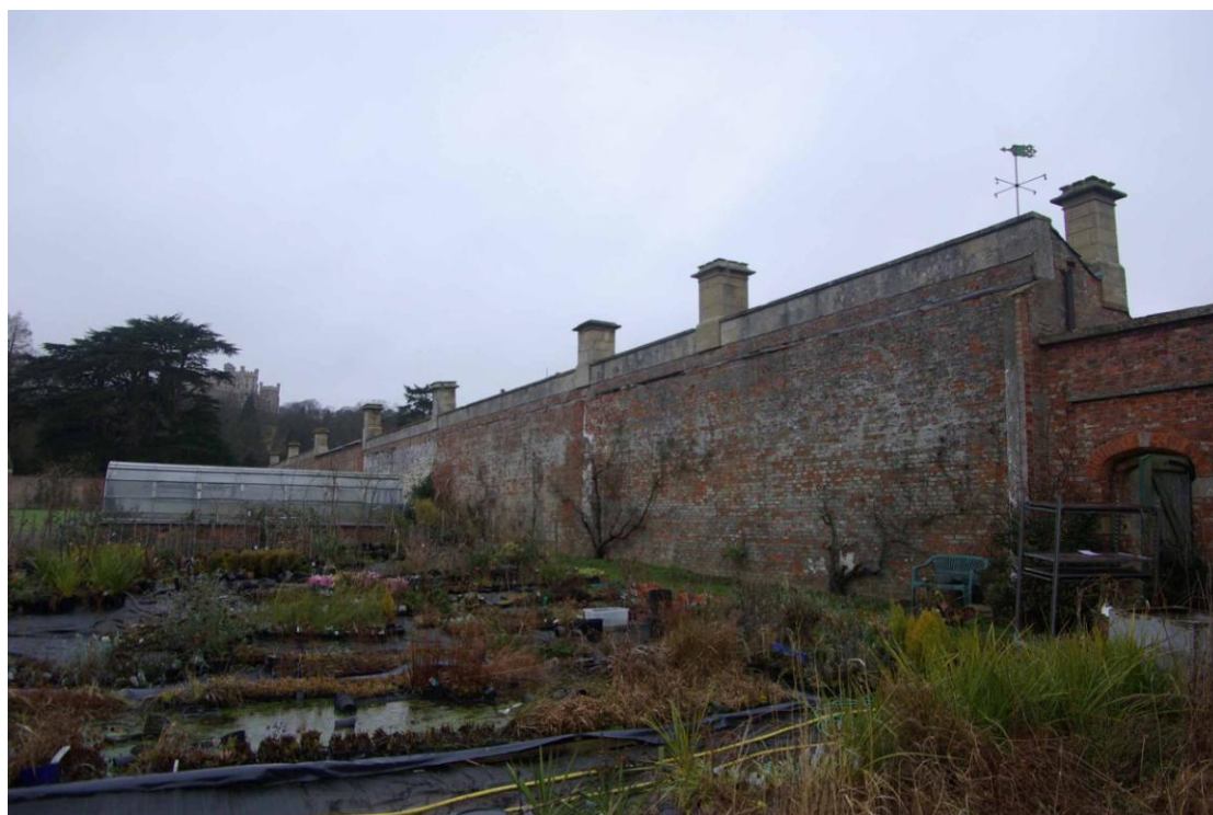
Figure 8. South wall of bothy from walled garden. Looking north west.
