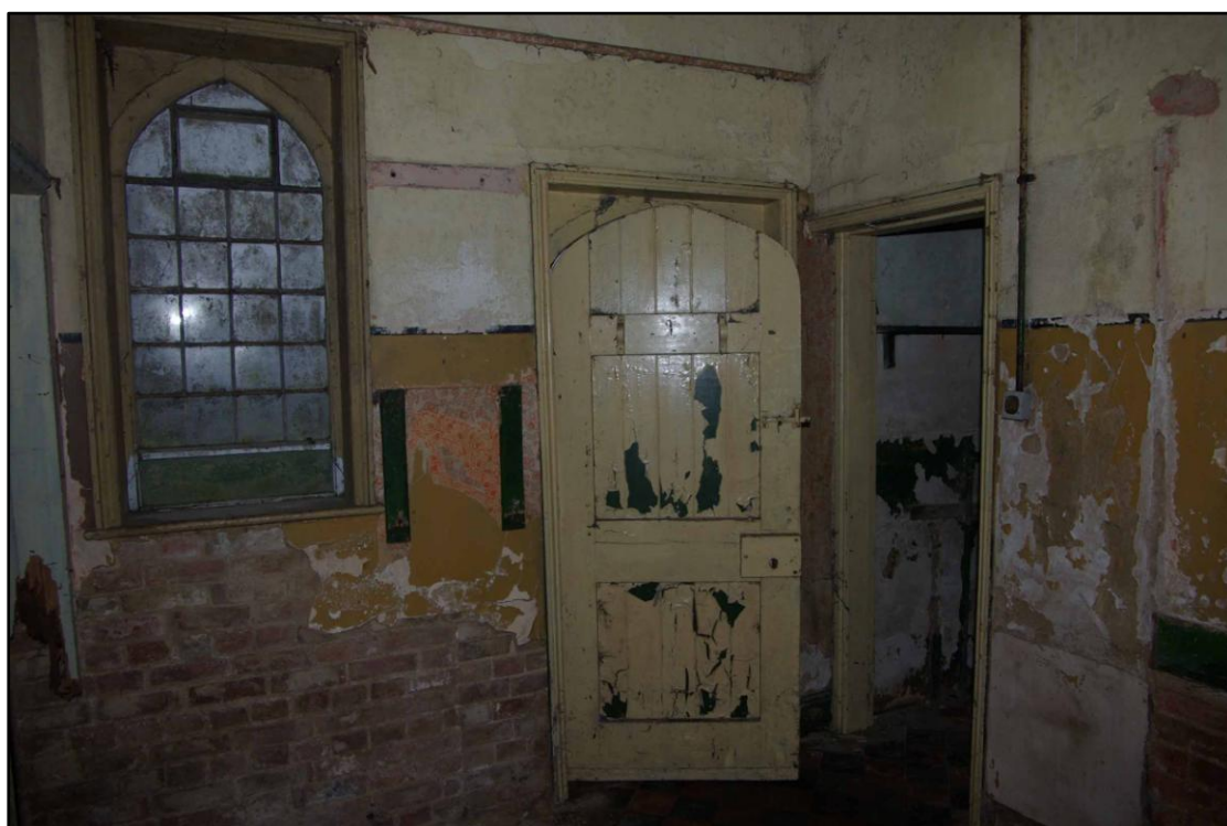
Figure 12. Room three and front door. Looking north-east.
