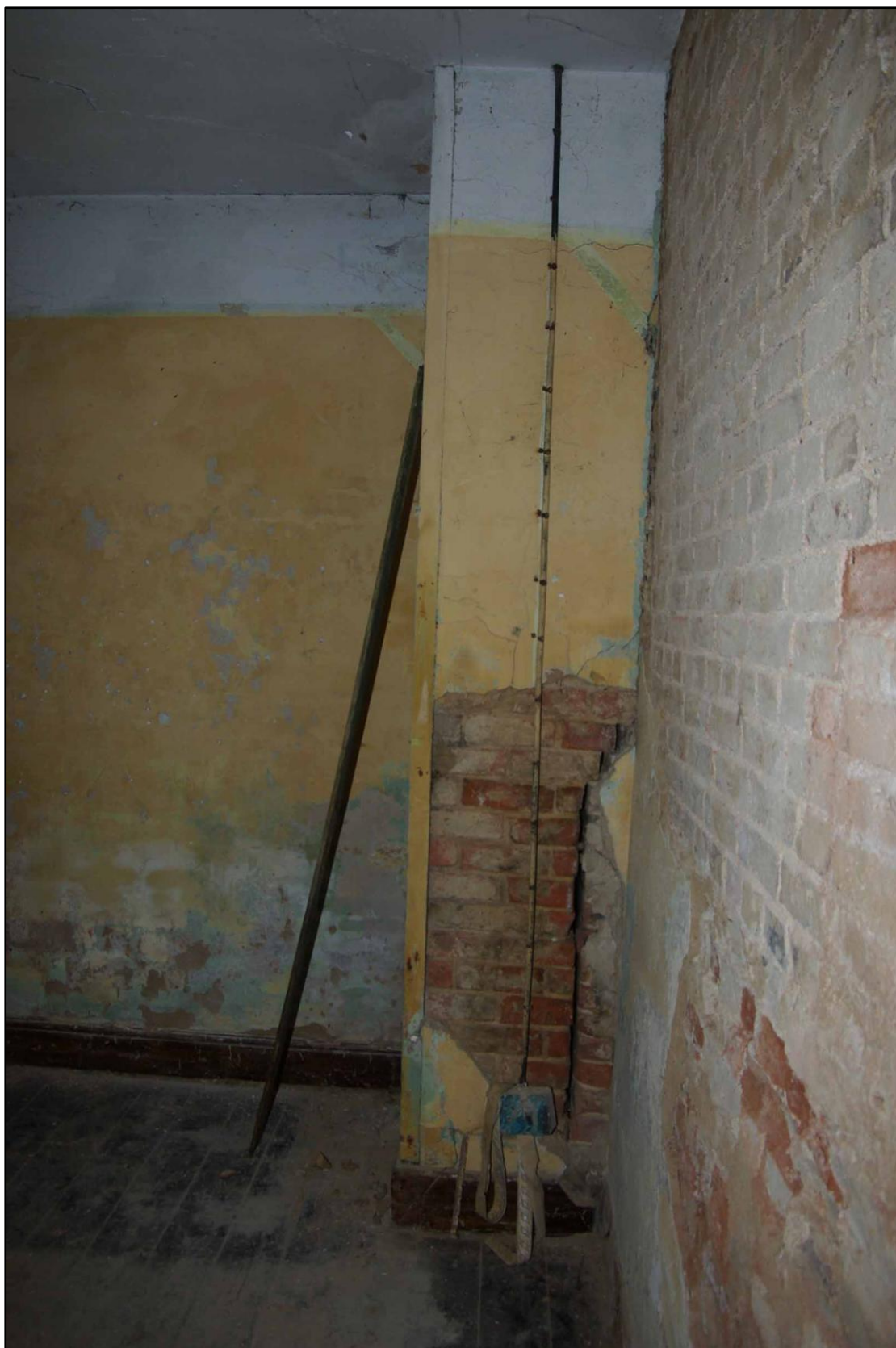
Figure 18. Room six. Straight line joint at chimney. Looking east.
