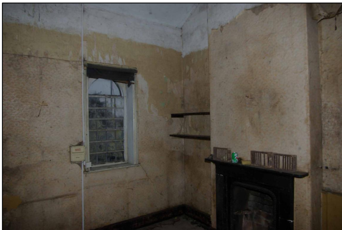
Figure 9. Room one. Looking north-east.
