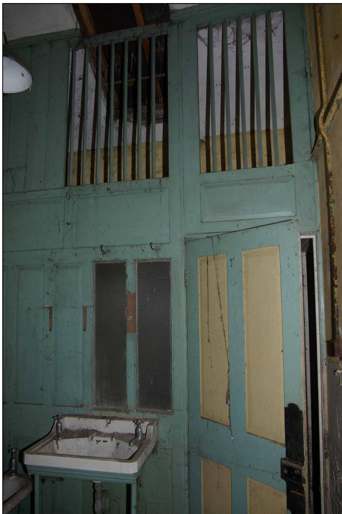
Figure 16. Room five bathroom partition. Facing north.
