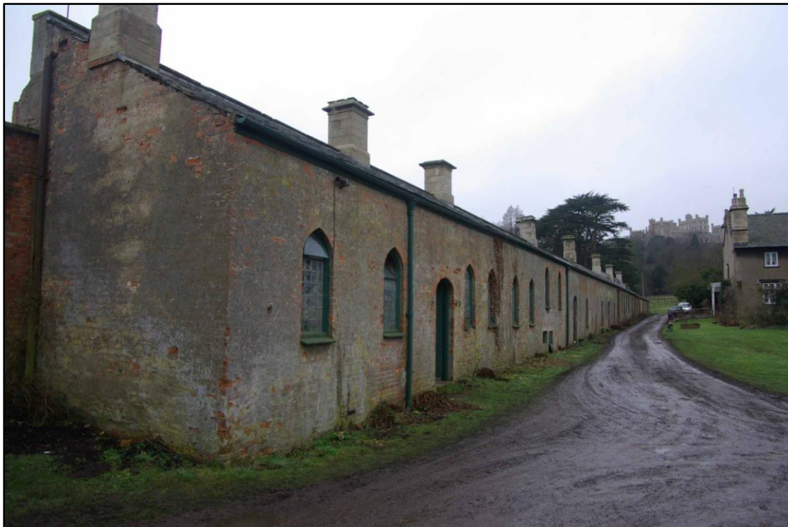
Figure 4. Bothy range looking west.
