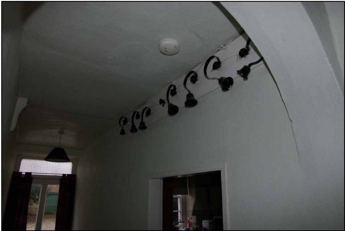
Figure 15 Servant bells in rear corridor Looking north west
