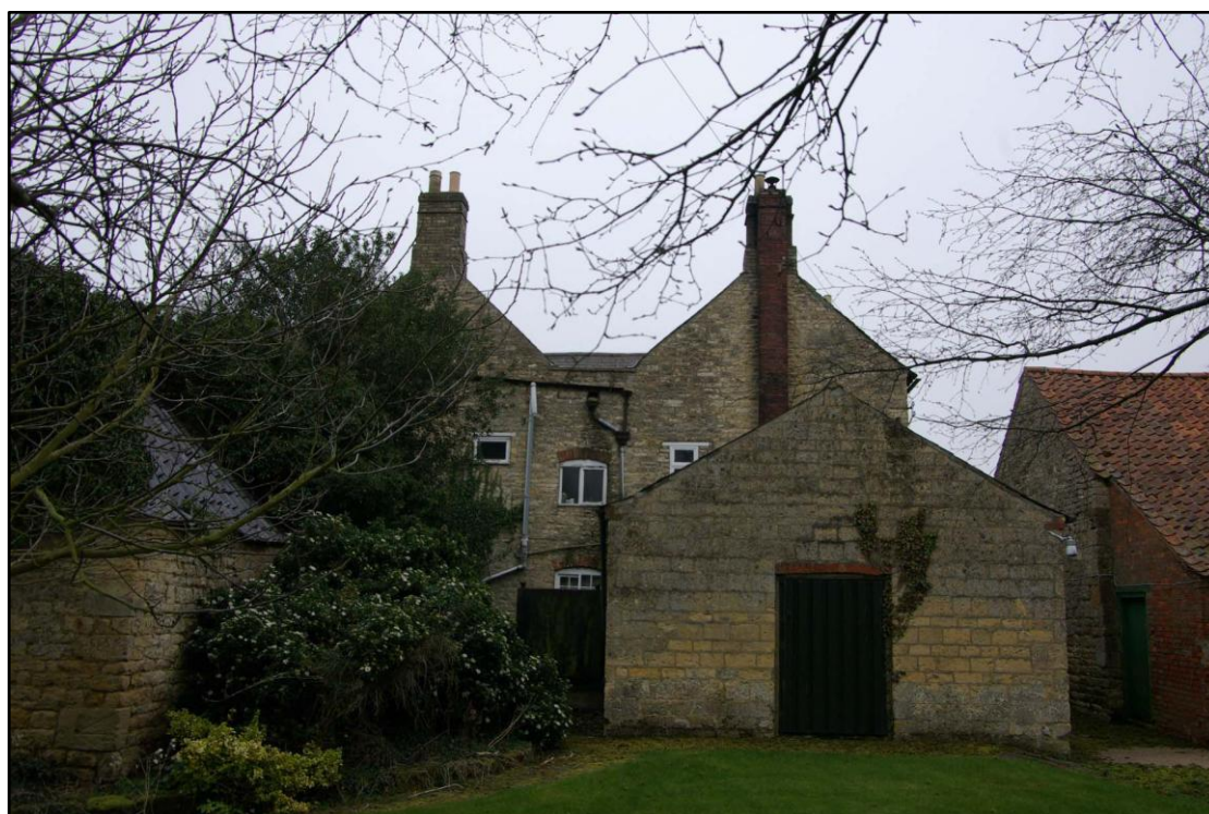
Figure 11 Bescaby House north west facing elevation and extension
