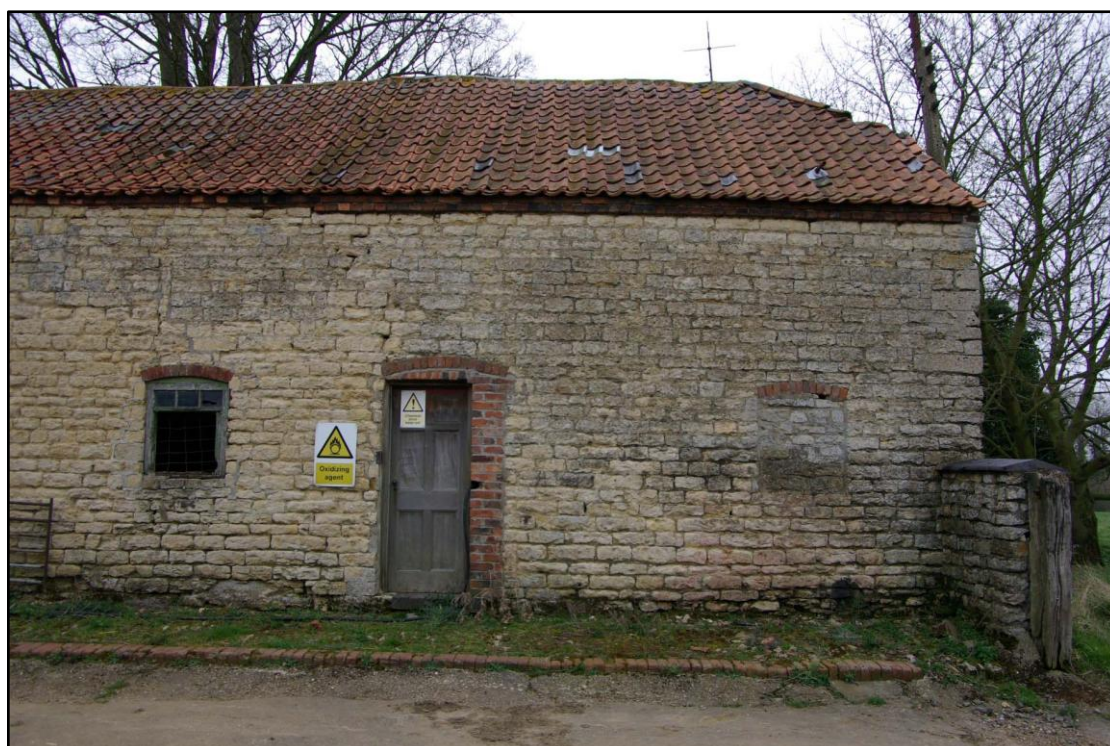
Figure 58 North west to south east stables, southern end Looking north east
