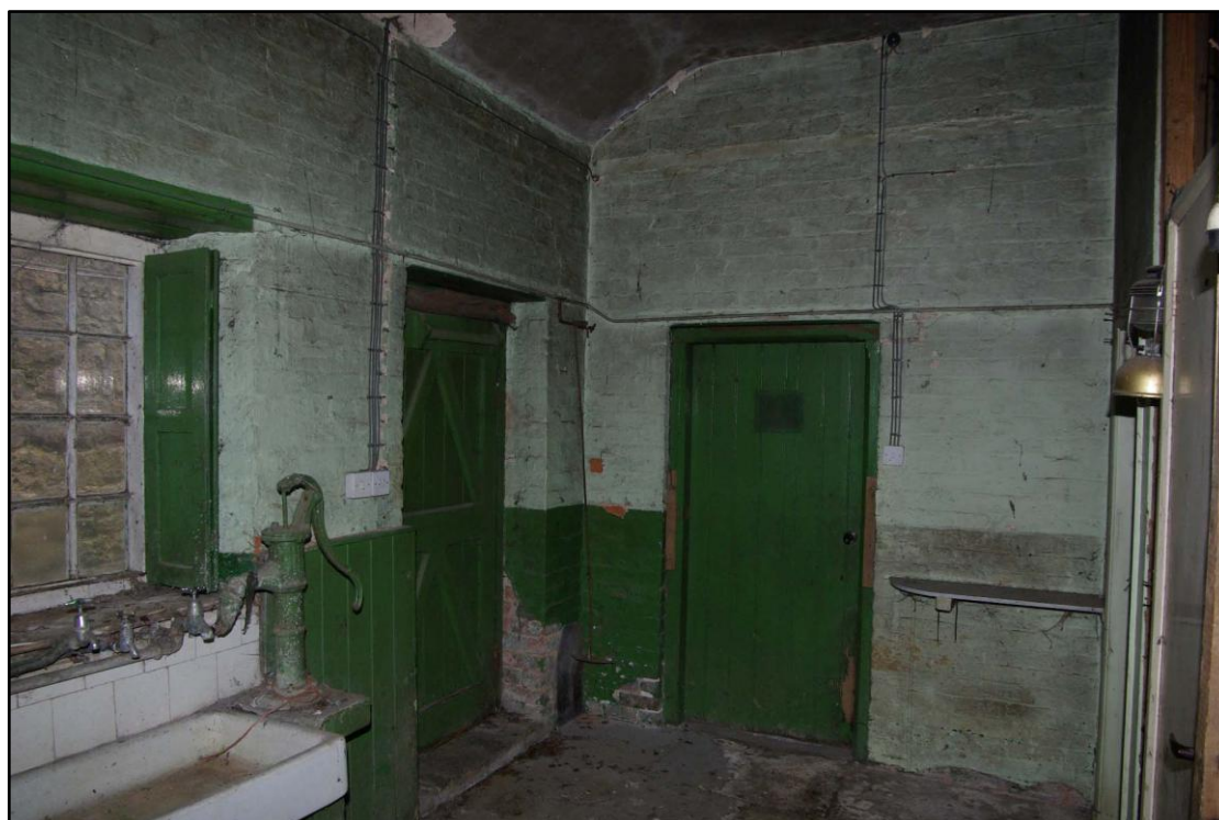
Figure 33 Rear extension, north end room Looking north west
