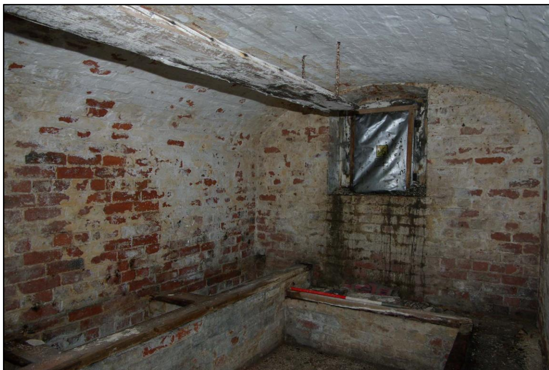
Figure 28 Cellar, north eastern room Looking north. 1m scale
