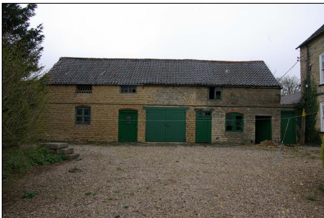
Figure 47 Stables, south east elevation Looking north west
