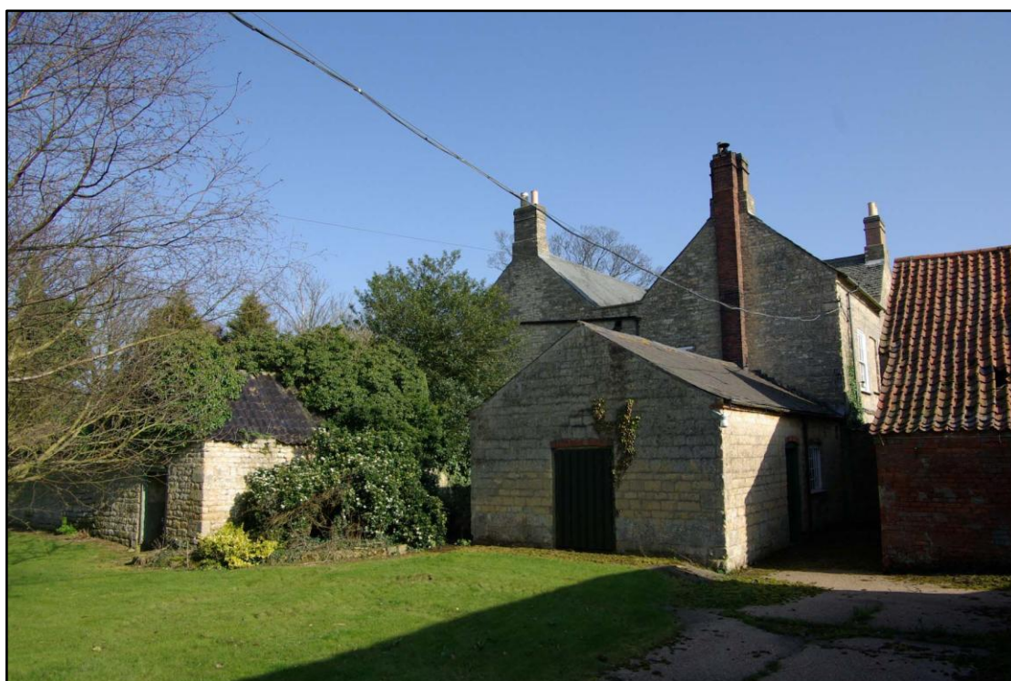
Figure 74 Outside toilet (building on left), servant's side Looking east
