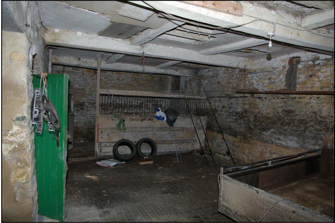
Figure 51 Stables, western room Looking west
