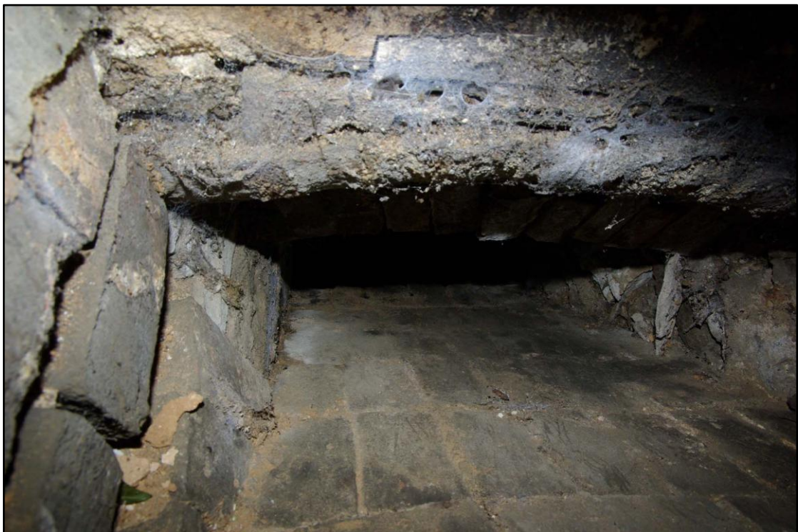
Figure 76 Chute from servant's toilet Looking south west
