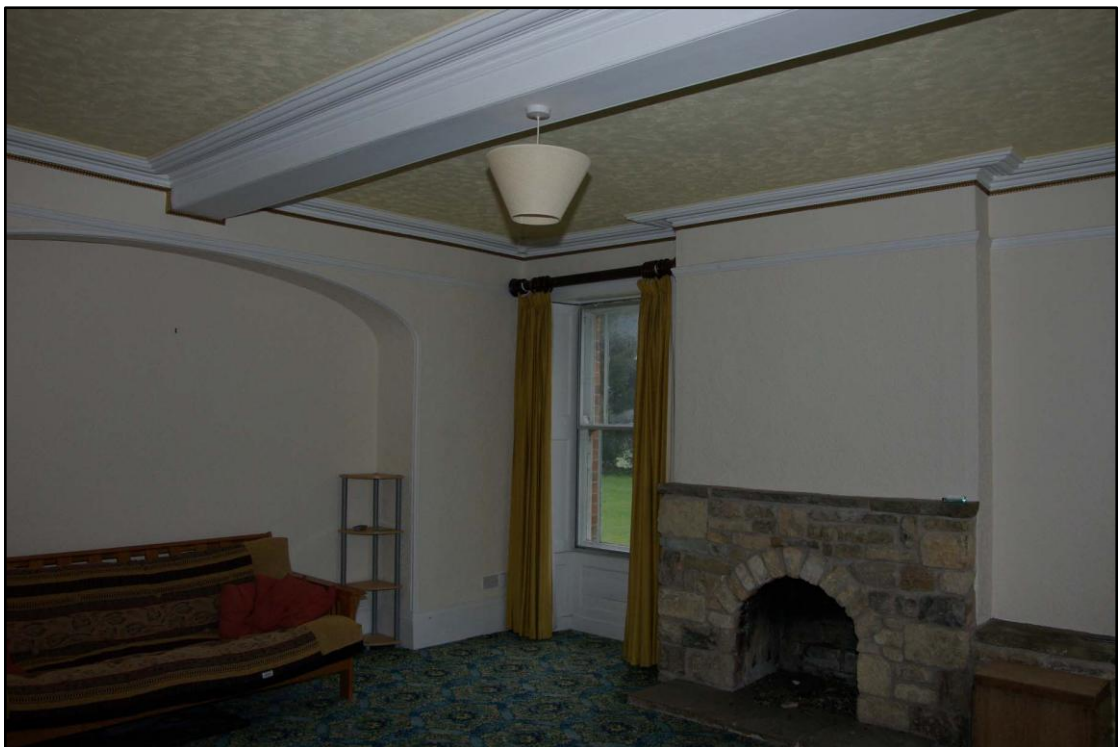
Figure 21 Front, eastern room Looking north
