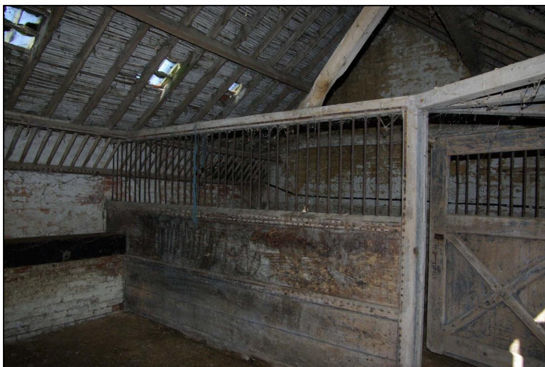
Figure 53 Stables, western brick extension Looking north
