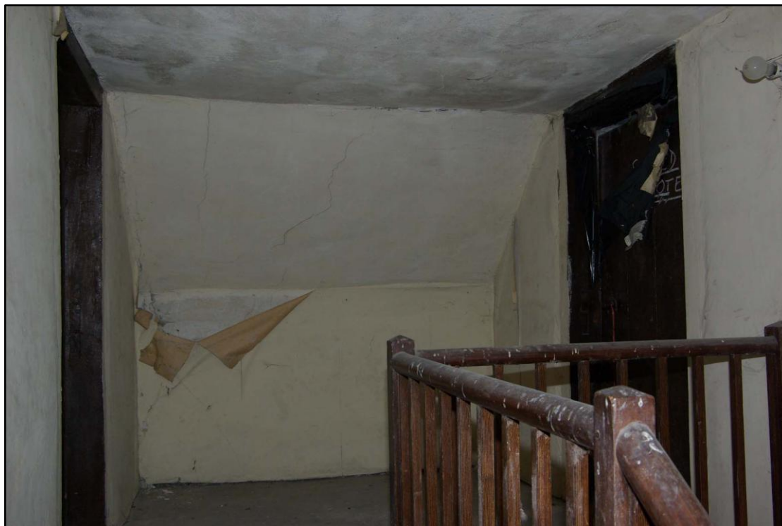
Figure 43 Top floor servant's landing Facing north
