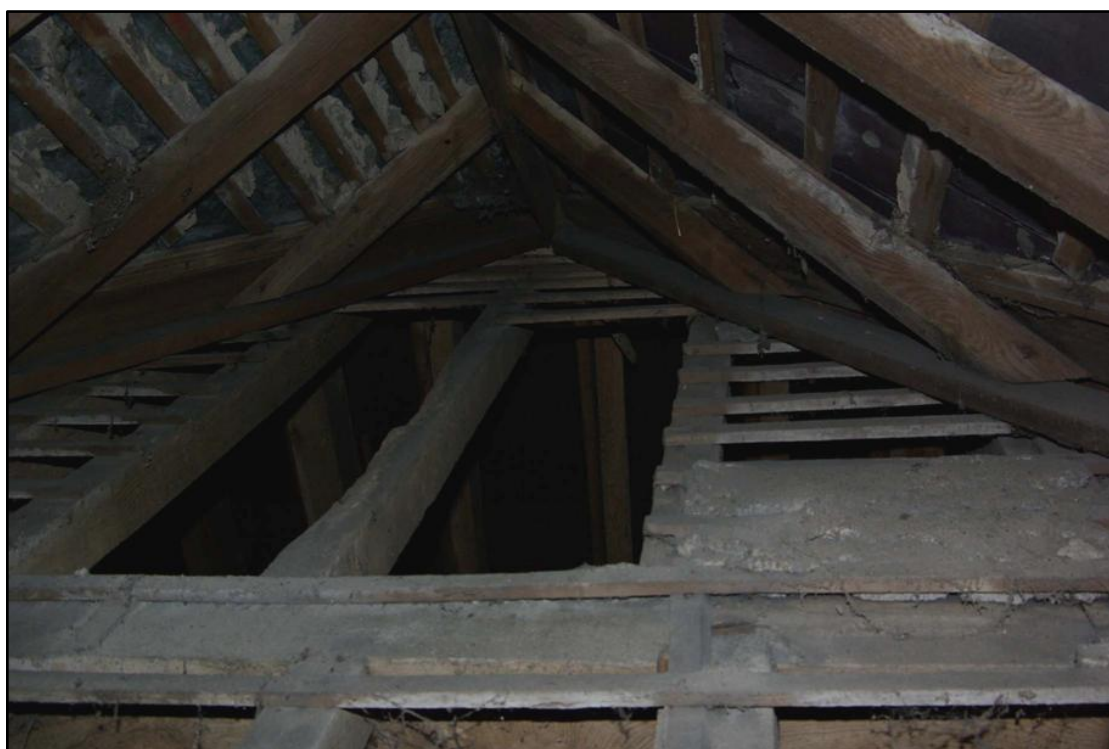
Figure 46 Junction of house roof and eastern rear gable Looking south east
