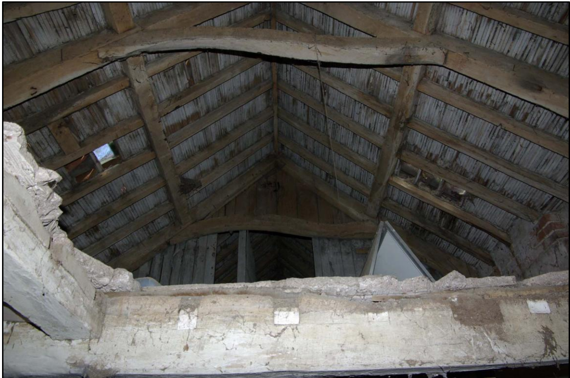
Figure 52 Stables roof structure Looking north east
