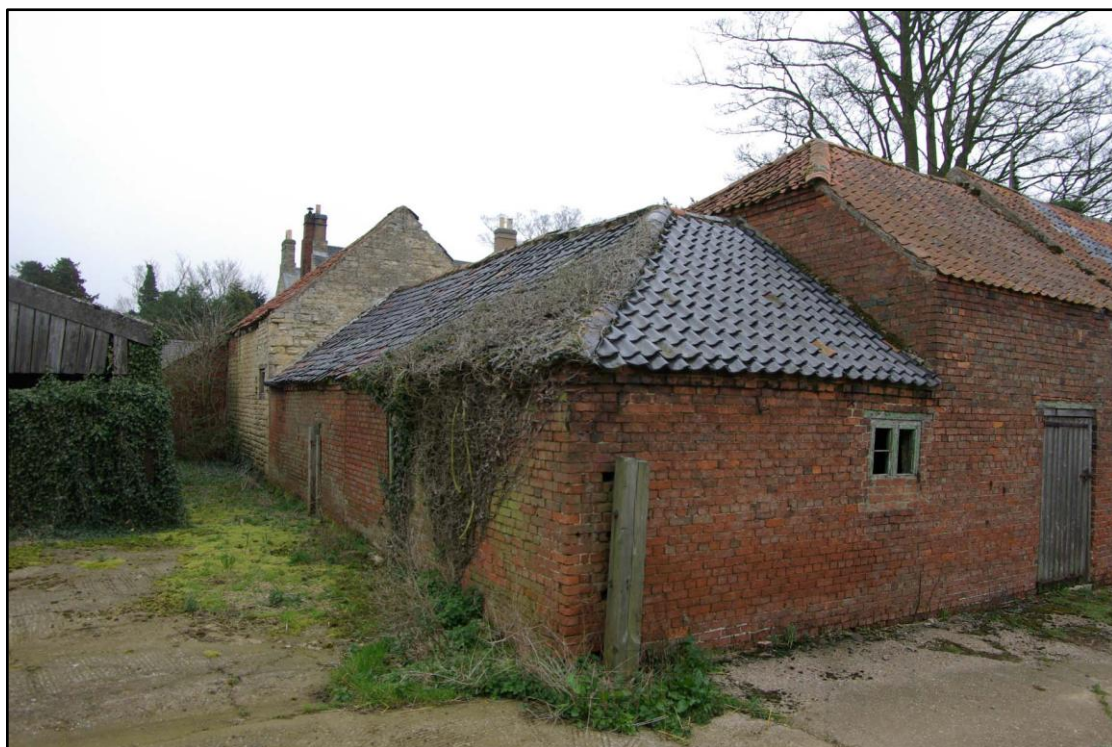
Figure 56 Rear of western extension to stables Looking east
