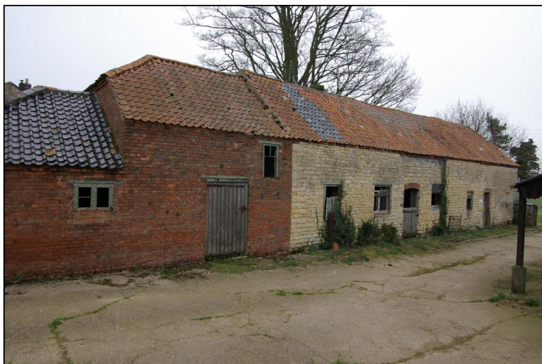
Figure 57 North west to south east stables, south west elevation Looking east
