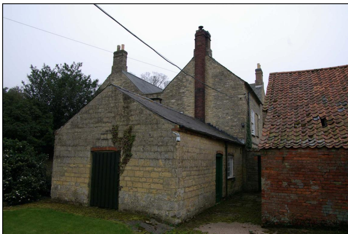
Figure 12 Bescaby House north western extension
