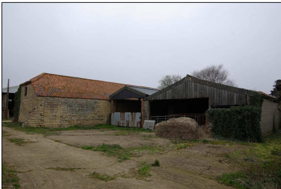
Figure 68 Modern barns between stables and cart shed Looking north
