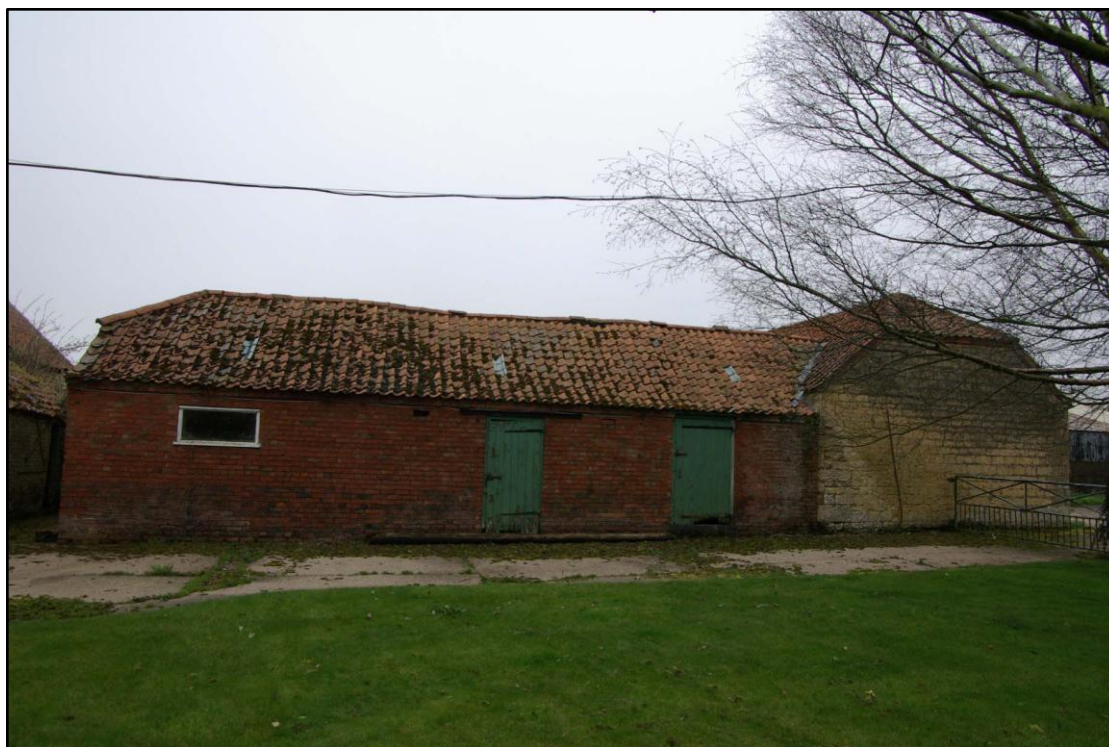
Figure 71 Outbuildings to south east of cart shed Looking east
