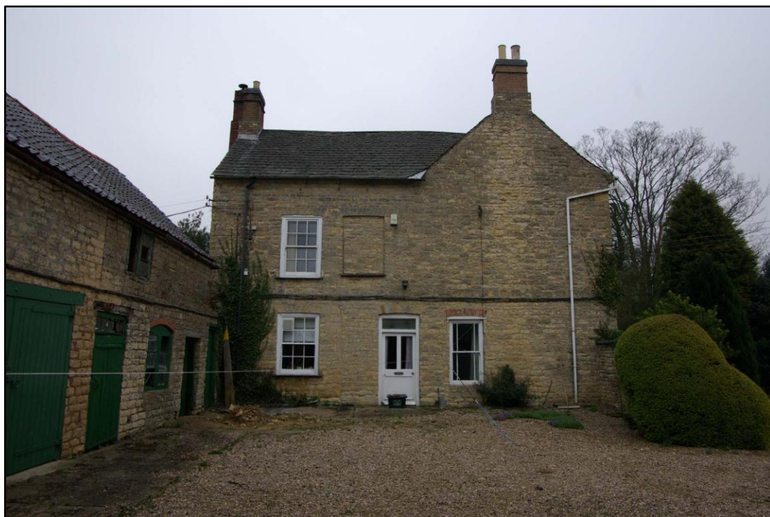
Figure 9 Bescaby House south west facing elevation
