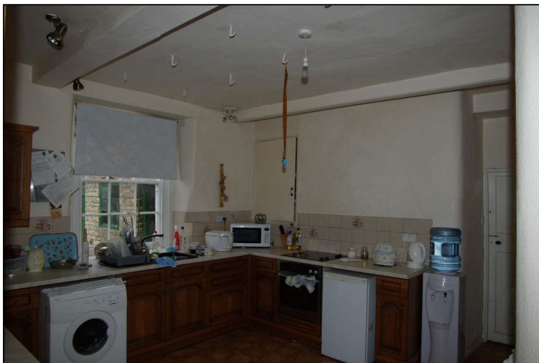
Figure 29 Kitchen Facing west. Note chamfer by window
