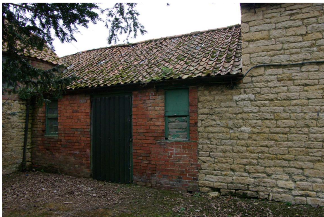
Figure 48 Brick extension to stables Looking west
