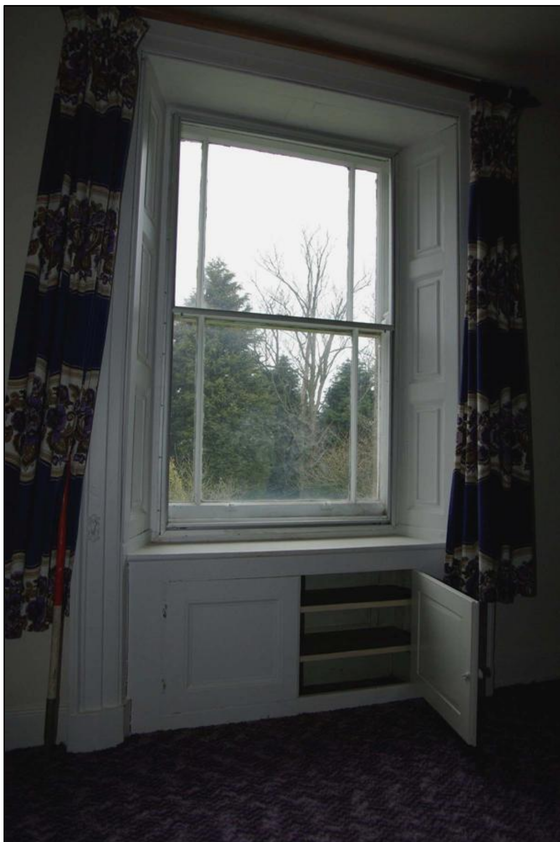
Figure 38 Rear, eastern bedroom. Window cupboards Looking east
