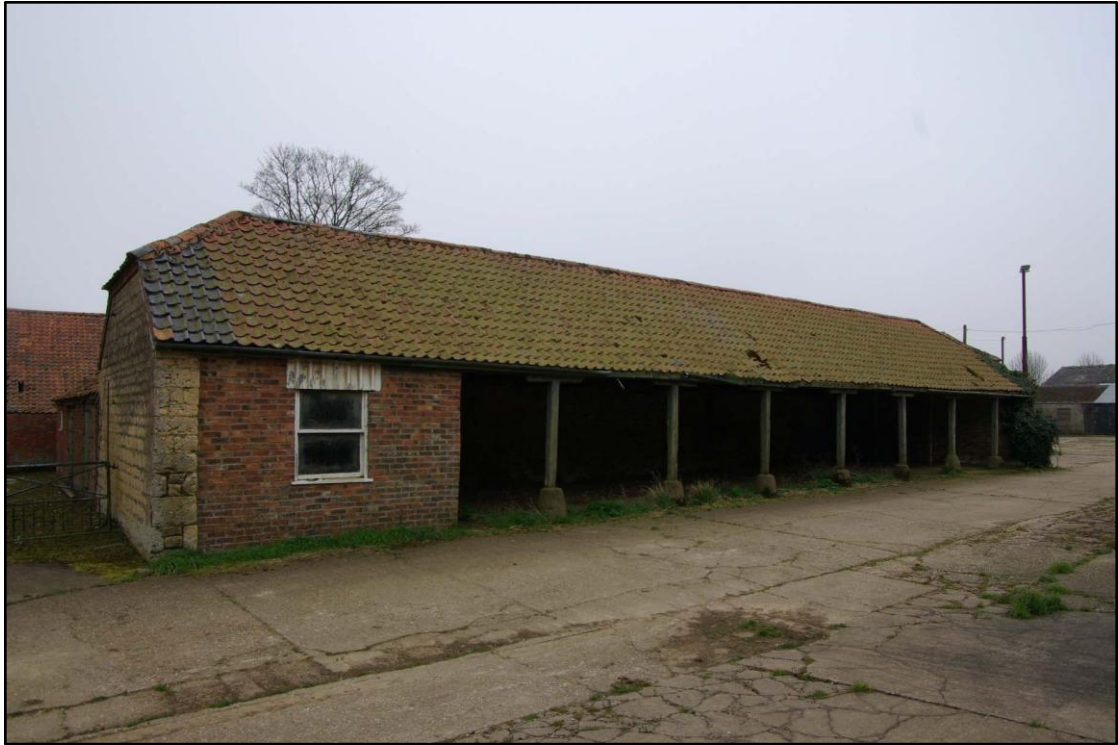
Figure 69 Cart shed, north west elevation Looking south
