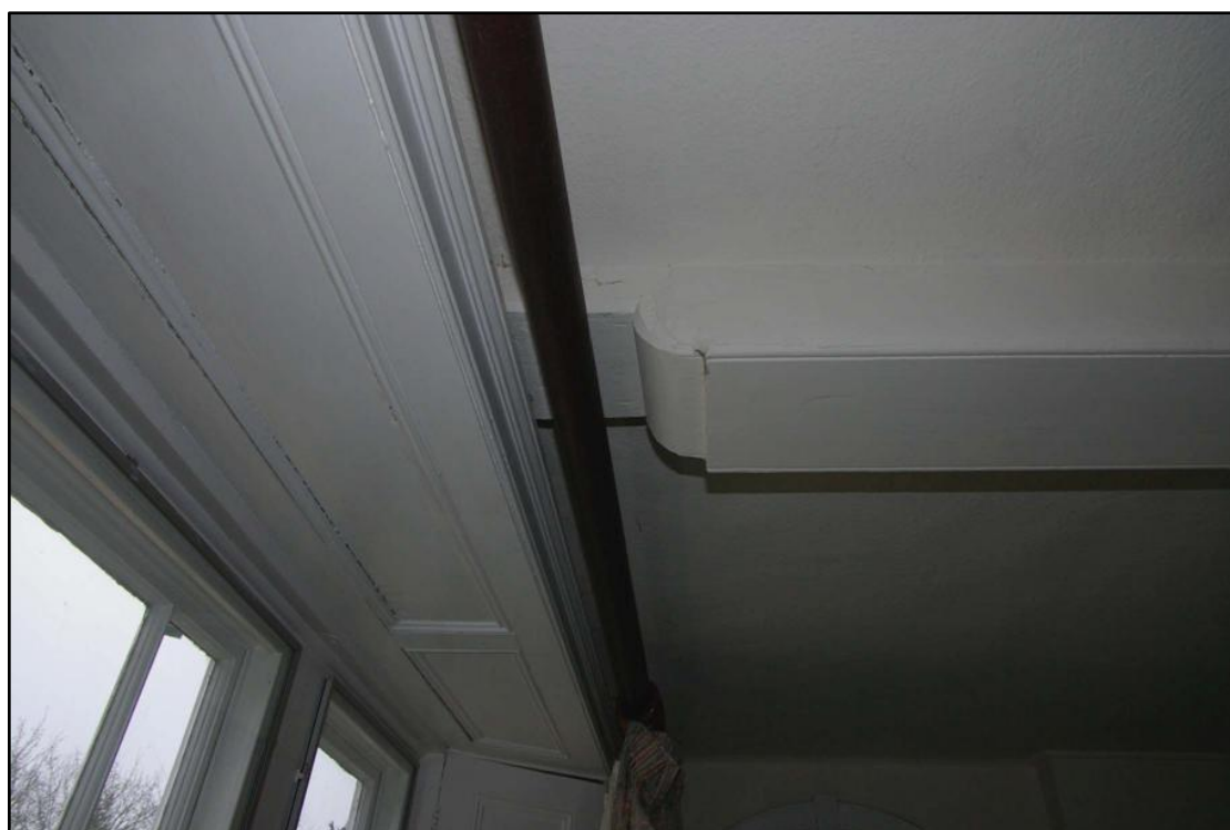
Figure 18 South end of ceiling beam in front, western room Looking west
