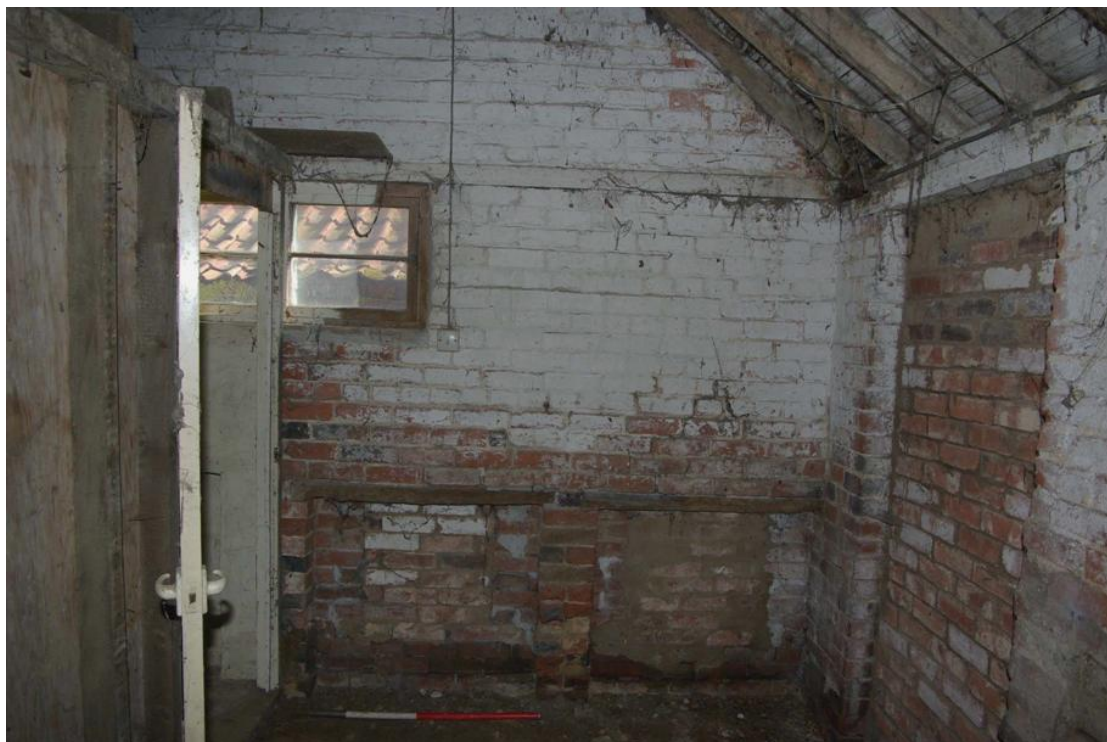
Figure 73 Outbuildings, southern room Looking south east. 1m scale
