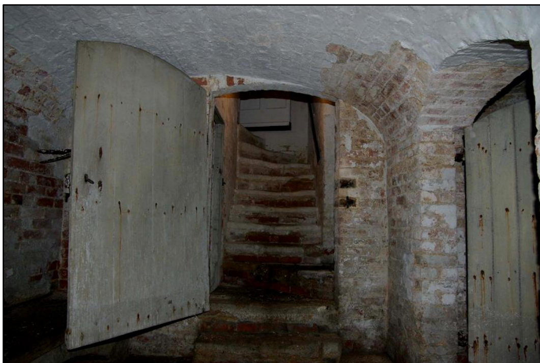
Figure 24 Cellar steps Looking south west
