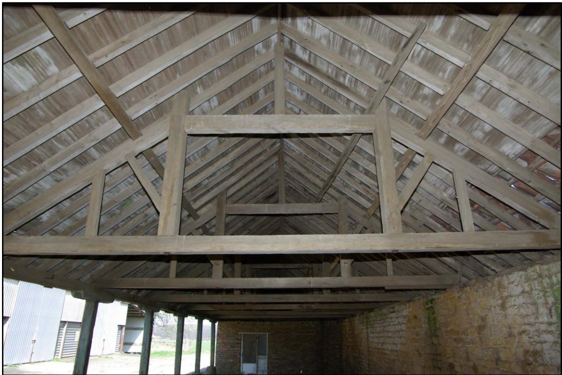
Figure 70 Cart shed roof structure Looking north east
