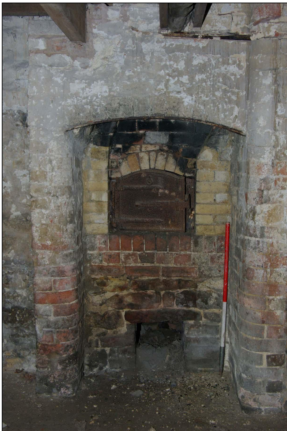
Figure 50 Stables, bread oven Looking north west. 1m scale
