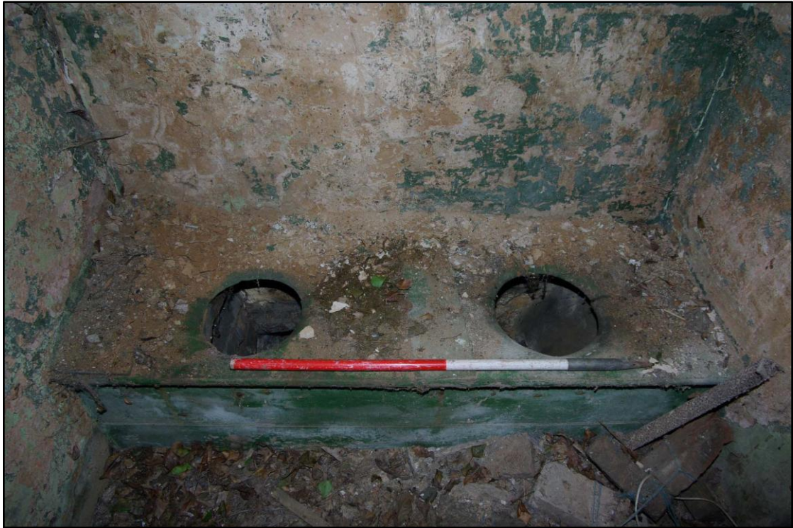
Figure 75 Outside toilet, servants side Looking south west. 1m scale
