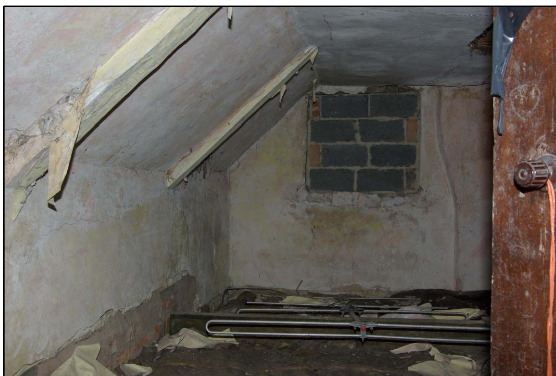
Figure 44 Top floor servant's accommodation, front west room Looking south west
