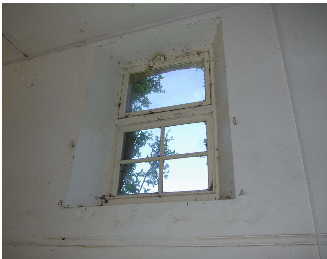
Figure 20 Ground floor window detail and plaster bead beneath
