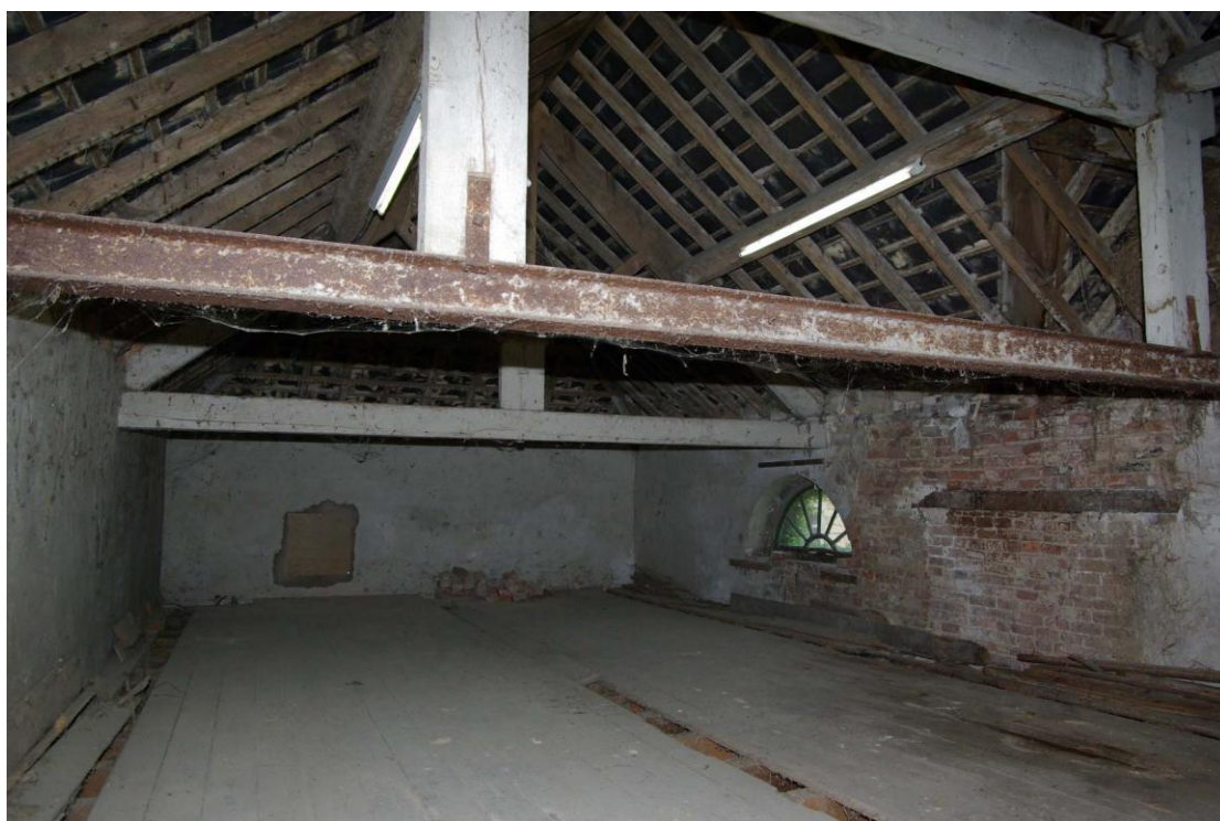
Figure 24 First floor, western room Facing west
