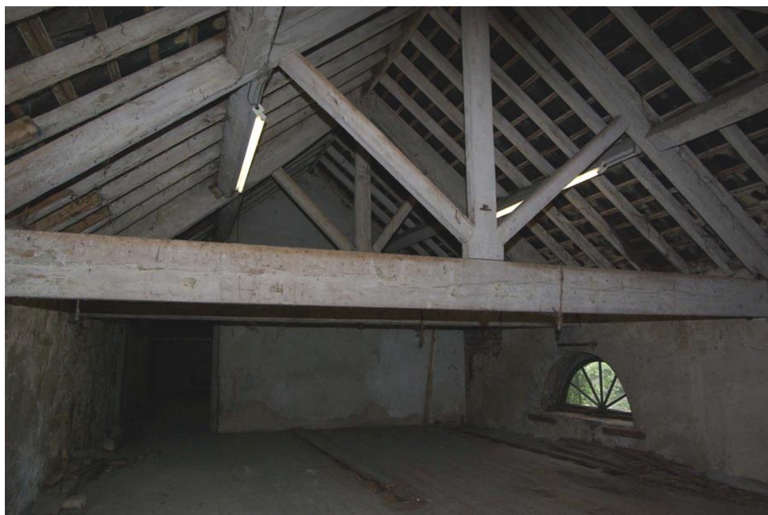
Figure 22 First floor, eastern room Facing west
