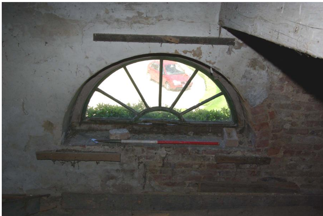
Figure 28 First floor, western room semicircular window 1m scale
