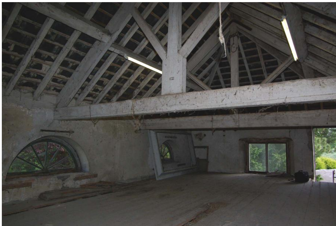
Figure 23 First floor, eastern room Facing north-east
