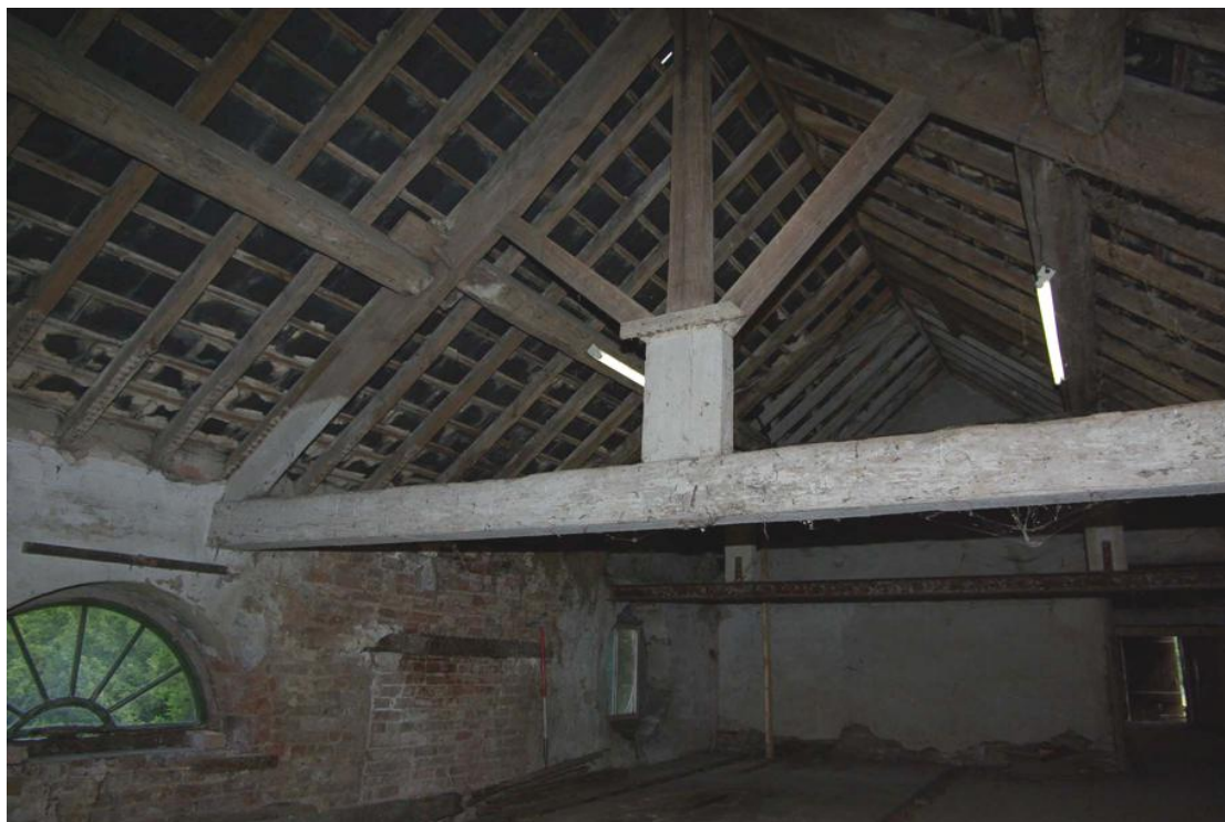
Figure 25 First floor, western room Facing north-east
