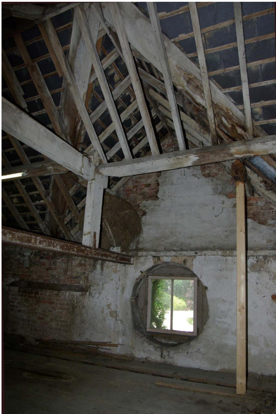
Figure 27 Gable and roof detail Facing north-west
