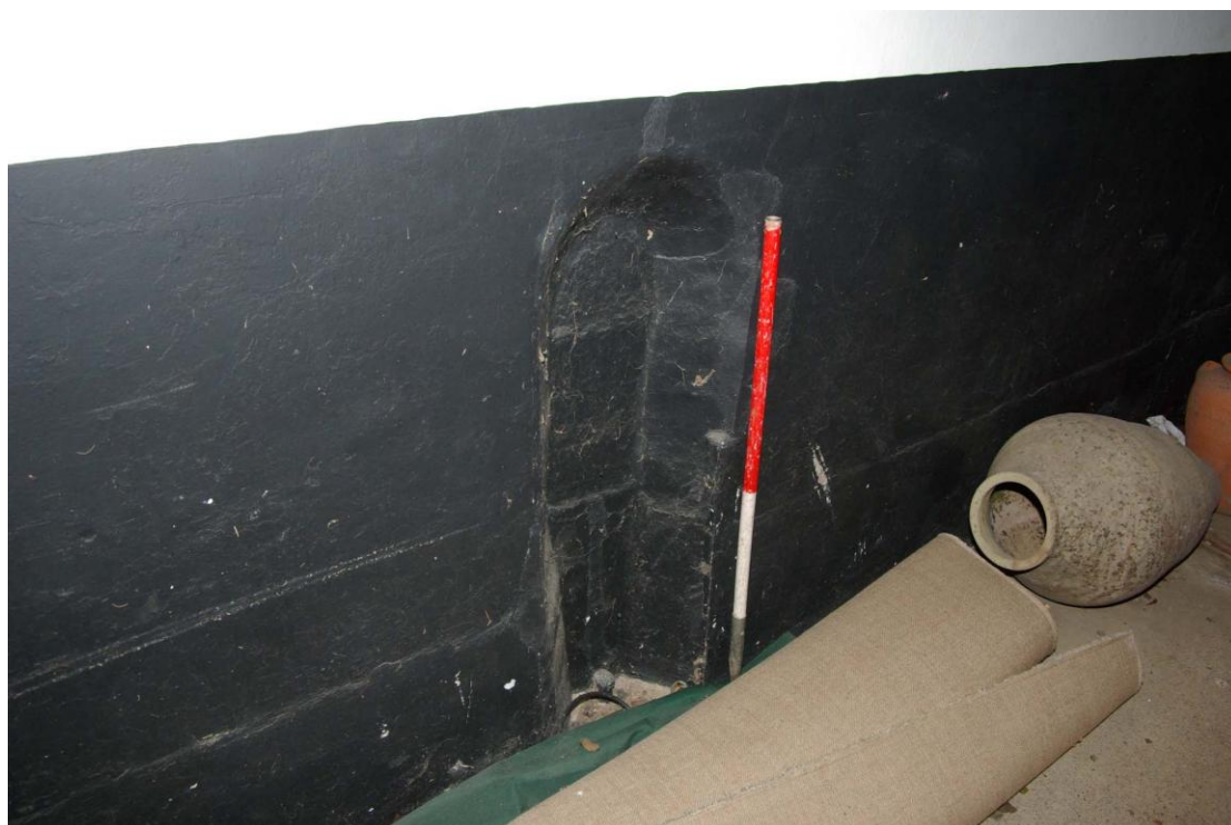
Figure 21 Recess in south-eastern wall 1m scale
