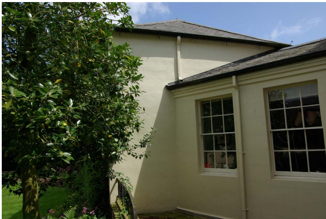
Figure 7 Boot room joining the pavilion to the hall
