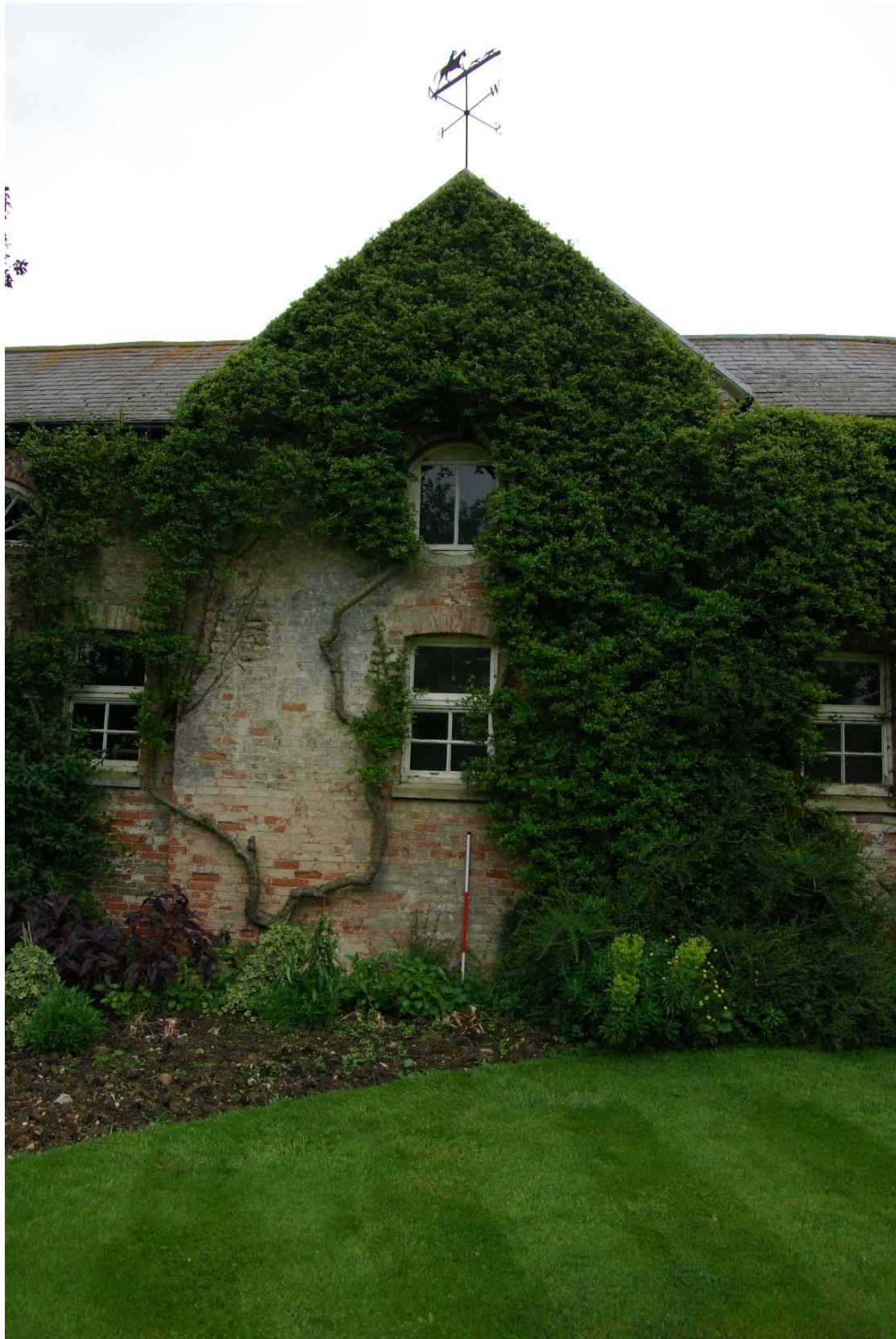
Figure 10 North-west elevation gable 1.5m scale
