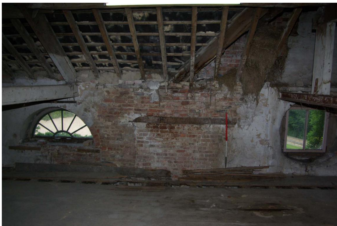
Figure 31 Blocked opening behind gable 1m scale
