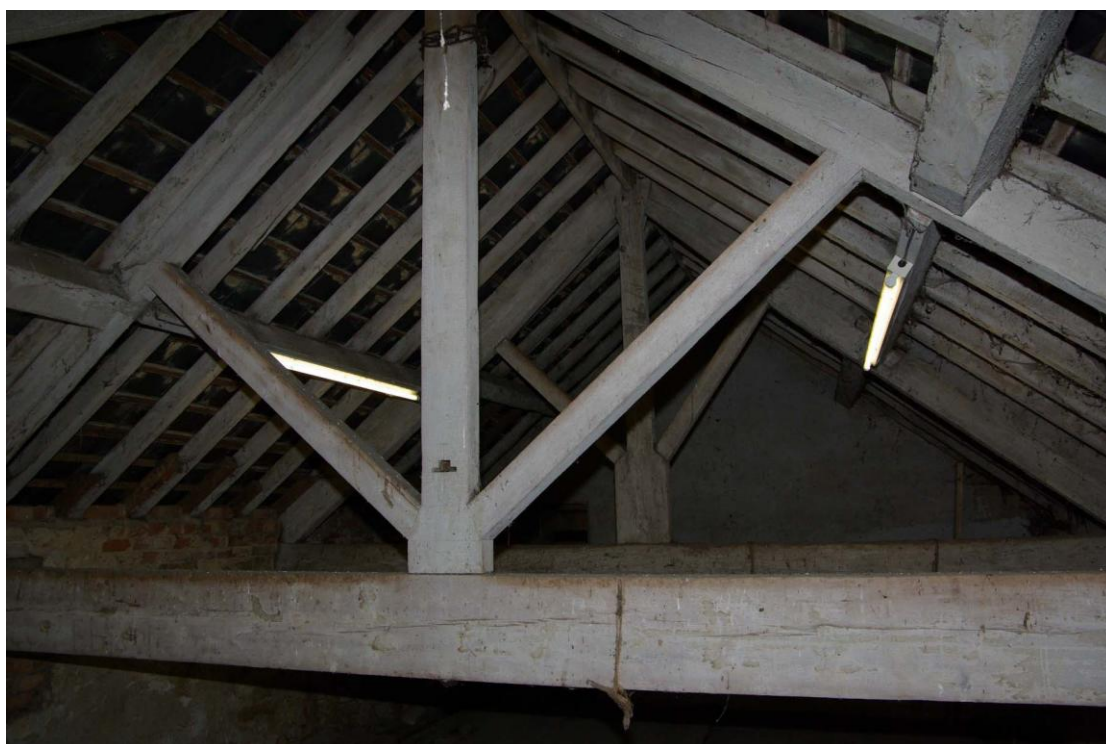
Figure 26 First floor roof details Western room, facing south-west
