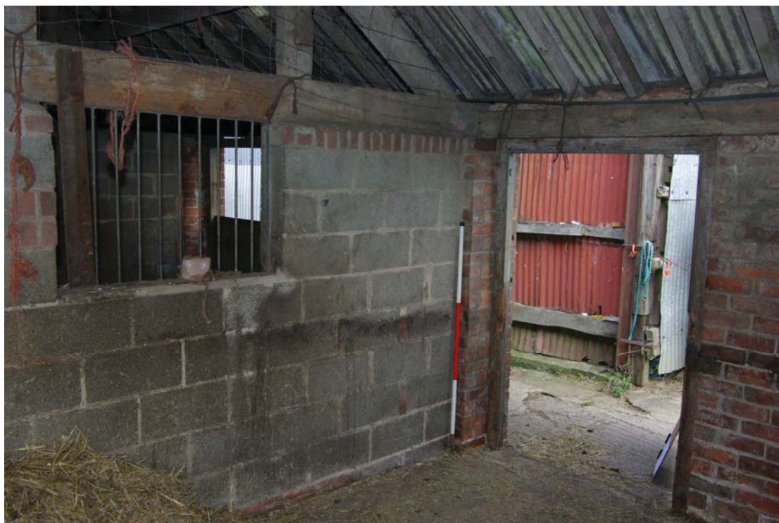
Figure 38 Barn B eastern bay Looking north. 1.5m scale.
