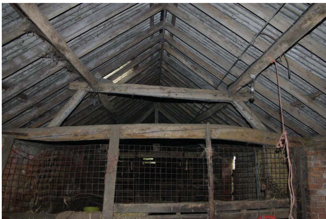
Figure 23 Barn A western bay roof structure Looking south-east.
