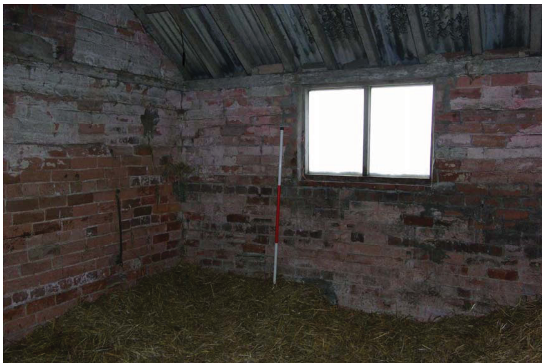
Figure 40 Barn B east end room Looking south. 1.5m scale.
