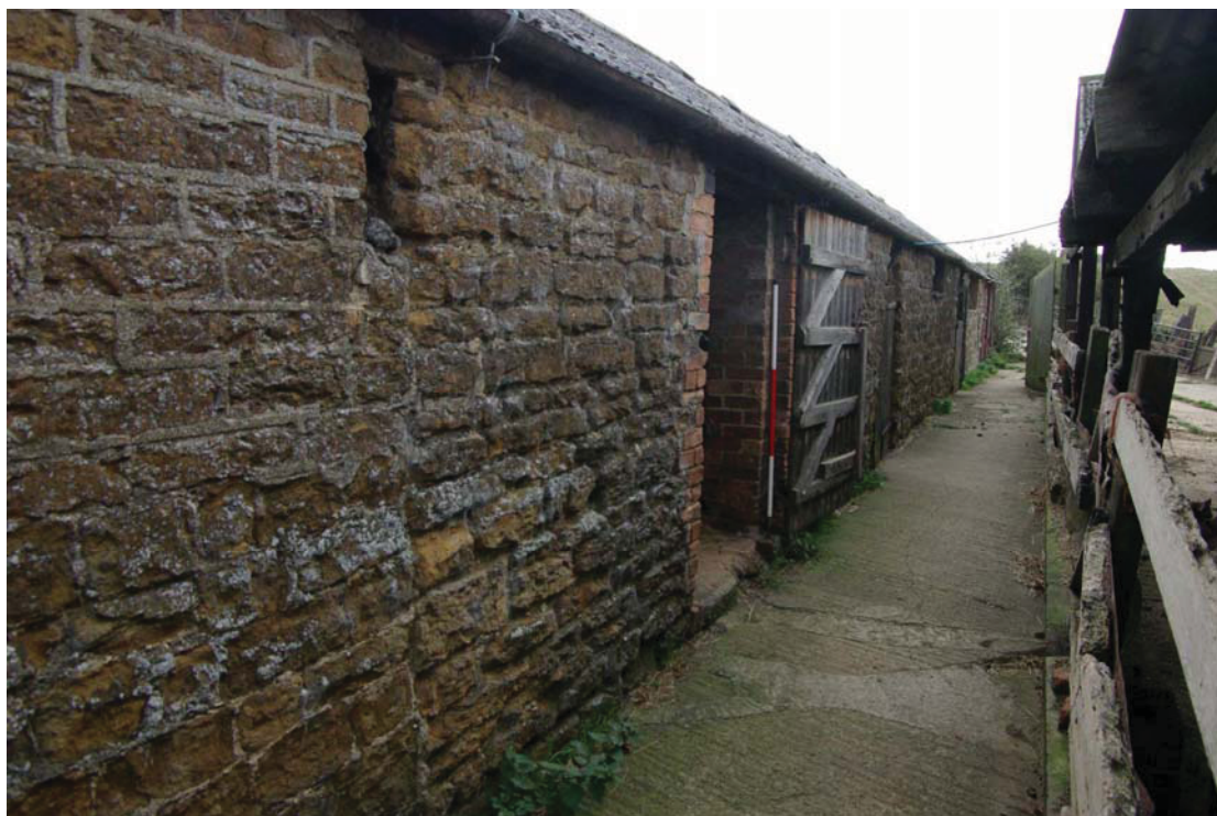
Figure 14 Barn A. Straight line joint Looking east. 1.5m scale
