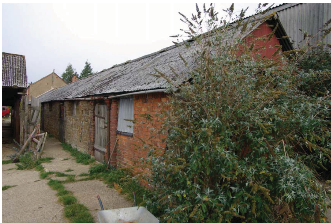
Figure 13 SW elevation of Barn A Looking north-west.
