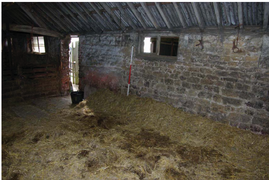
Figure 28 Barn A third bay Looking south. 1.5m scale.
