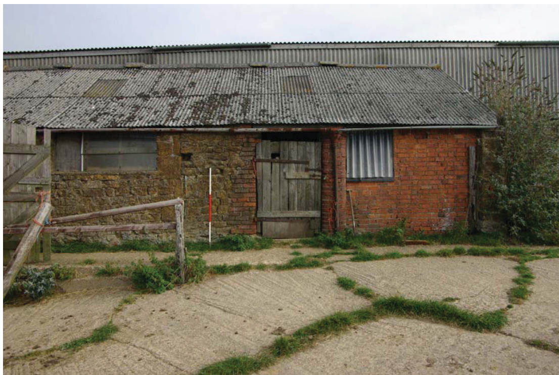
Figure 17 Barn A east end Looking north-east. 1.5m scale.
