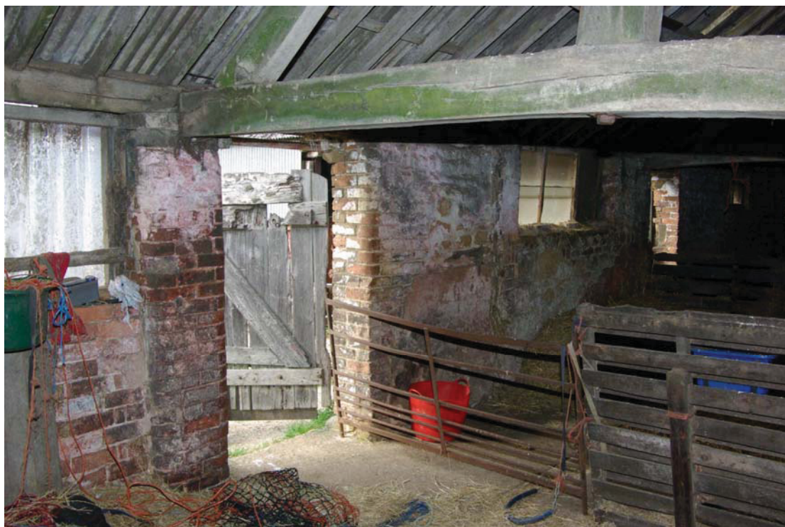
Figure 31 Barn A east end bay Looking west.
