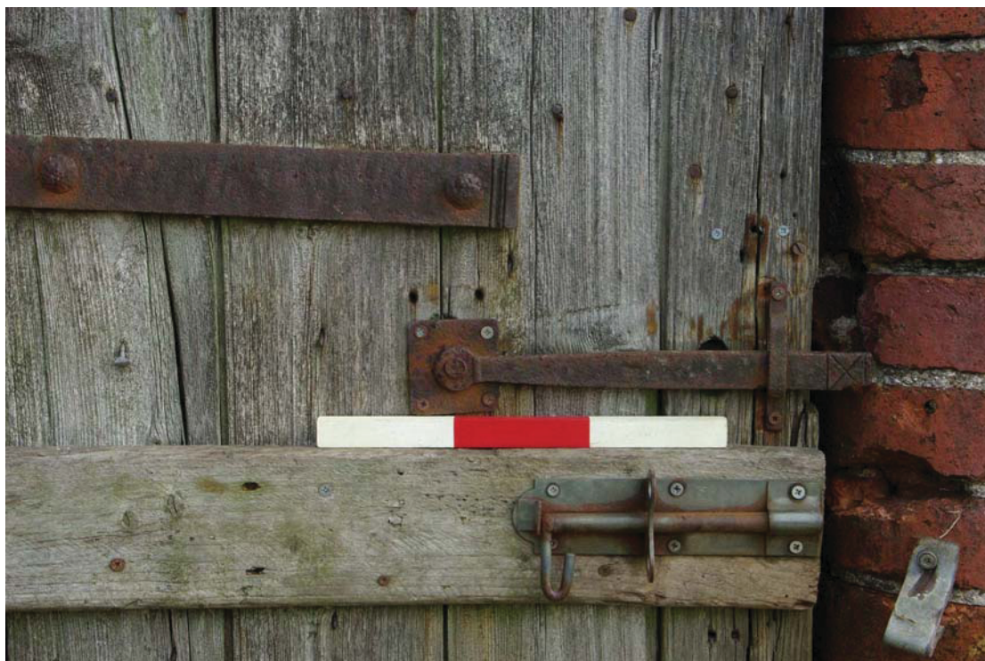
Figure 16 Barn A hinge and latch detail 0.3m scale.
