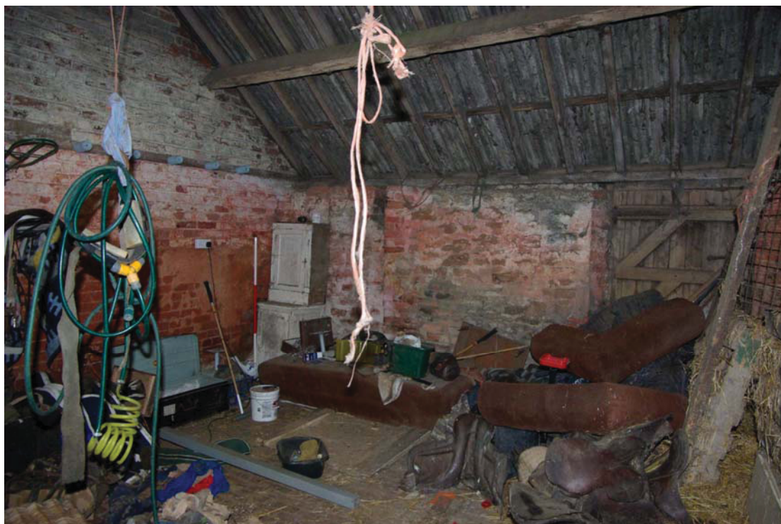
Figure 21 Barn A western end bay Looking north. 1.5m scale.
