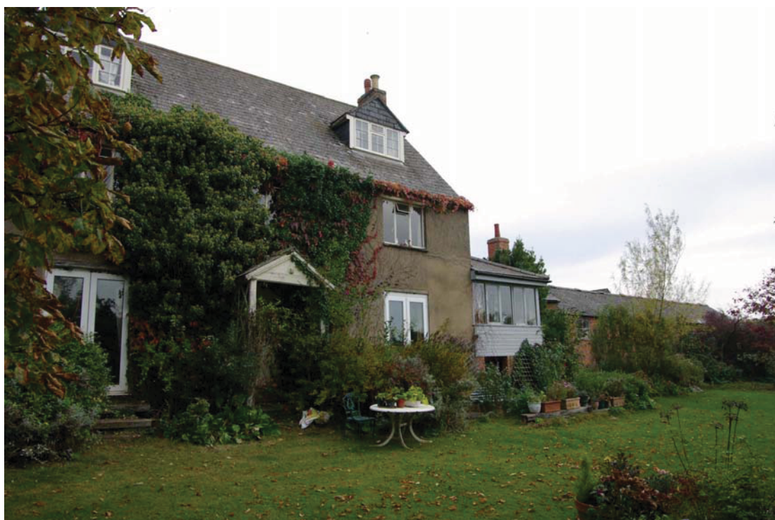
Figure 9 SW elevation of farmhouse and Barn B Looking east.
