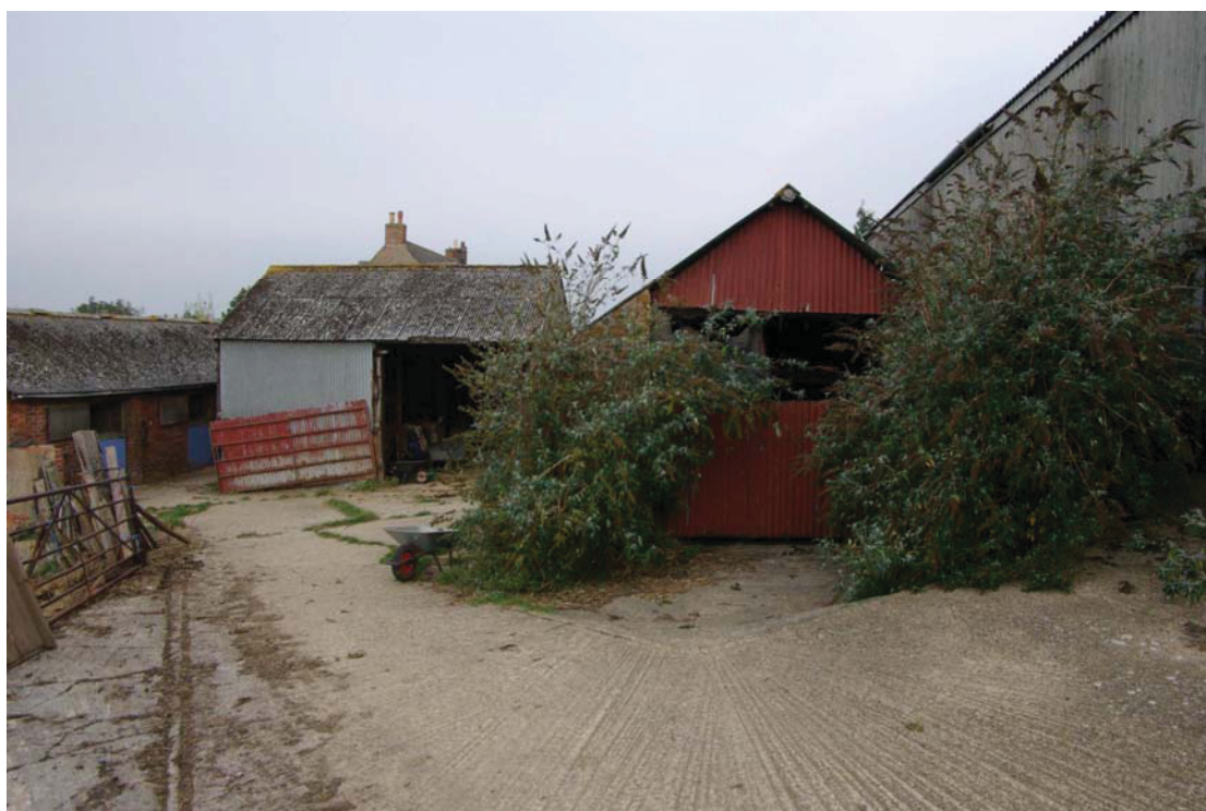
Figure 18 Barn A SE elevation Looking north-west. Barn B to left of picture.
