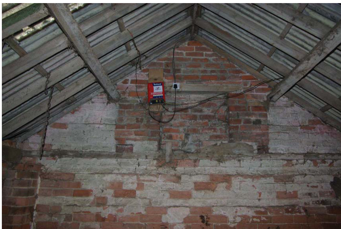
Figure 41 Barn B east end gable blocked window Looking south-east.
