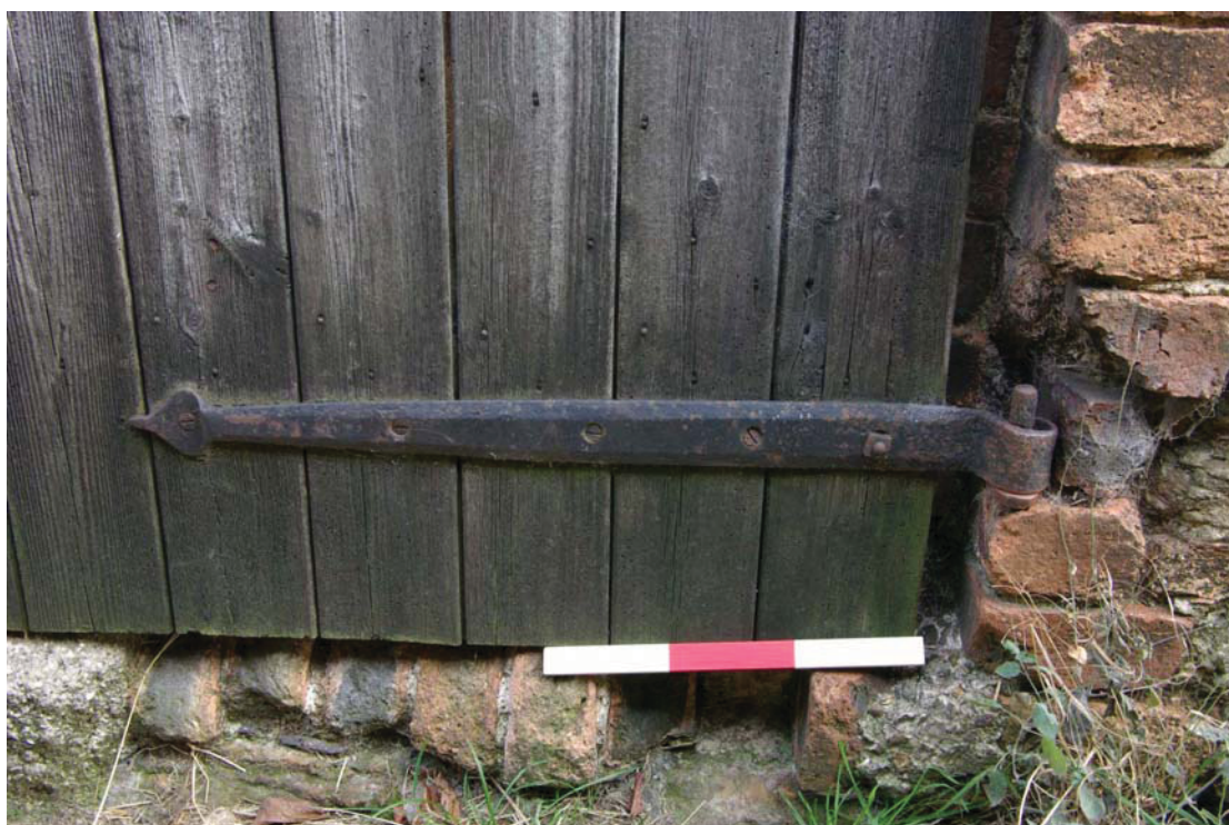
Figure 15 Barn A door hinge detail 0.3m scale.
