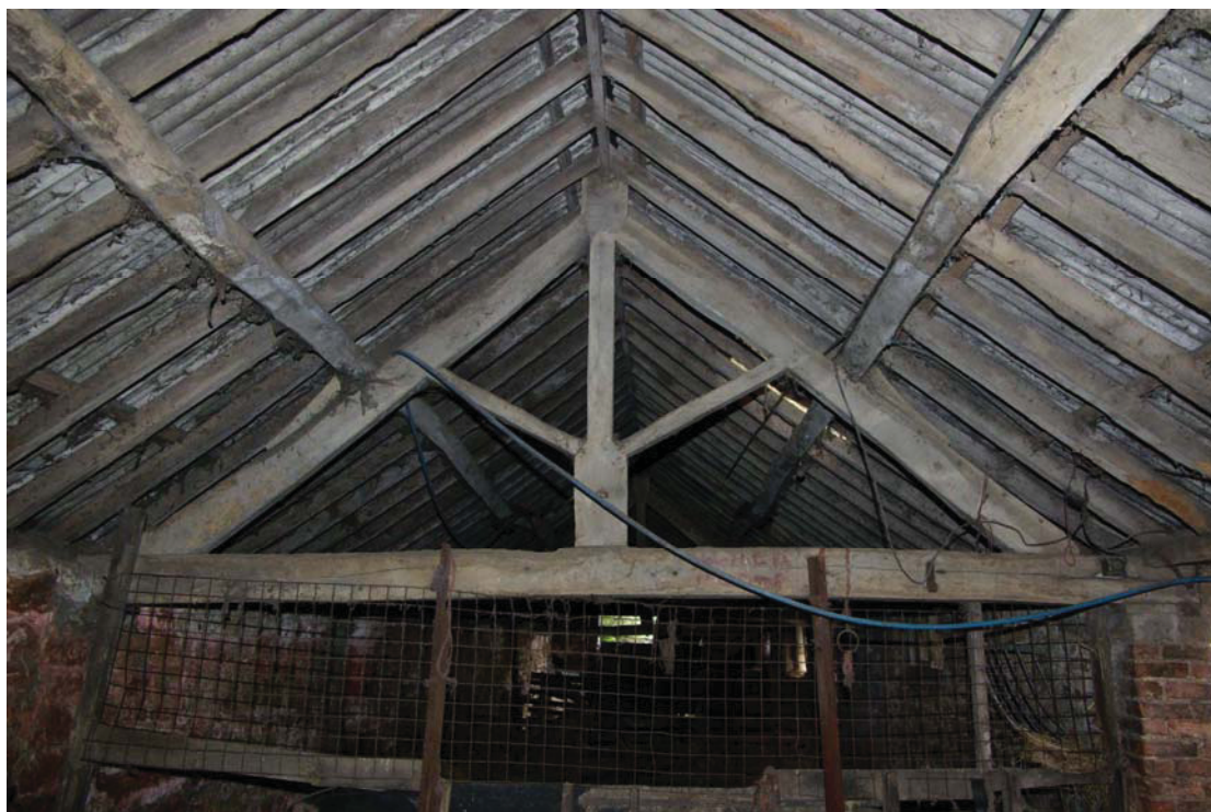
Figure 24 Barn A roof structure Looking south-east.
