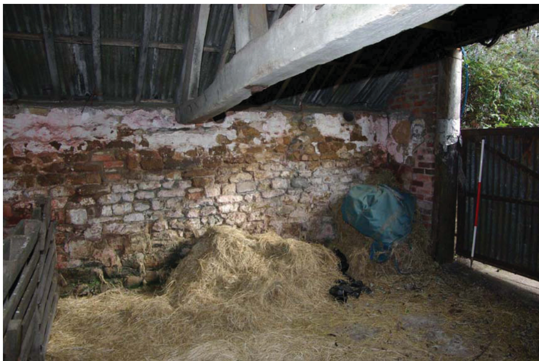
Figure 30 Barn A east end bay Looking north-east. 1.5m scale.
