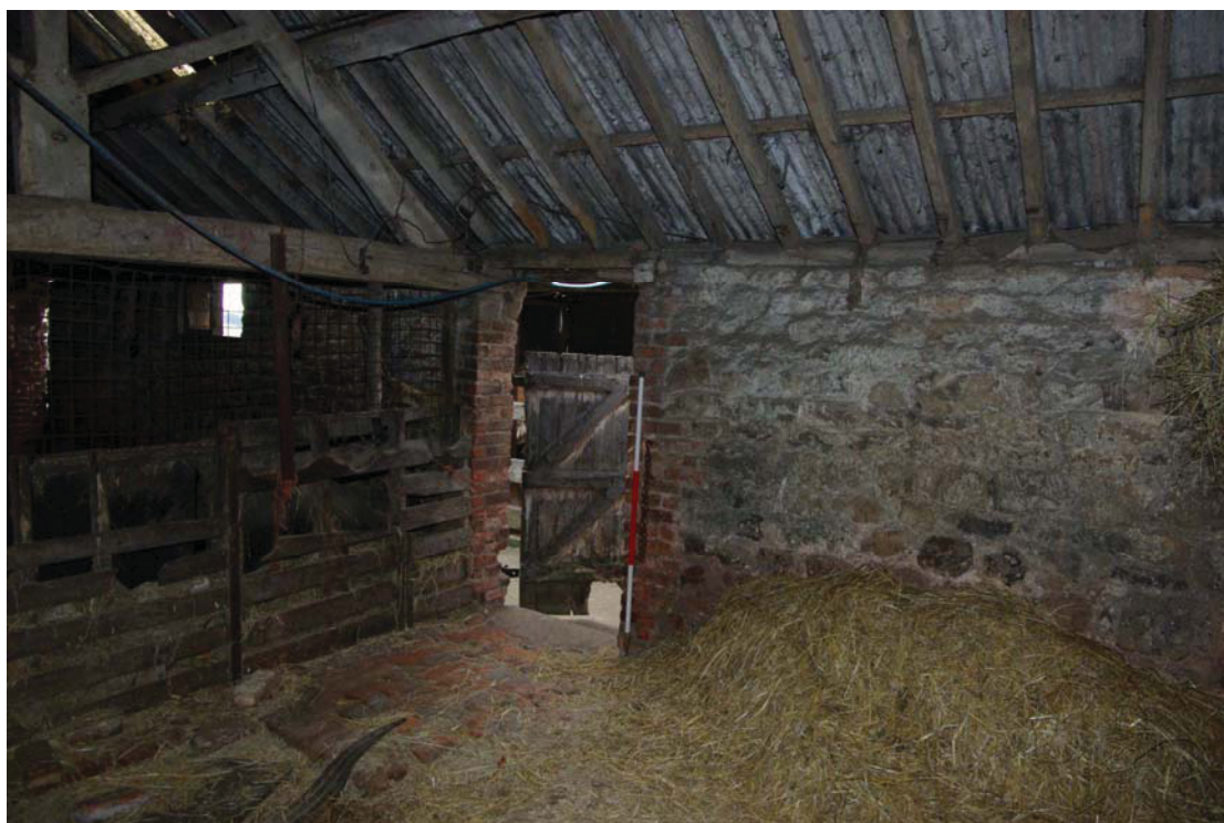
Figure 26 Barn A second bay Looking south.
