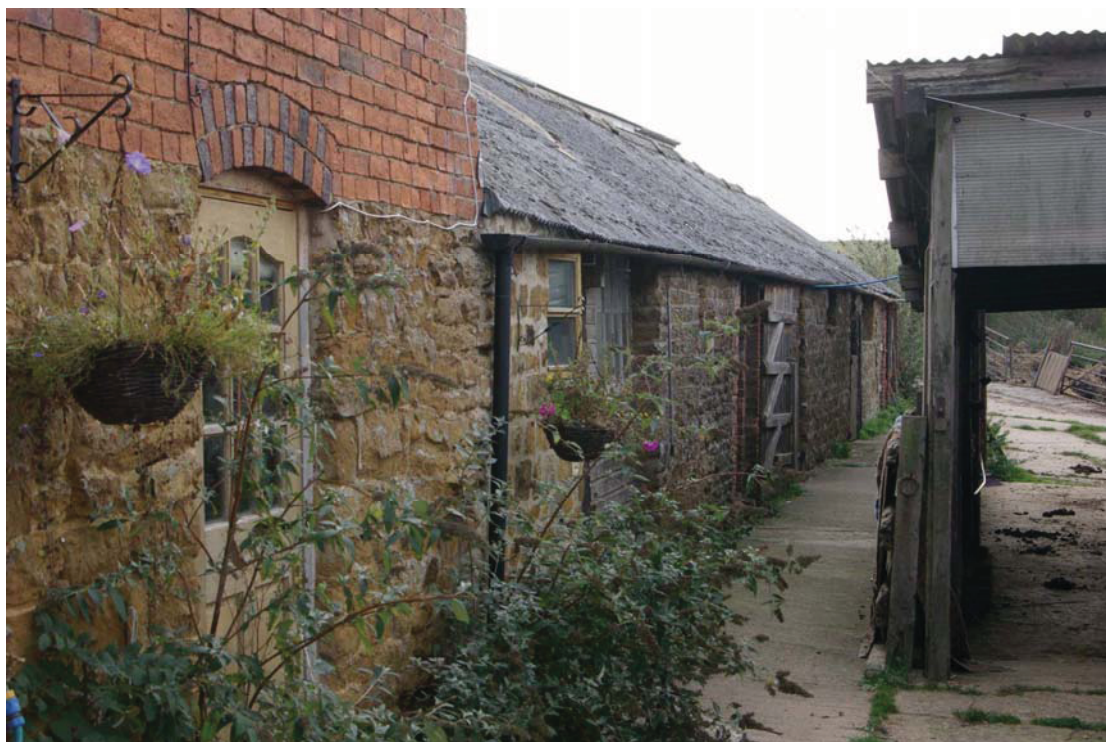
Figure 12 SW elevation of Barn A Looking east.
