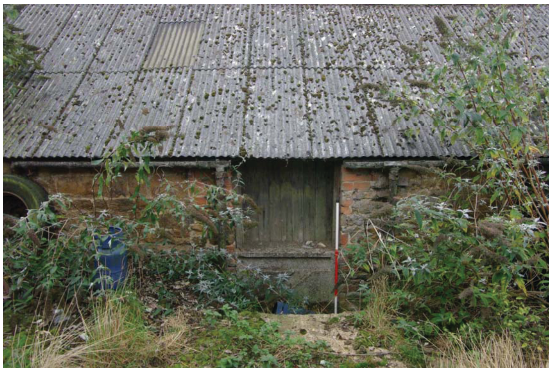
Figure 20 Barn A NE blocked doorway Looking south-west. 1.5m scale.
