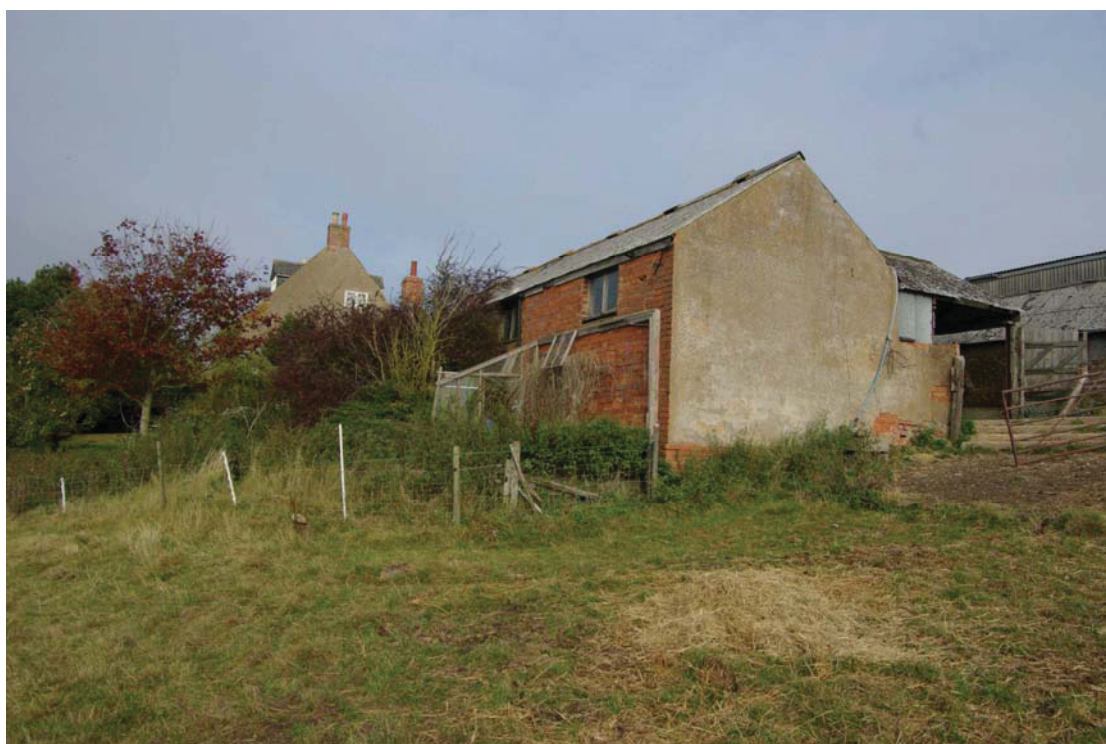
Figure 35 Barn B SE gable end Looking north-west.
