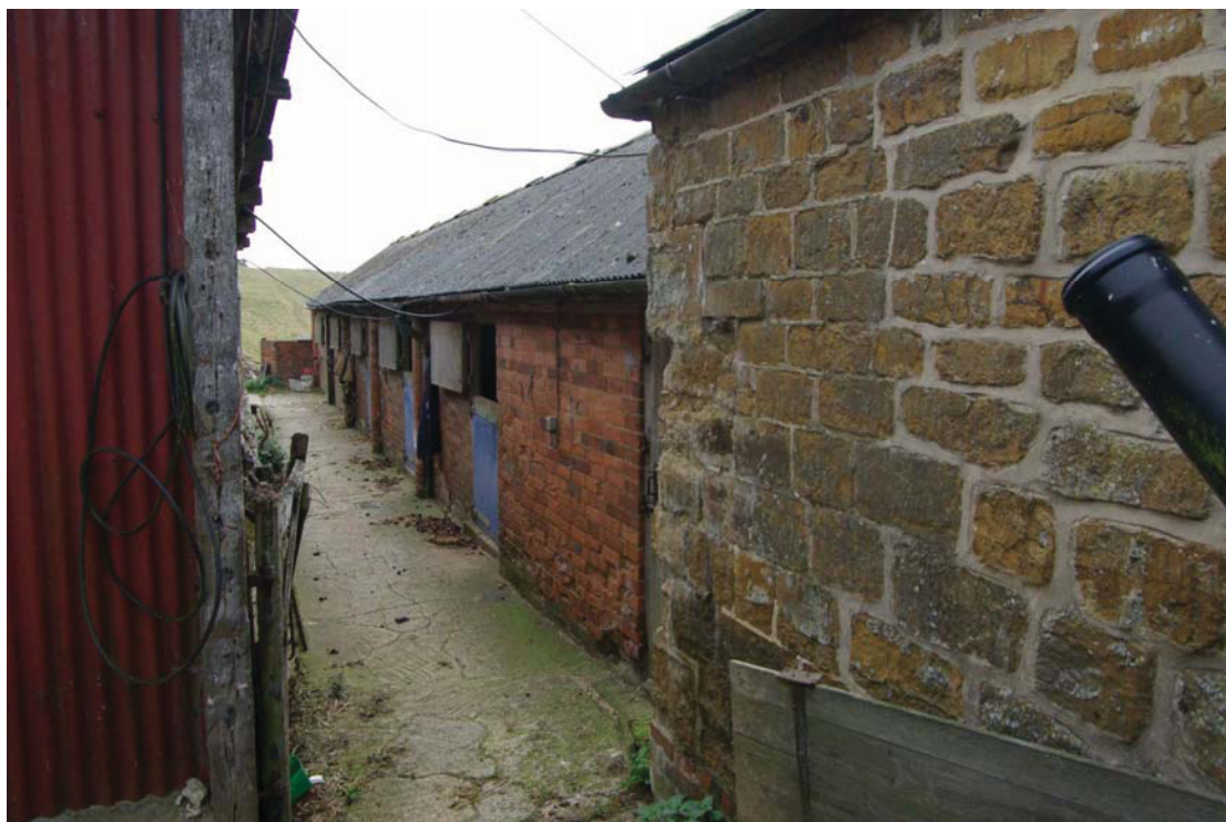
Figure 37 Barn B NE elevation Looking south-east.
