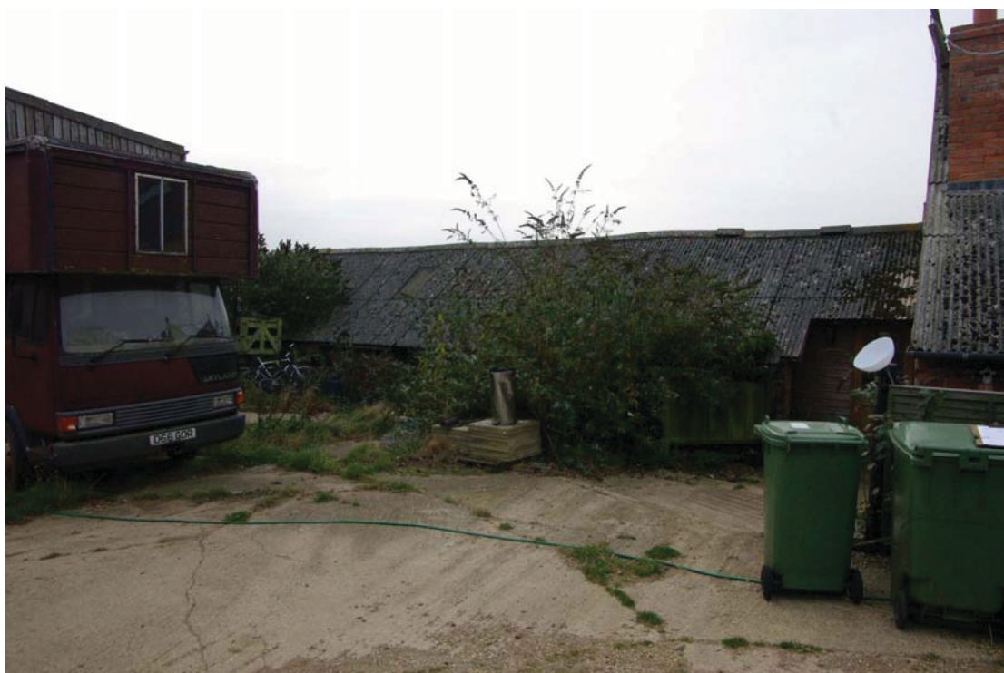
Figure 19 Barn A NE elevation Looking south.
