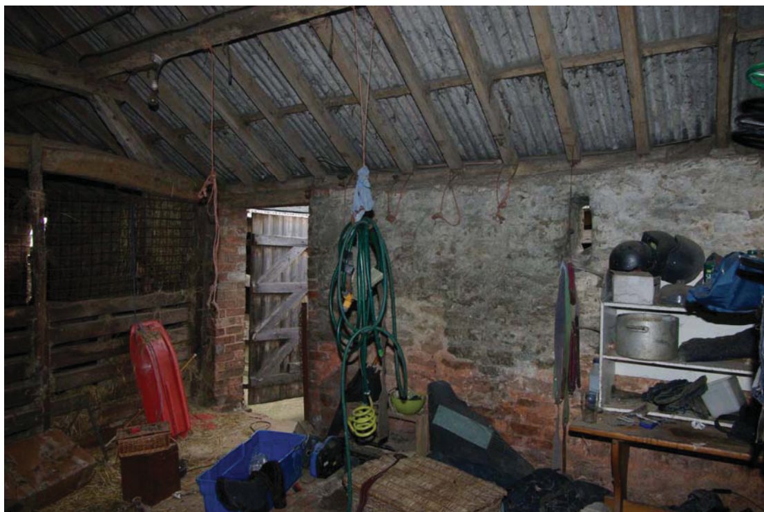
Figure 22 Barn A western end bay Looking south.
