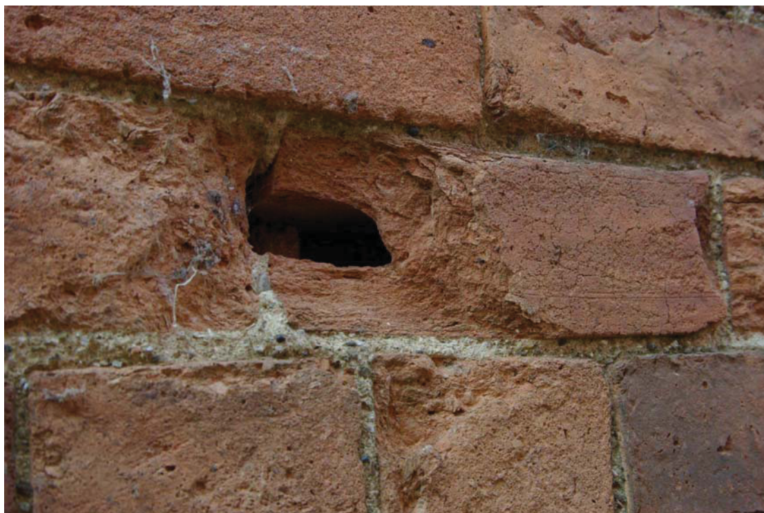
Figure 34 Barn B example of hollow brick
