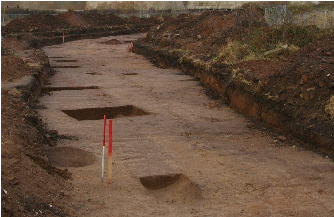
Plate 5: Post-excitation view of Haul Road, looking north
