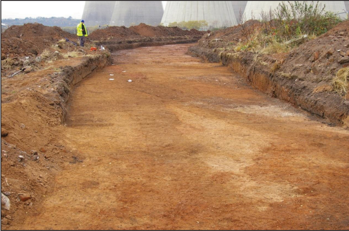
Plate 2: Haul Road trench, after stripping, looking north-east
