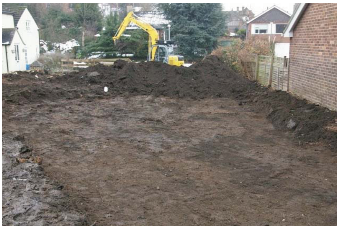
Figure 4: Ground reduction for driveway on the west side of development area
