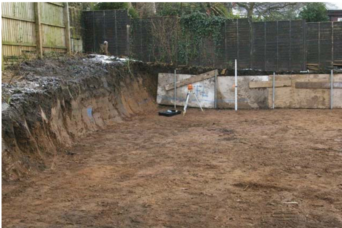
Figure 3: Ground reduction at rear of 26 Loughborough Road Shepshed
