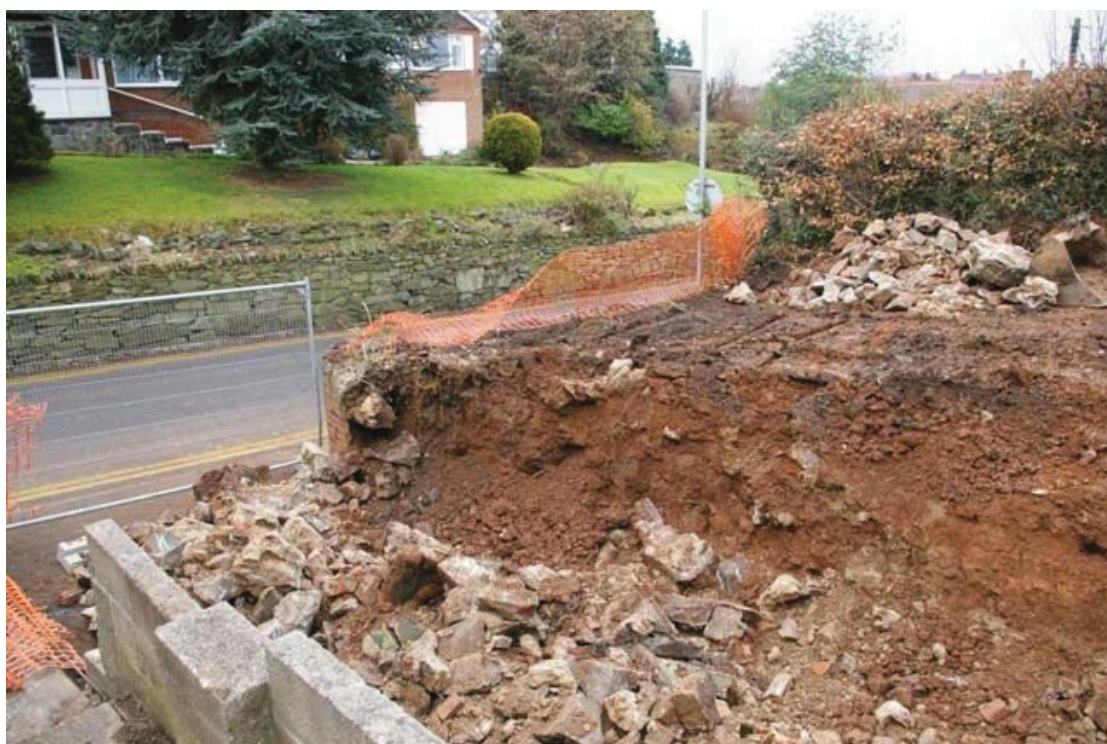
Figure 5: Demolition of car port and ground reduction at the front of 26 Loughborough Road Shepshed.
