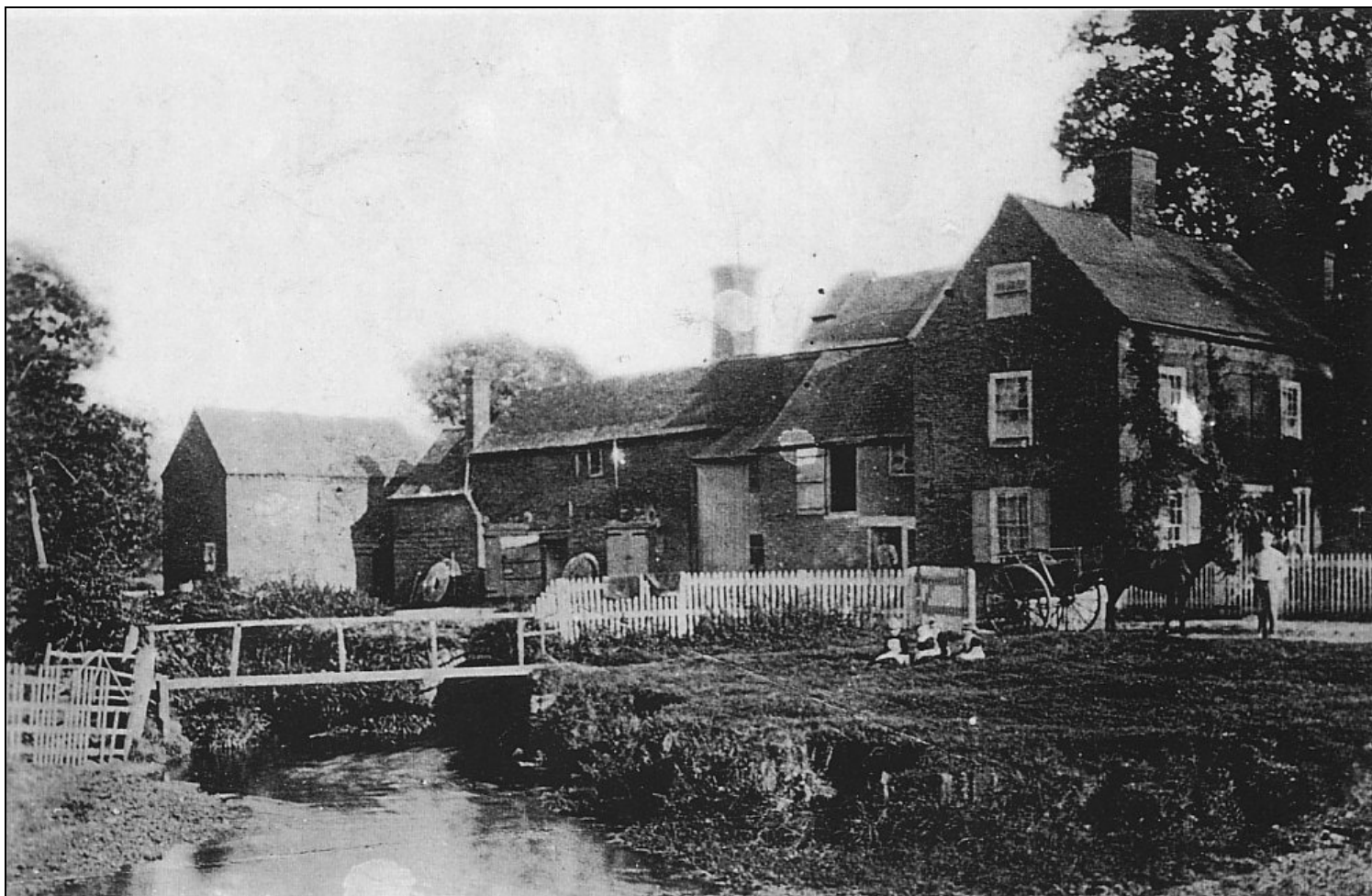
Plate 1 Photograph of the 19th century Mill buildings looking south. Note the brick culvert and the two millstones either side of the door of the middle building. Date c. 1892
