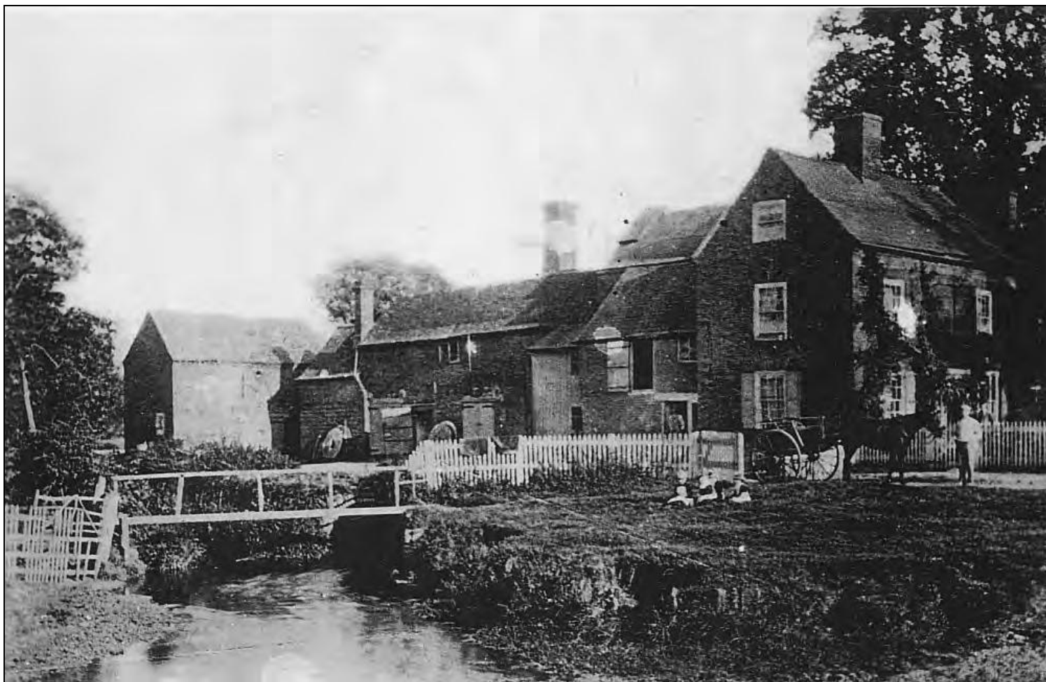
Plate 1 Photograph of the 19th century Mill buildings looking south. Note the brick culvert and the two millstones either side of the door of the middle building. Date c. 1892
