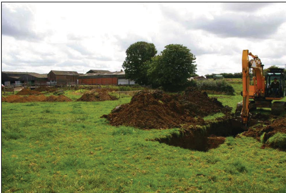
Figure 2: General view south-east across development area
