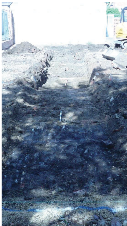
Figure 5: Trial trench looking east
