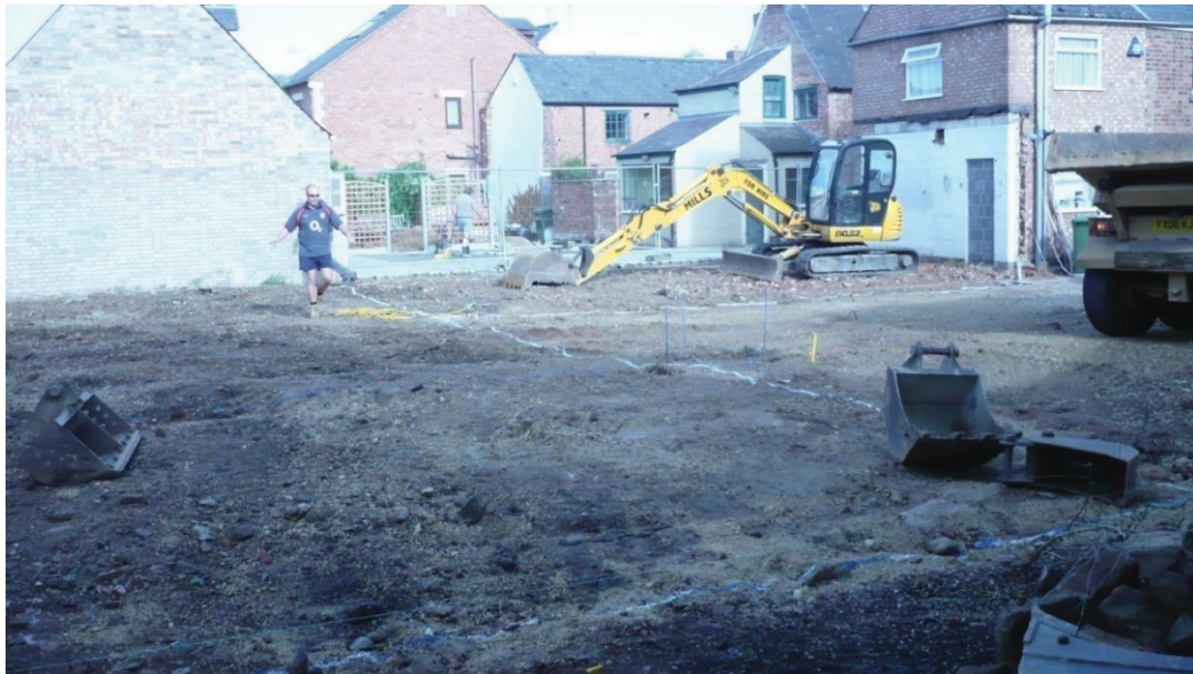
Figure 4: General site view looking north-west
