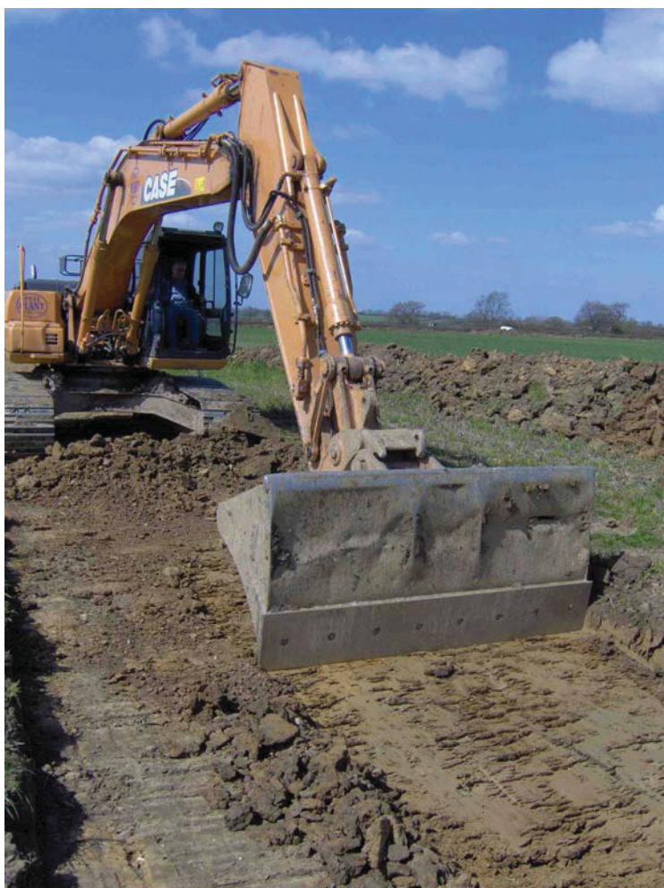
Figure 3: Machining in progress; view north-west
