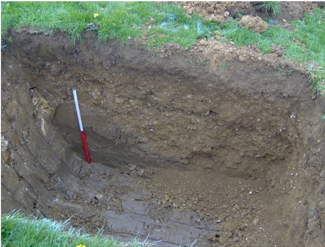
Figure 4: Winch trench – showing the natural clay dropping off to the north. Looking south-west.
