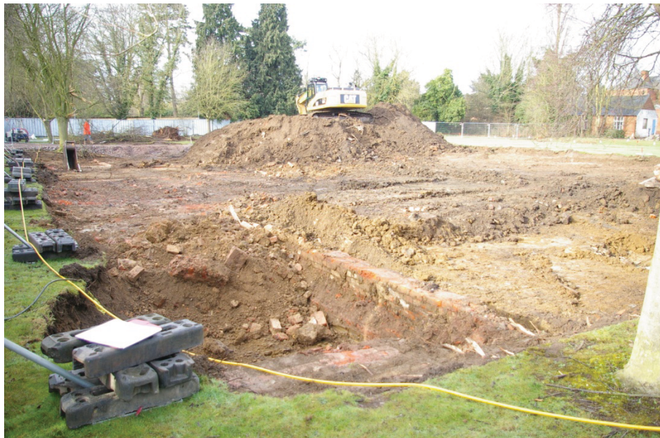
Figure 4: Site after initial strip looking west towards Leicester Road.
