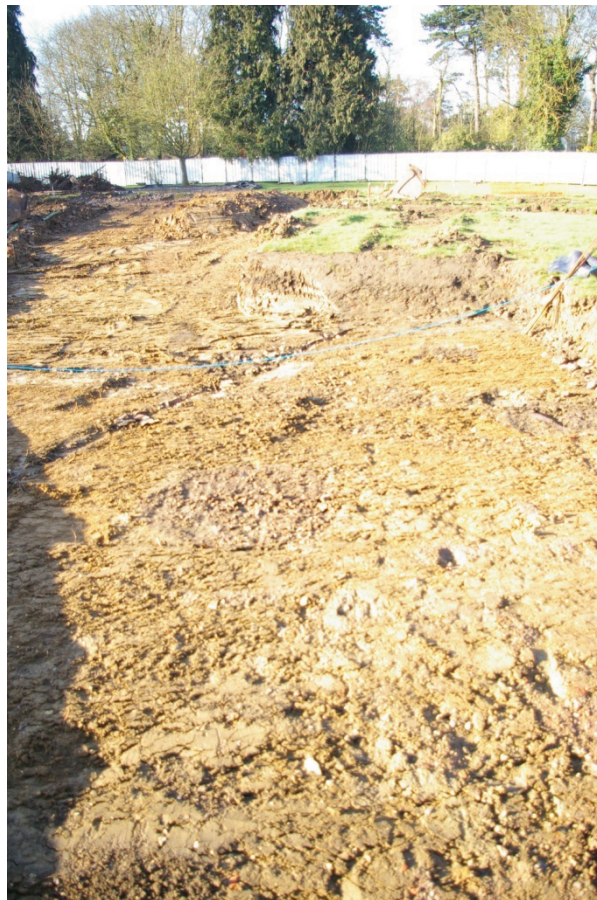
Figure 5: Looking south at the yellow clay exposed by the haul road.
