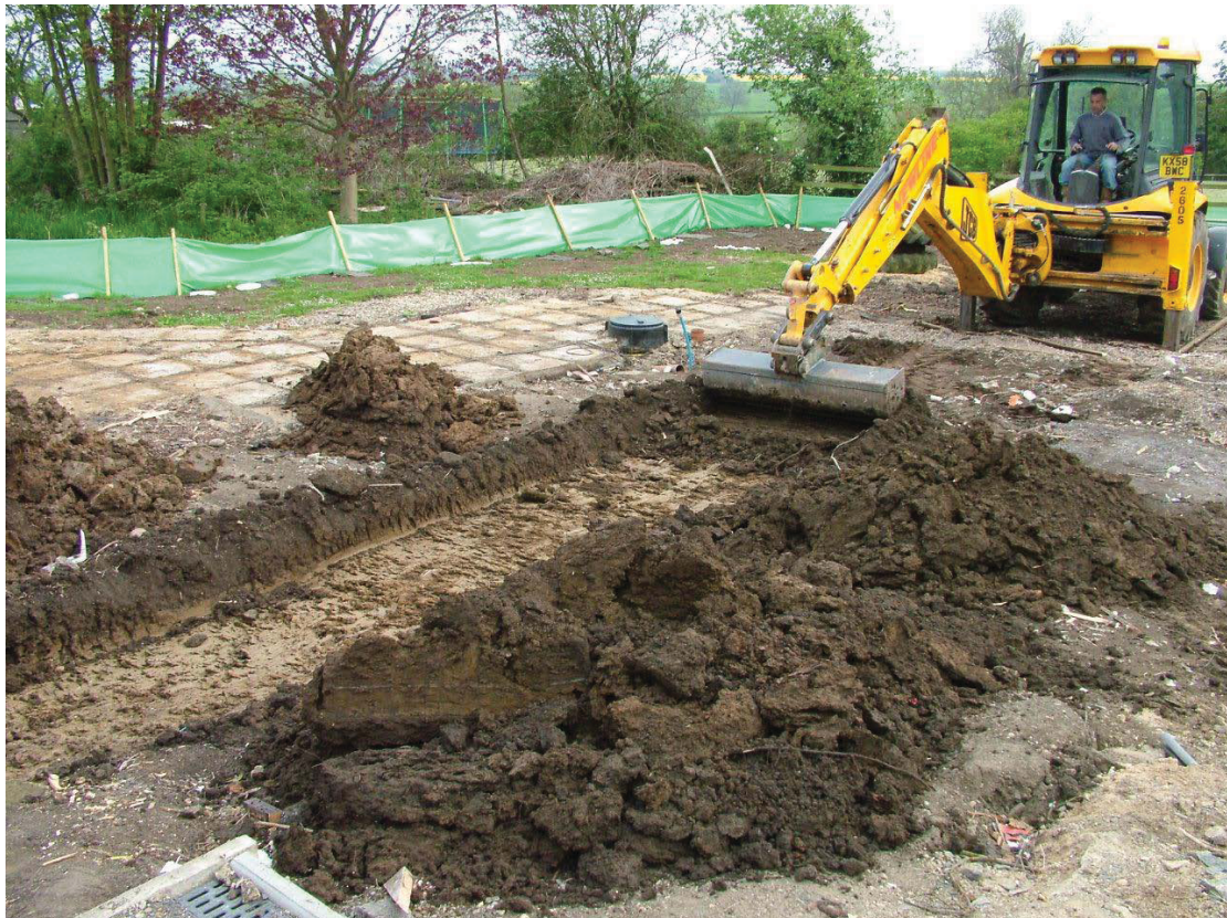
Plate 2: Work in progress on evaluation trench, looking north
