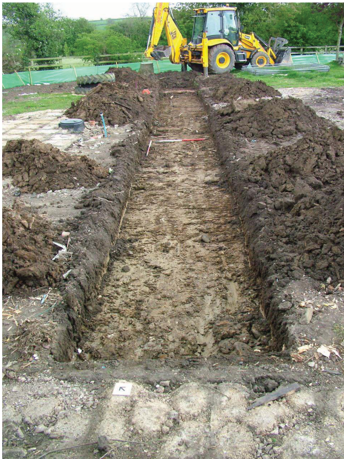
Plate 3: Post-excitation view of trench, looking north-east
