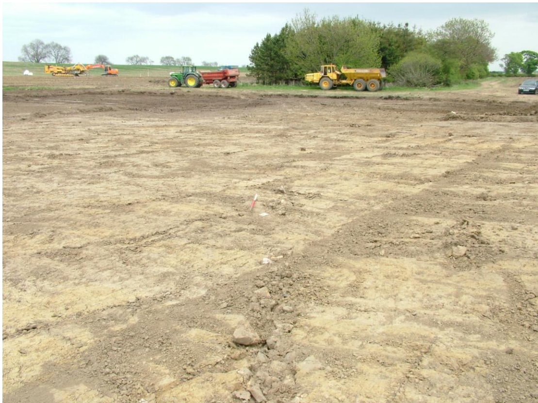
Plate 2: The site stripped to substratum, with stone filled drains running across site, looking north-east
