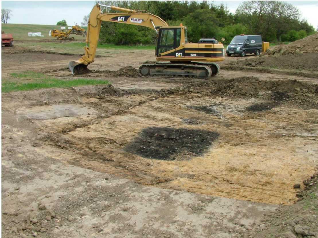
Plate 3: Work in progress revealing black silt filled pits, looking east
