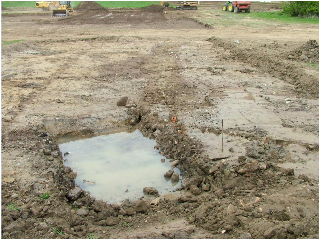
Plate 6: Spring, drains and linear feature, looking north
