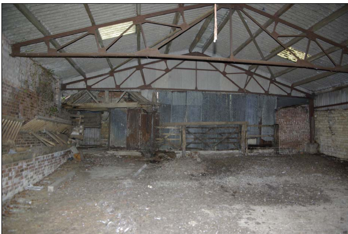
Plate 28. Infill structure interior, with brick feeding troughs and timber hayracks. Looking east.
