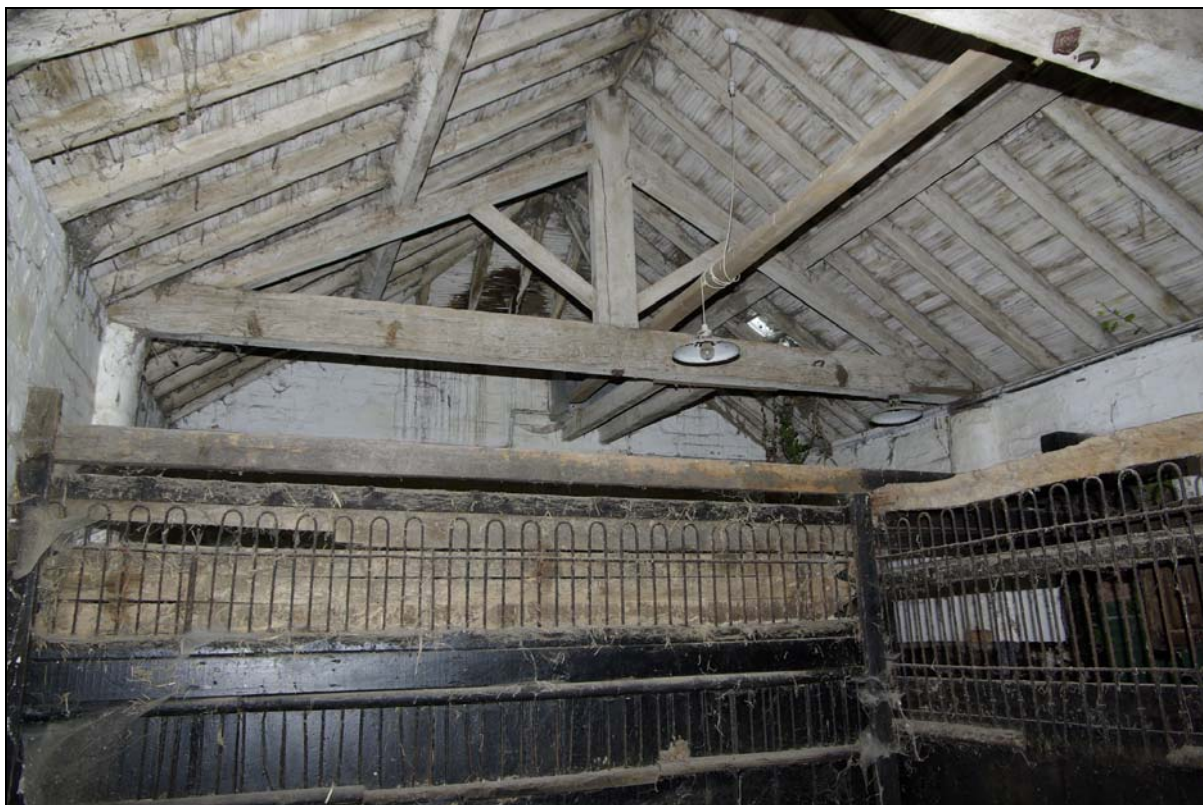
Plate 30. King post roof truss and timber partition walls forming stabling for horses at southern end of cow-shed. Looking south.
