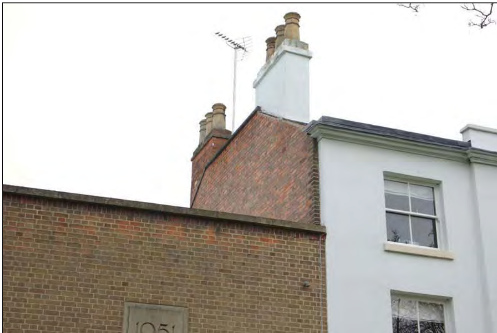
Plate 5. Brickwork skin added to gable to 58-60 New Walk. Looking east.
