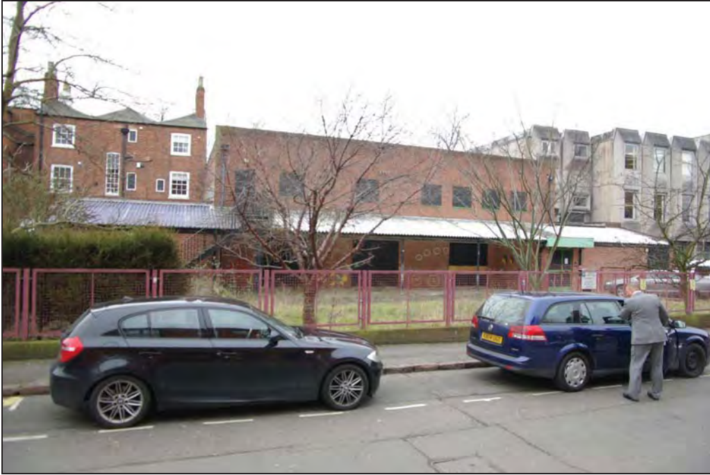
Plate 2. 50-56 New Walk/69 Wellington Street: Wellington Street Elevation, looking south-west.
