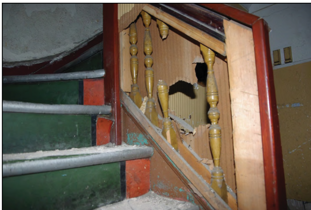
Plate 19. Staircase detail. Looking west.
