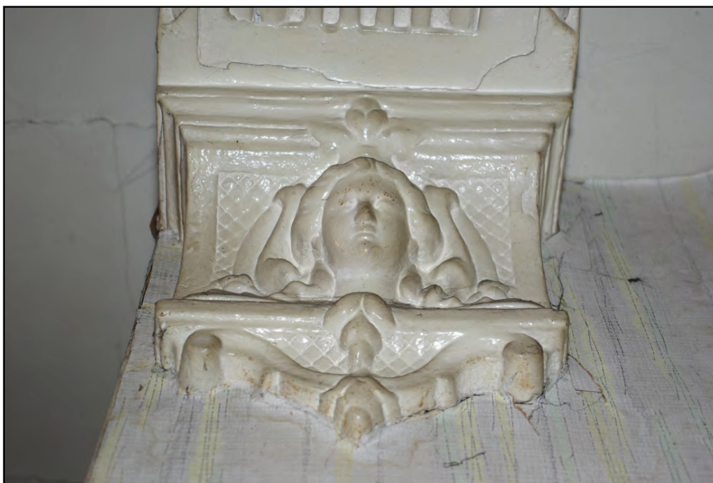
Plate 10. Plasterwork detail. Looking south.
