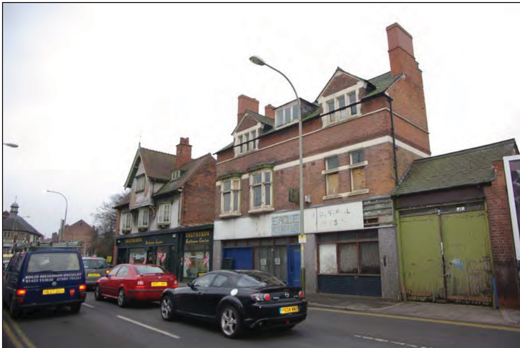
Plate 1. Numbers 4 and 10 Northgate Street, Leicester. Looking south
