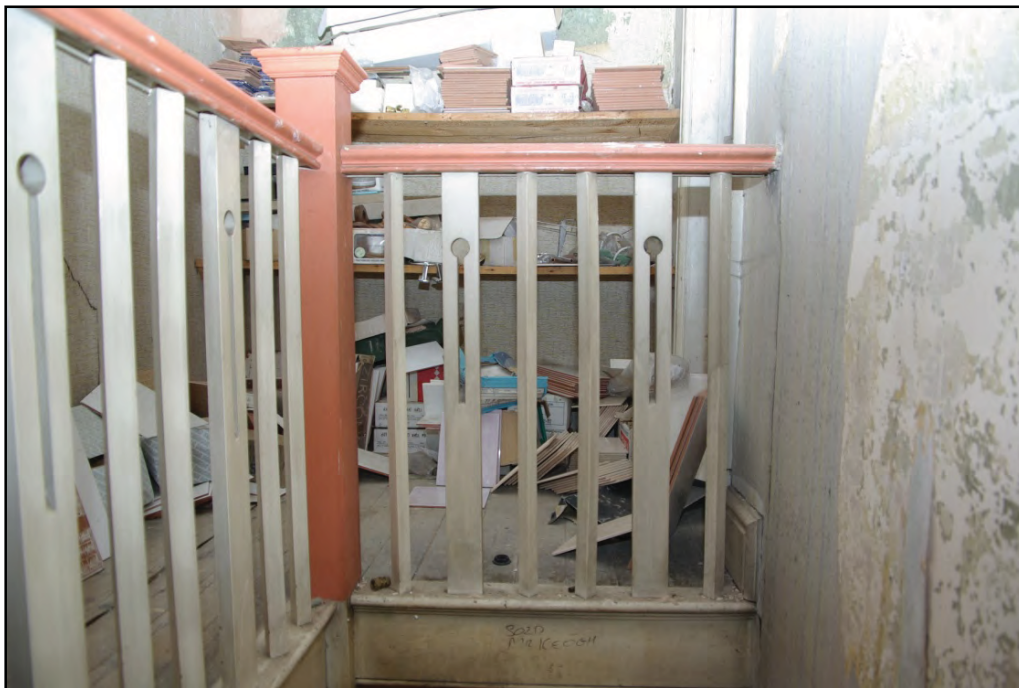
Plate 12. Attic floor staircase. Looking north.
