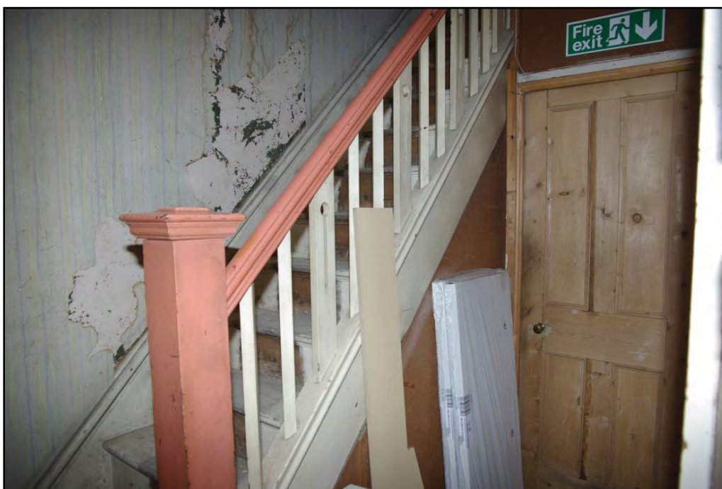
Plate 11. First floor staircase. Looking east.
