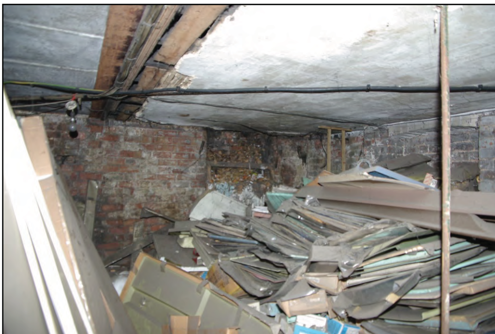
Plate 7. Basement, with chimney stack. Looking southeast.
