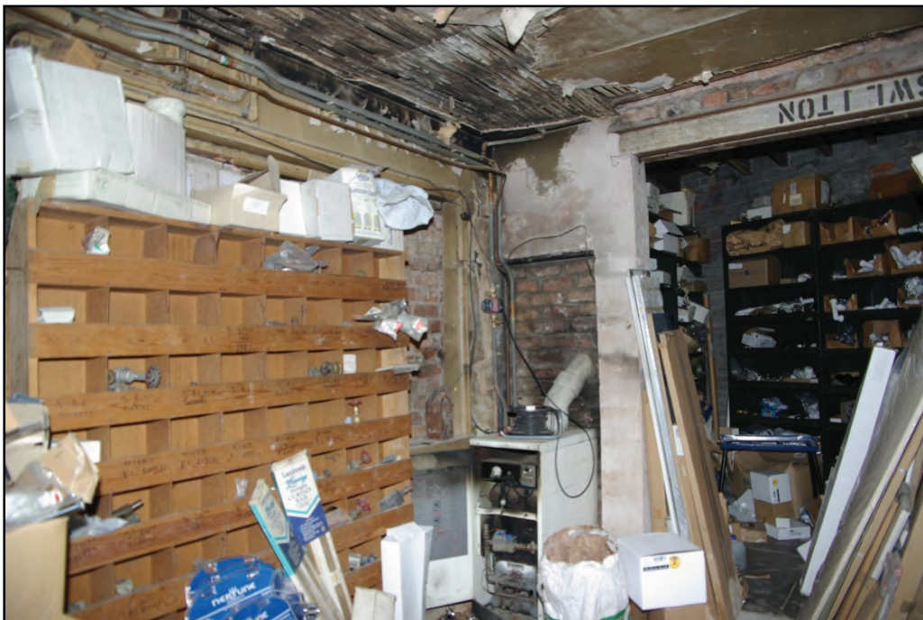
Plate 5. Former kitchen with blocked window opening. Looking southwest.
