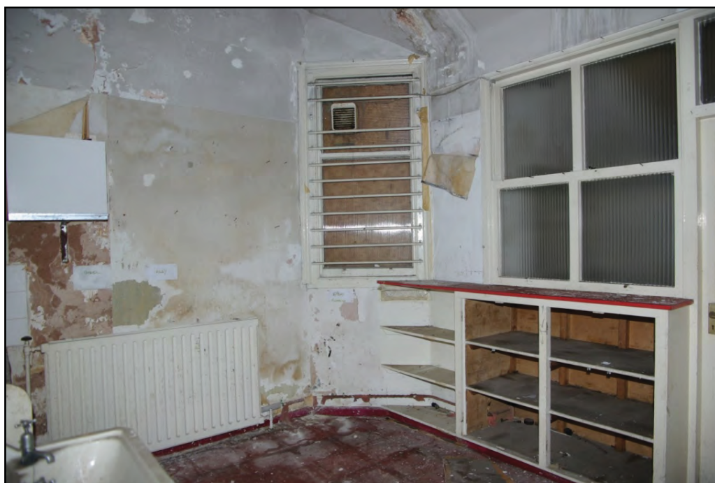
Plate 18. Rear kitchen, within lean-to extension. Looking west.
