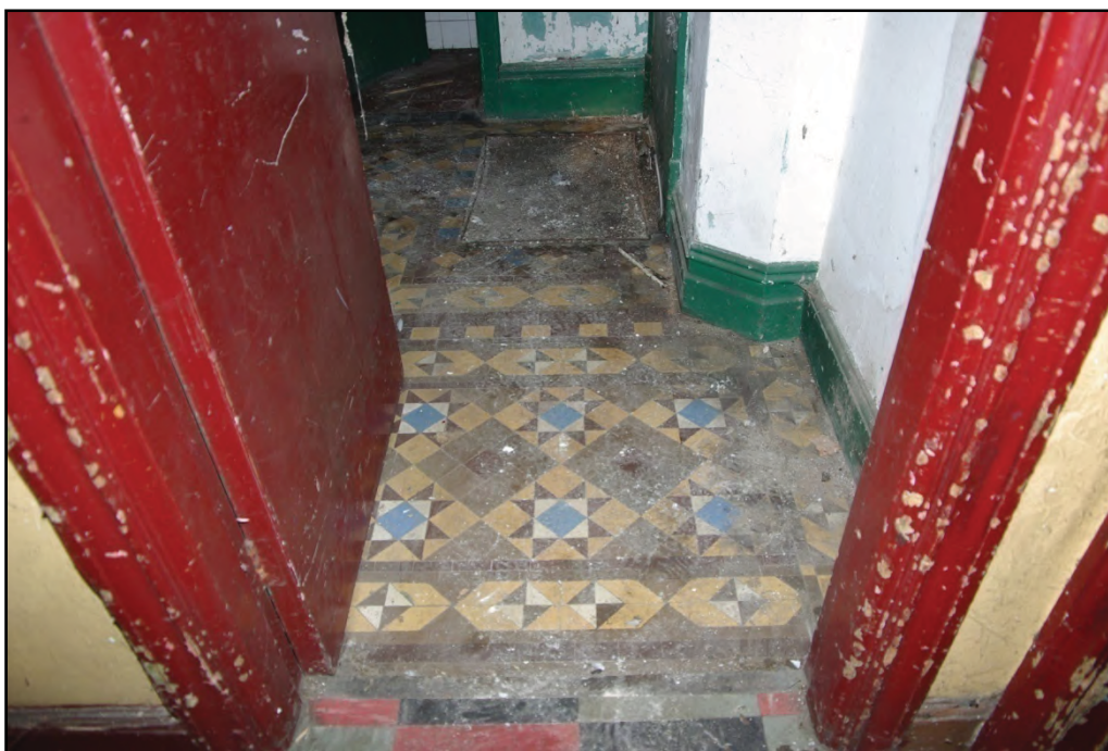
Plate 20. Tiled floor within former rear lobby. Looking west.
