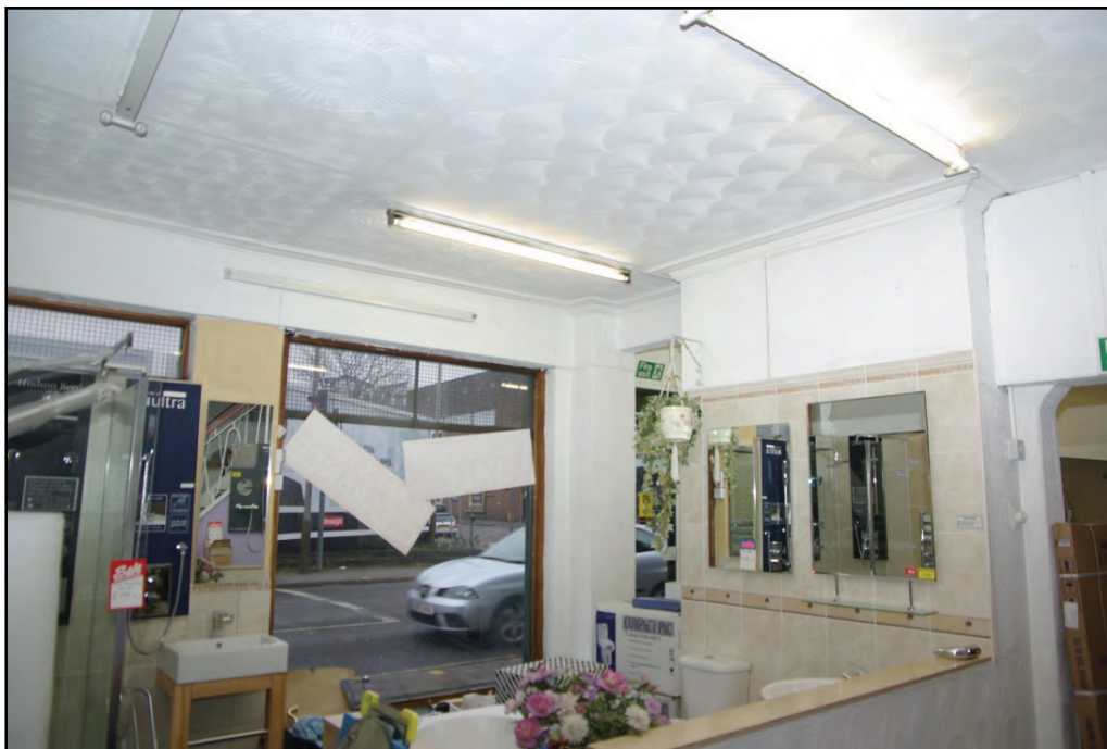
Plate 3. Former sitting room, looking southeast.
