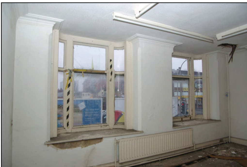
Plate 21. Oriel windows lighting first floor clubroom. Looking east.
