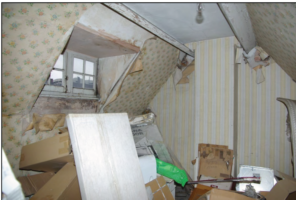
Plate 13. Former attic bedroom. Looking southeast.
