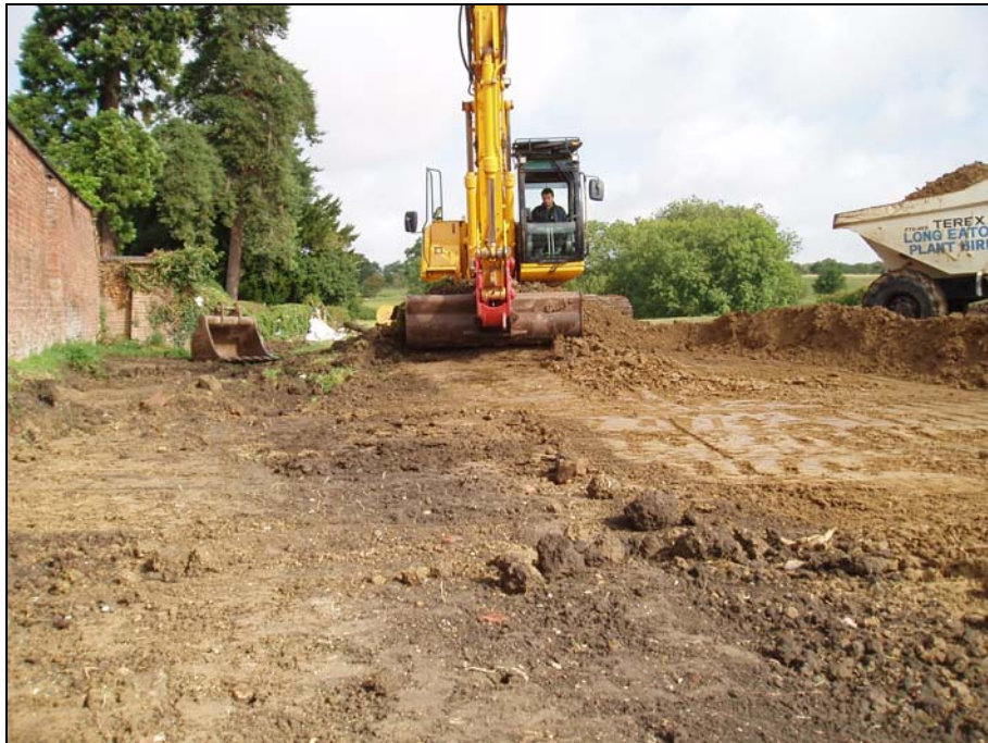
Plate 26. Topsoil stripping over footprint of stable block. Looking north.
