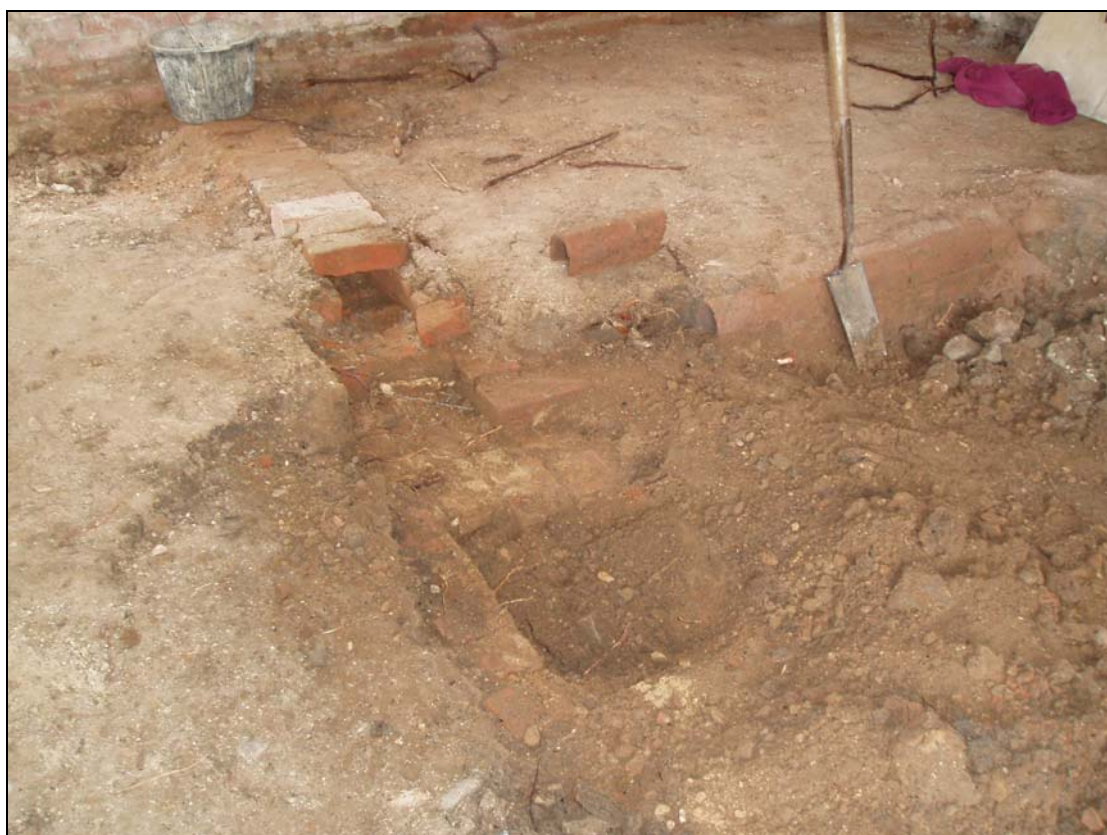
Plate 18. Under-floor drainage system located within former workshop. Looking north.
