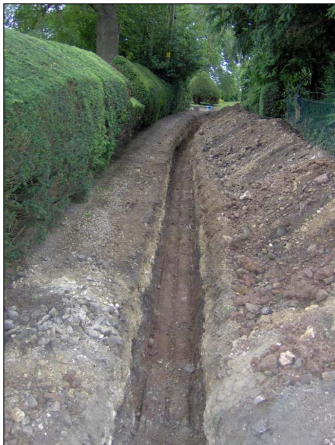
Plate 31. Service trench along driveway. Looking east from Main Street.
