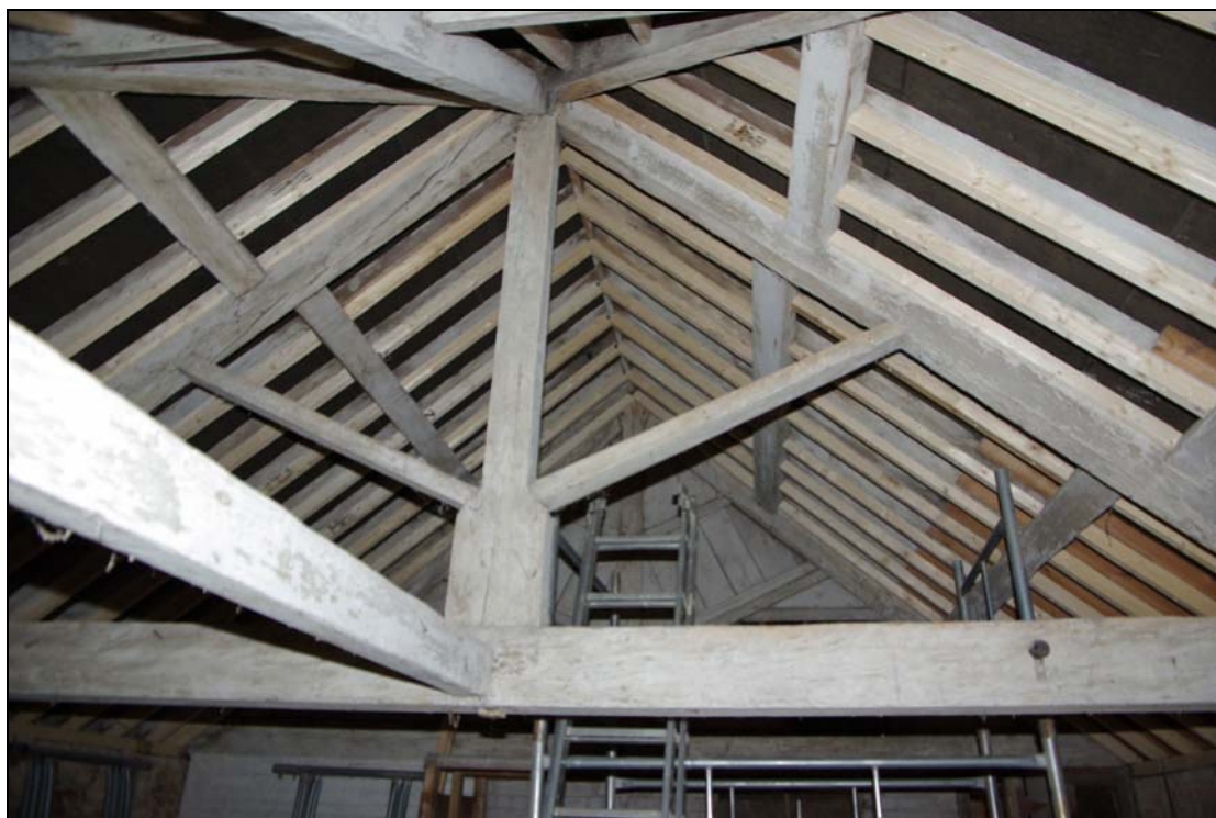
Plate 13. King post roof truss, looking west.
