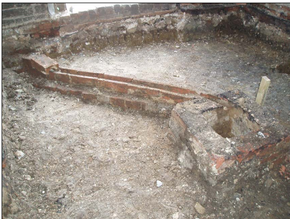
Plate 20. Drainage system located beneath stable floor. Looking west
