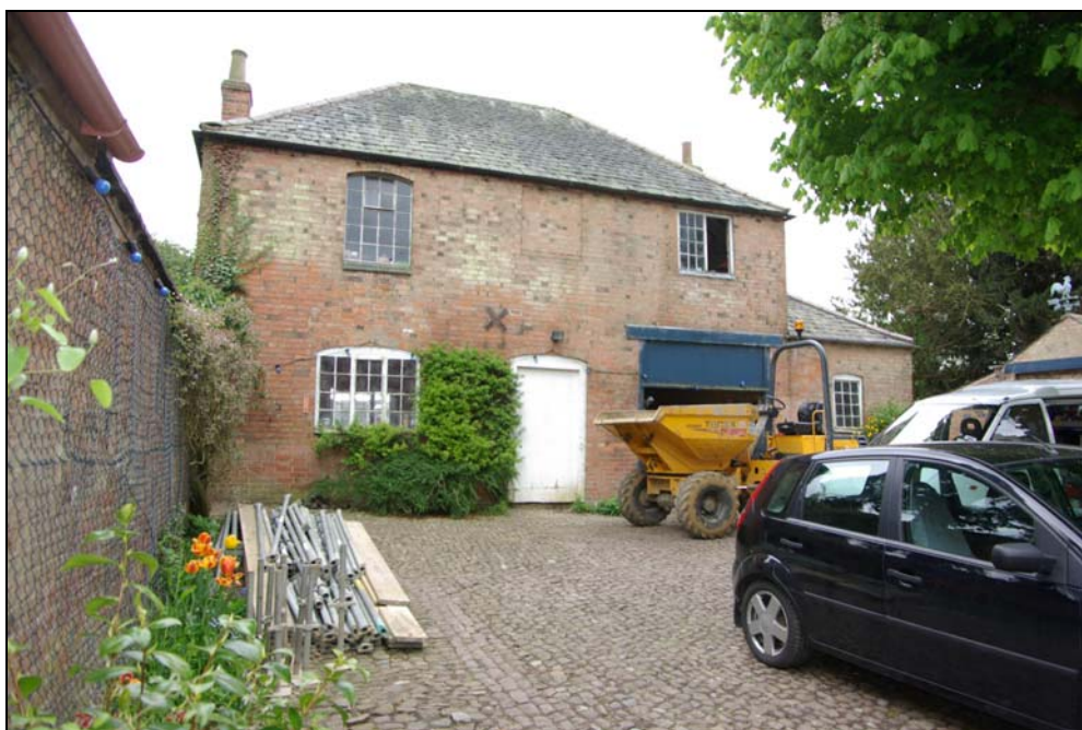
Plate 2. Principal elevation, looking south.
