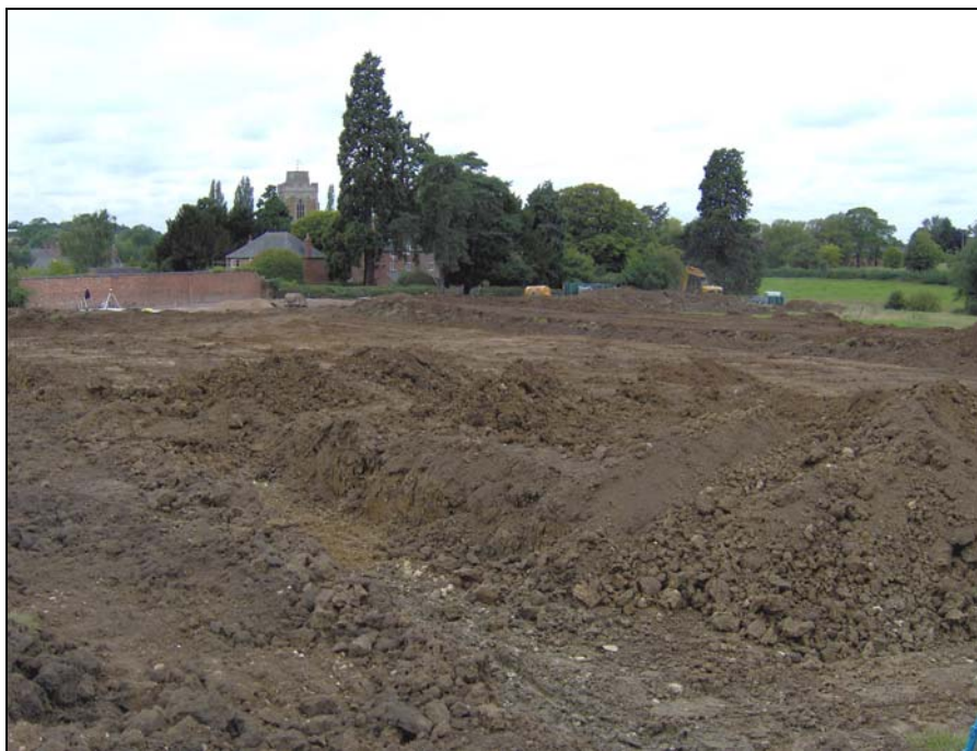
Plate 29. Topsoil stripping in manège area. Looking west.
