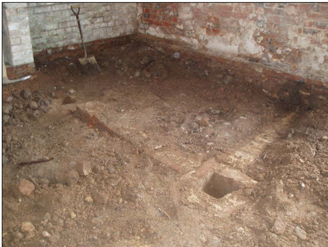
Plate 17. Under-floor drainage system located within former workshop. Looking east.
