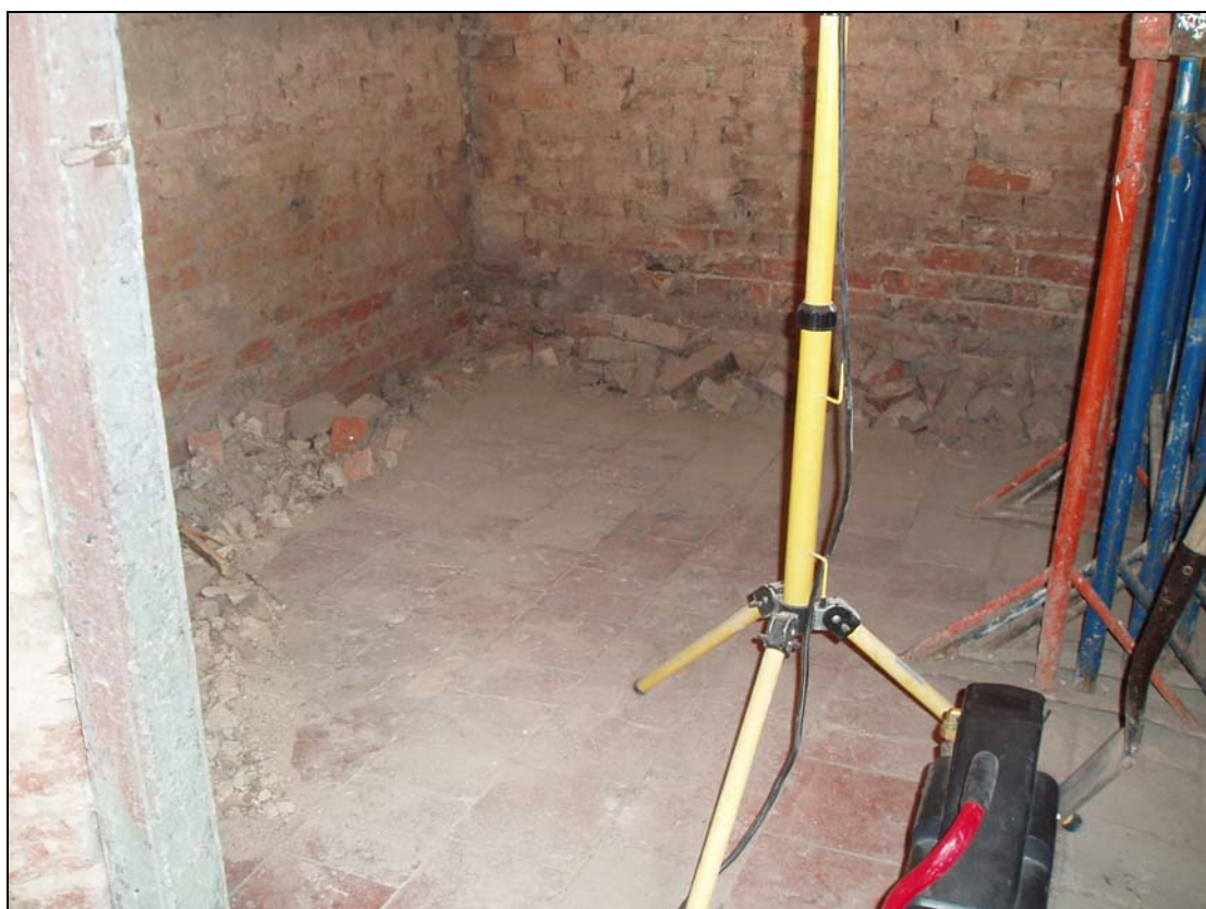
Plate 22. Quarry tiled floor of sitting room. Looking south.
