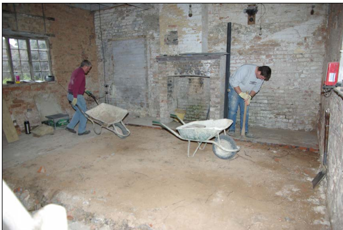
Plate 4. Ground floor workshop, looking east.
