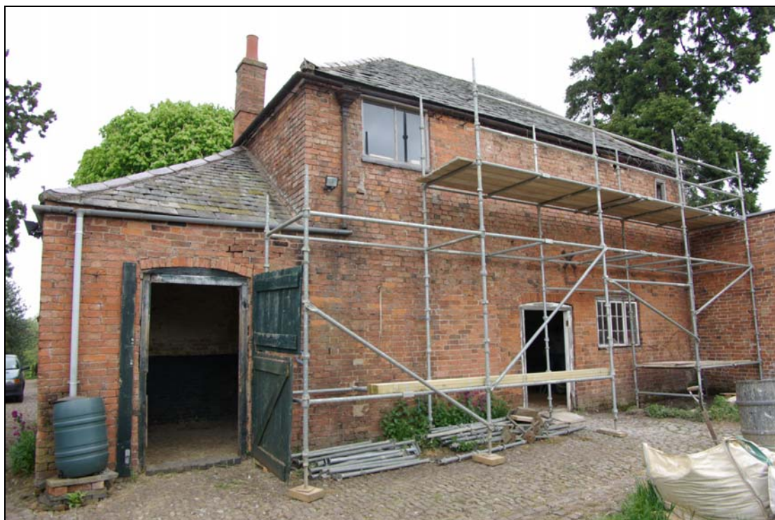
Plate 3. Rear elevation, looking north-east.
