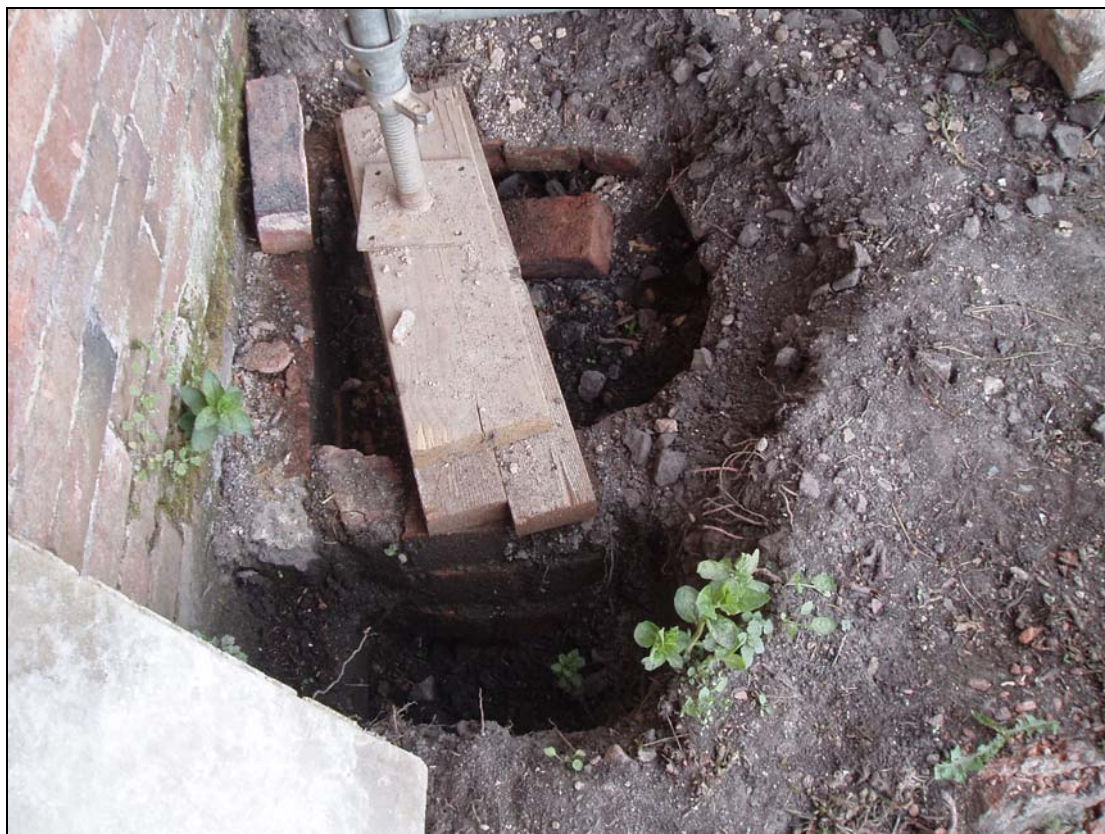
Plate 19. Brick-lined sump located externally, to rear of building. Looking north-east.
