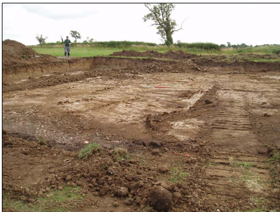
Plate 27. Reduced ground level in stable block area. Looking south.
