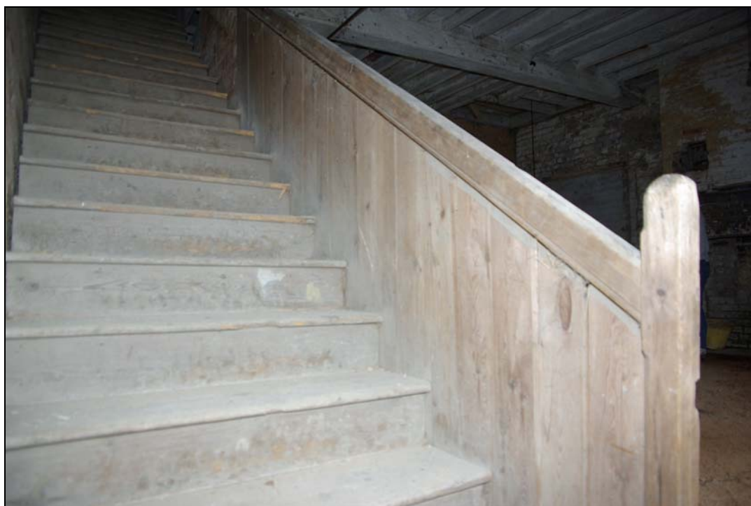
Plate 9. Handrail and newel post staircase detail.
