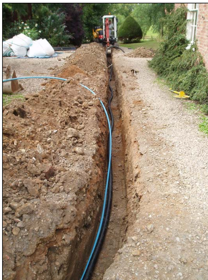
Plate 30. Service trench along driveway. Looking north.
