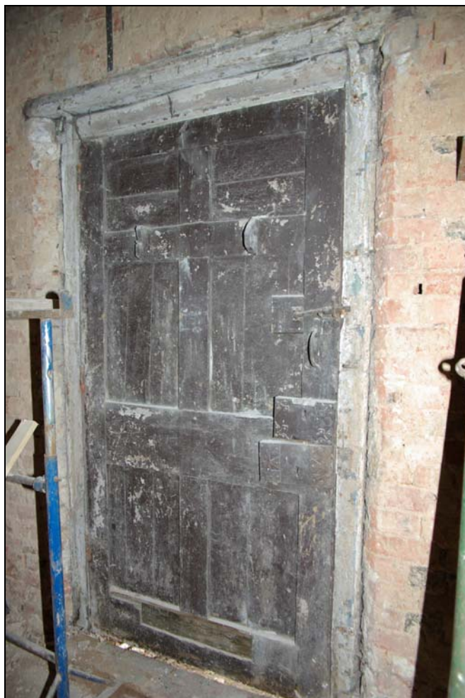
Plate 5. Early timber door to principal entrance, looking north.
