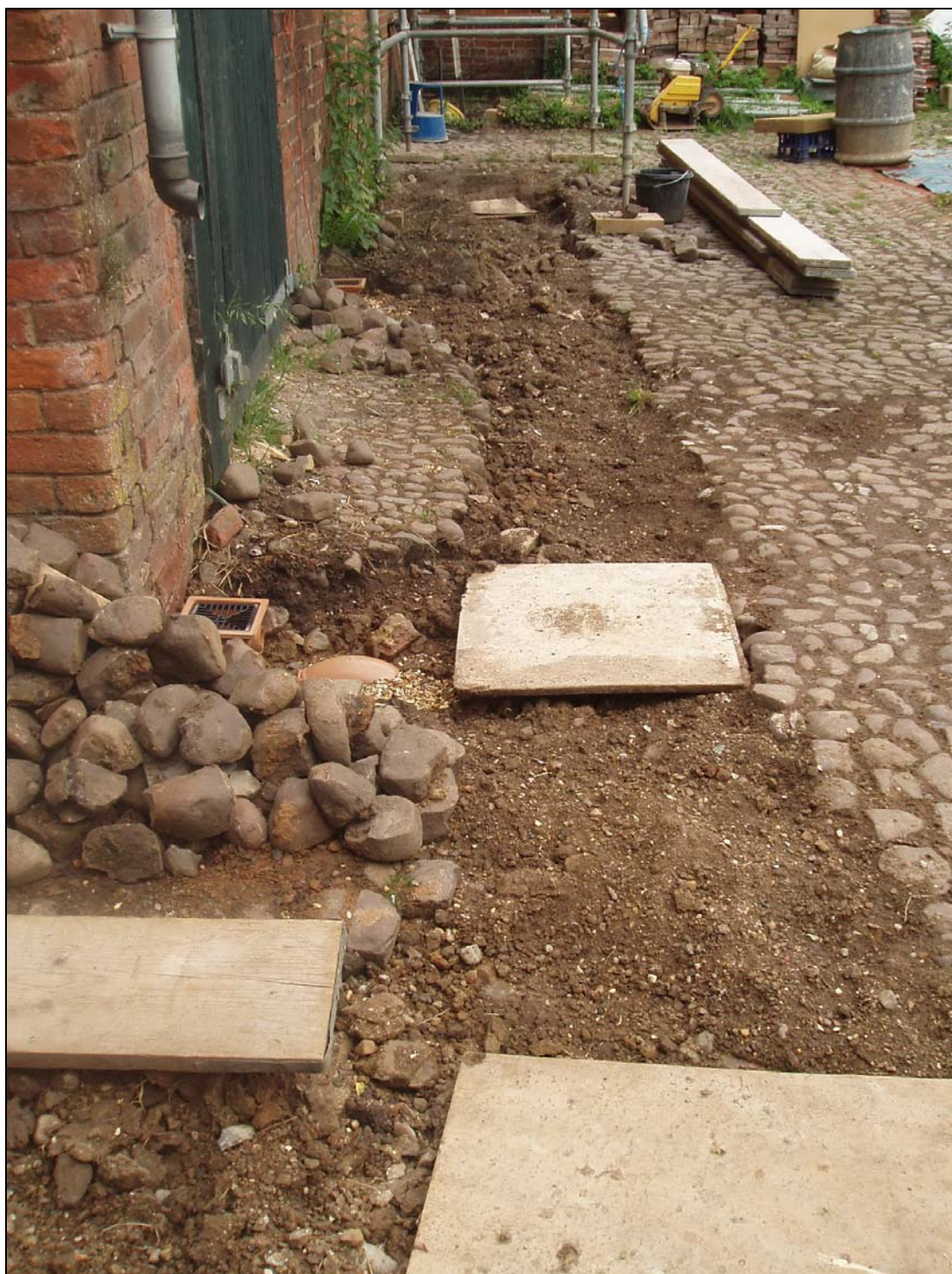
Plate 25. Back-filled service trenches. Looking north-east.
