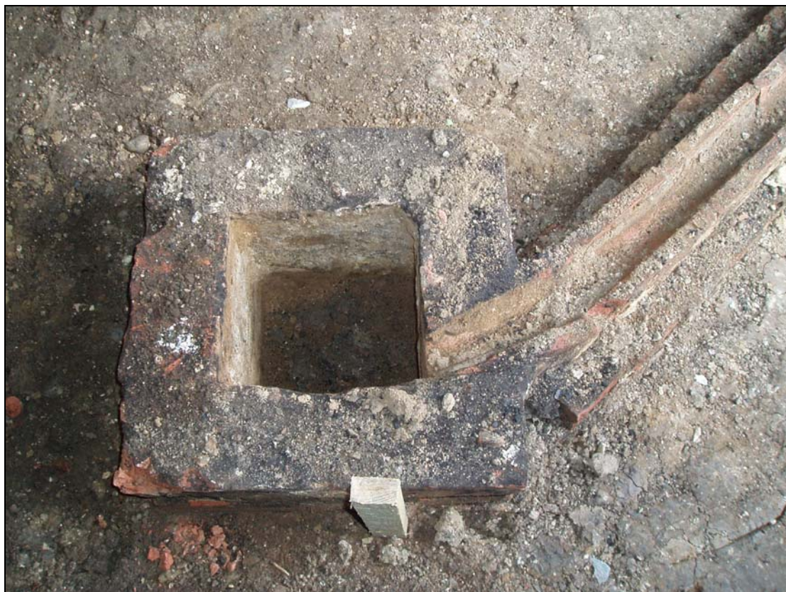
Plate 21. Concrete-lined drain beneath stable floor. Looking north-east.
