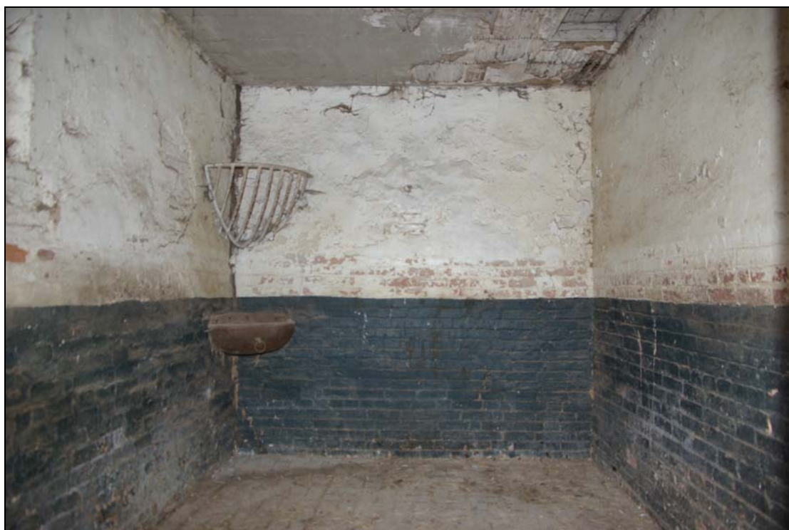
Plate 12. Rear loose-box, with cast-iron bowl trough and over-head hay rack. Looking north.
