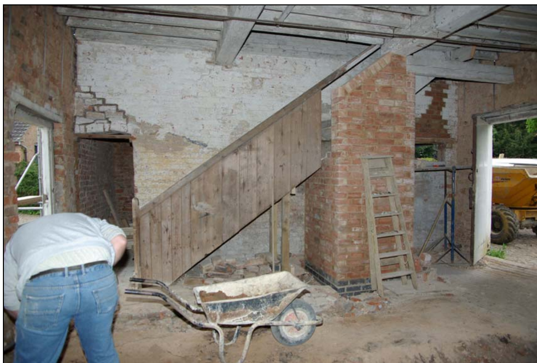
Plate 8. Timber staircase, with newly constructed brick pier. Looking west.
