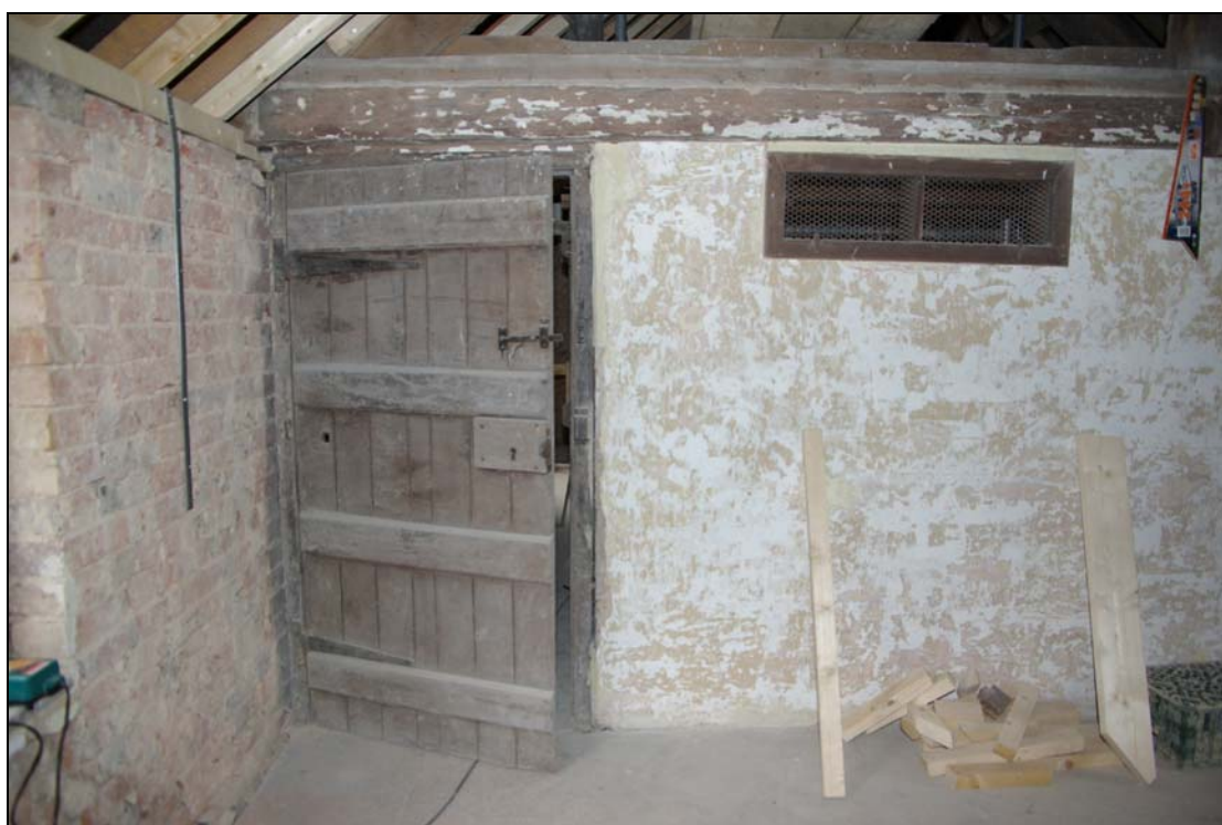
Plate 16. Early plank and batten door, with ventilation panel in wall, looking west.
