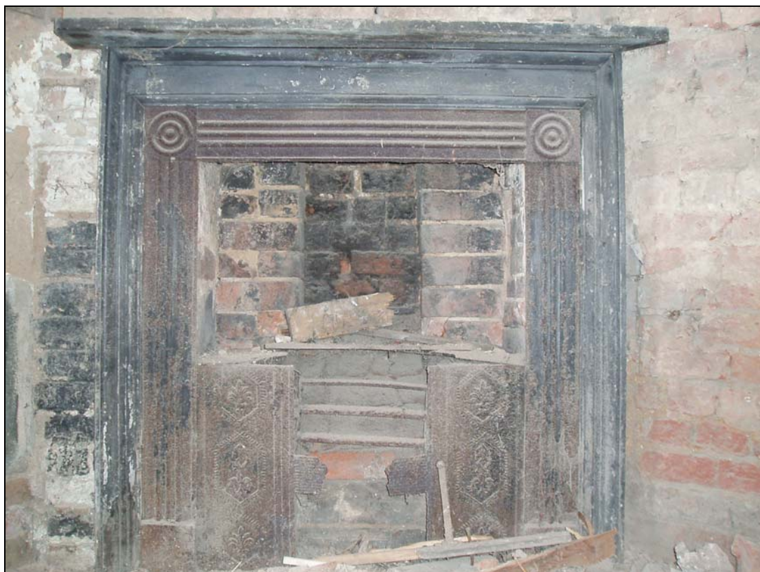
Plate 11. Cast-iron, pantheon pattern hob-grate, in ground floor sitting room. Looking south-east.
