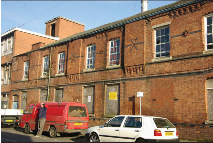
Figure 21. Block G. Decorative treatment to external chimney stacks. Looking northeast.
