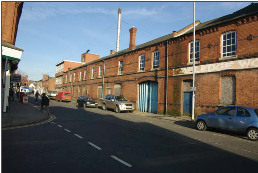
Figure 16. Block G Canal Street frontage, Orson Wright's 'Perseverance Works'. Looking north.
