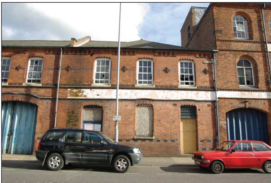
Figure 22. External junction between Blocks G, J and K. Looking east.
