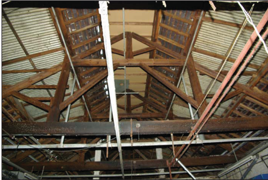
Figure 20. Block F Roof Structure, looking northwest.
