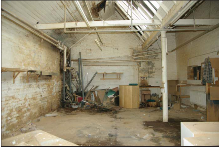
Figure 40. Northlight range to rear of No. 30 Canal Street, looking south.
