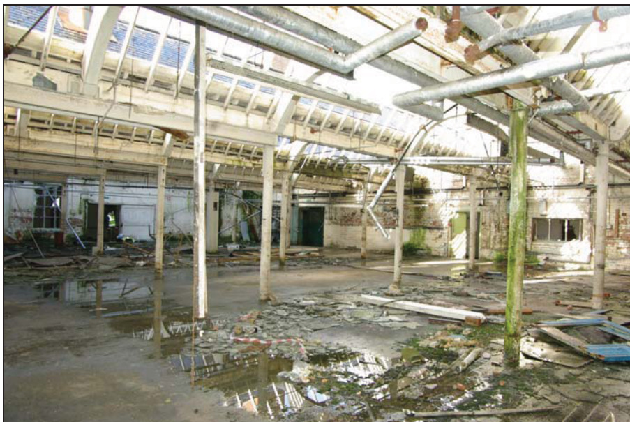
Figure 28. Block L, northlight factory to rear of Block K. Looking northwest
