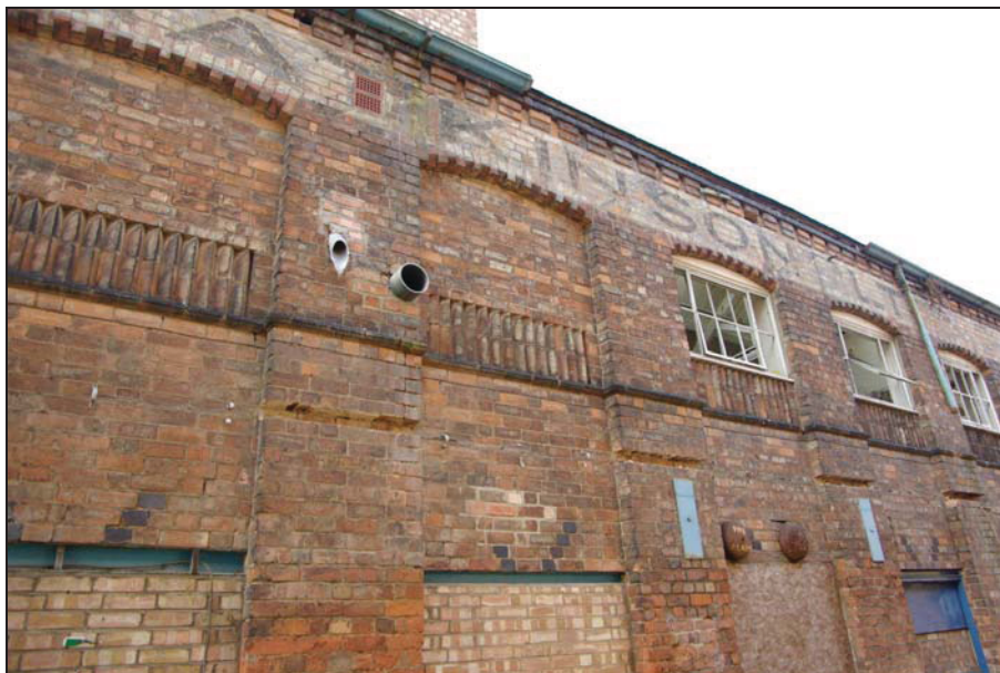
Figure 23. East facing façade of Block I, showing remnants of decorative brickwork.
