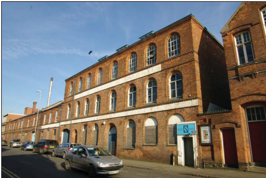
Figure 25. Block K (Benjamin Toone's Factory), Canal Street Elevation. Looking northeast.
