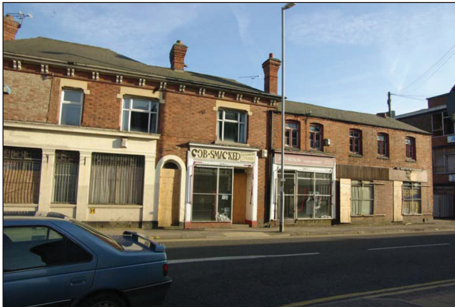
Figure 15. 4, 4a-8 Canal Street, looking east.
