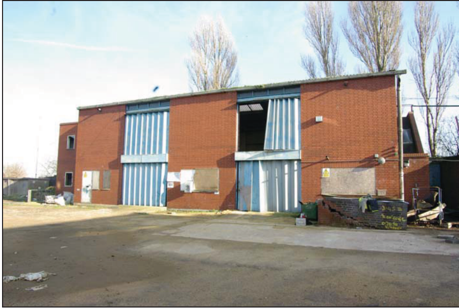
Figure 17. Block B, looking east.
