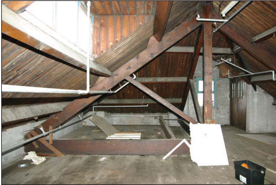
Figure 27. Block K, modified hipped roof structure. Looking north.
