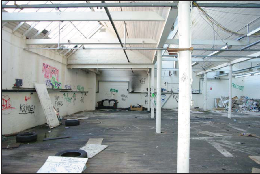
Figure 38. Block N Northlight factory, looking north
