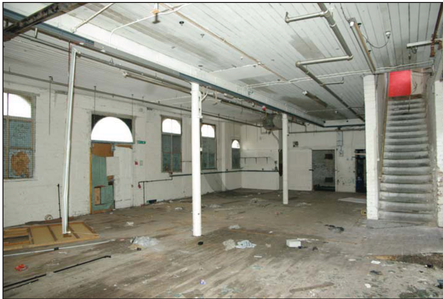
Figure 26. Block K, Ground Floor. Looking north.
