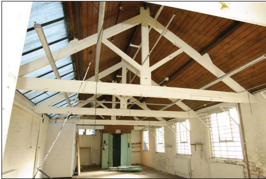
Figure 39 .King-post roof trusses to rear workshop at 28 Canal St, looking east.
